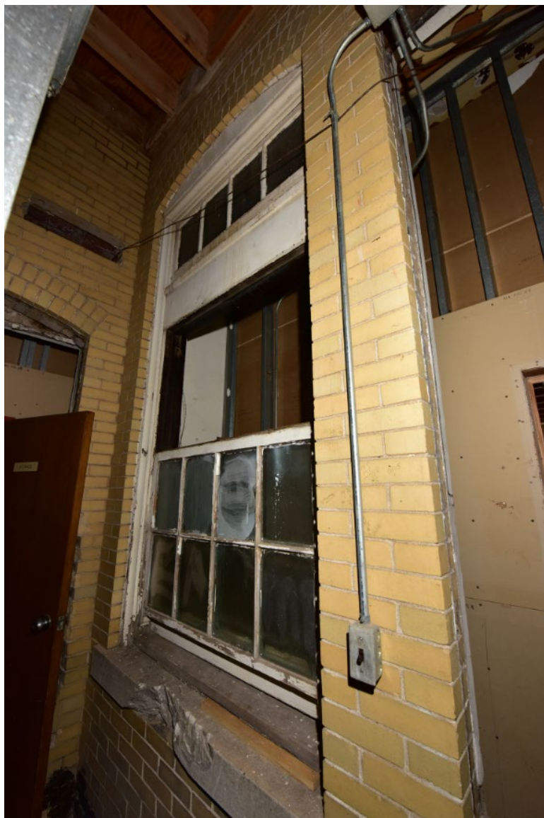
Figure 14. Lightwell to south of the former Boys' Lobby/current Meeting Room on first floor, looking NW. Source: Brad Finch, January 2021.
