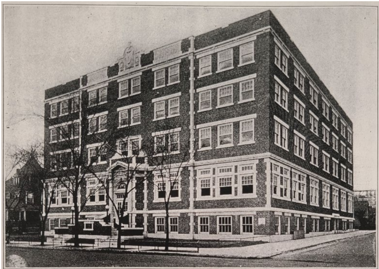
Figure 6. The Joplin YMCA in 1921, shortly after opening. View is looking southwest at the east and north elevations. Note the lawn and house to the south of the building. Source: "Organizations—YMCA" Vertical File, Joplin Public Library.
