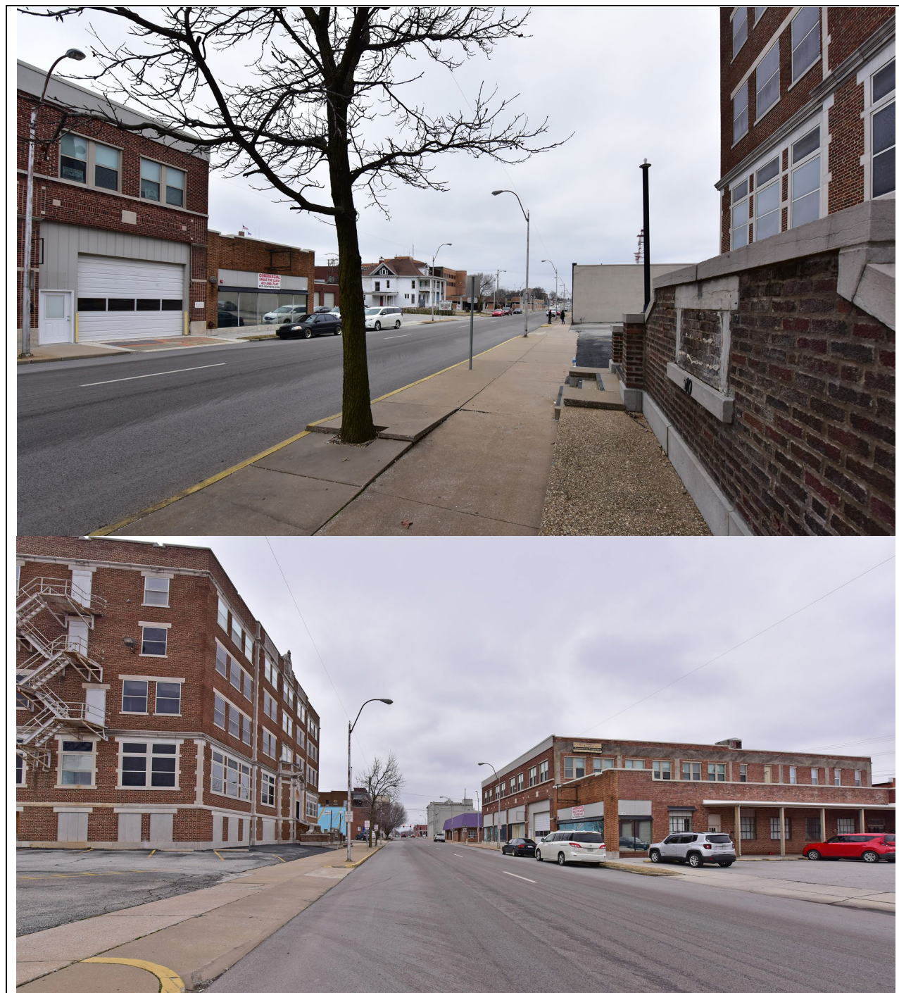
Figure 3. Contextual images of Wall Avenue, looking S (top) and north (bottom). Source: Brad Finch, January 2021.
