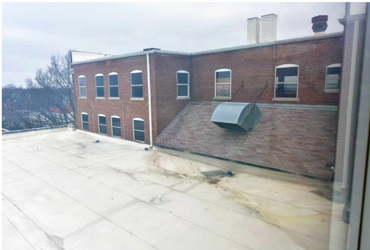
Figure 10. View from fourth floor, looking NW and showing the lightwell. Source: Brad Finch, January 2021.
