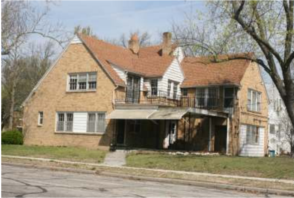
Southeast perspective looking northwest and showing 2-story porch in the angle of the rear ell, with cast metal railing and the possible in-fill of a former garage
