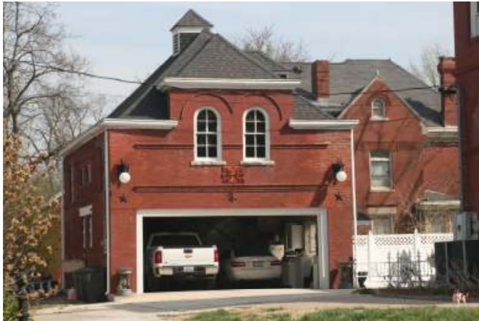
Carriage house behind main house, showing alteration to doors to accommodate overhead garage door.
