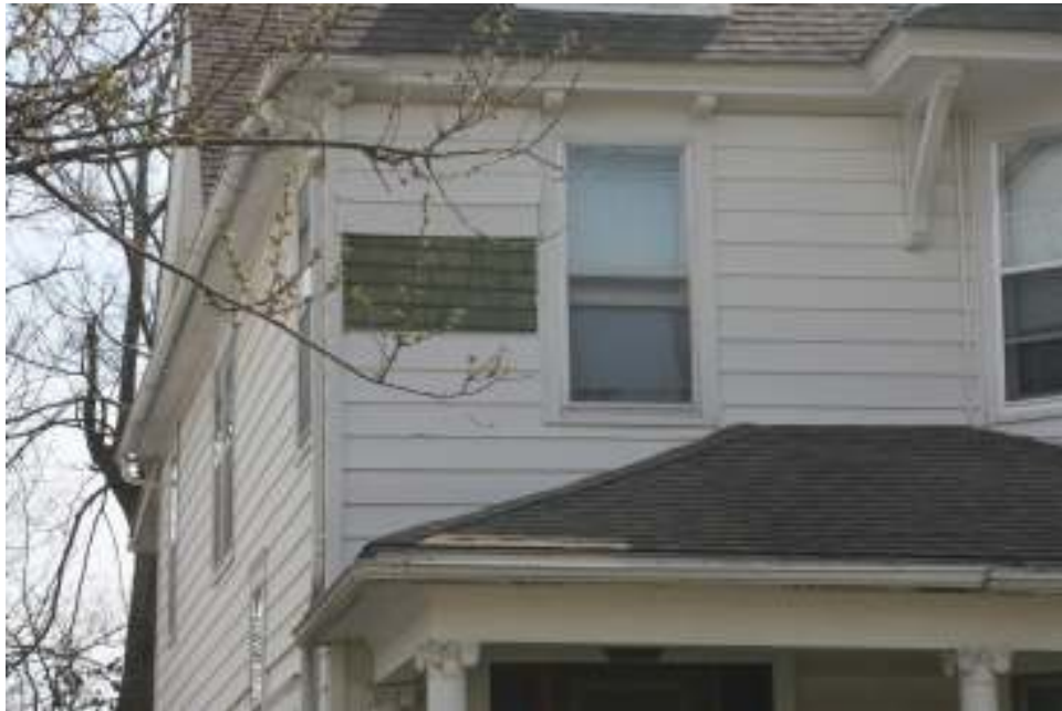
Detail of façade, showing original shingle finish under non-historic siding.
