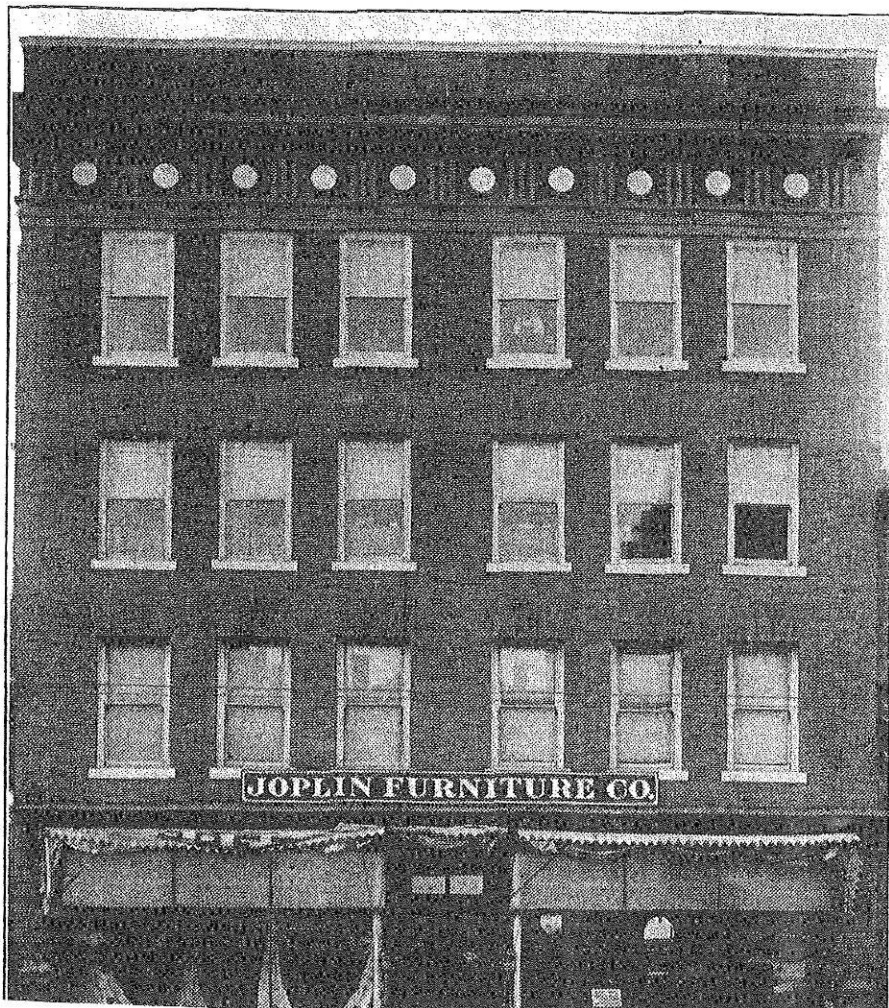
Figure 10: A 1912 Joplin Globe photograph of the Joplin Furniture Company after enlargement to four stories by architect August C. Michaelis. The adjacent north half of the combined structure would soon receive a two story expansion including a mirror image of the grand cornice and parapet shown above, completing the building. (from the collection of the Post Memorial Art Reference Library)
