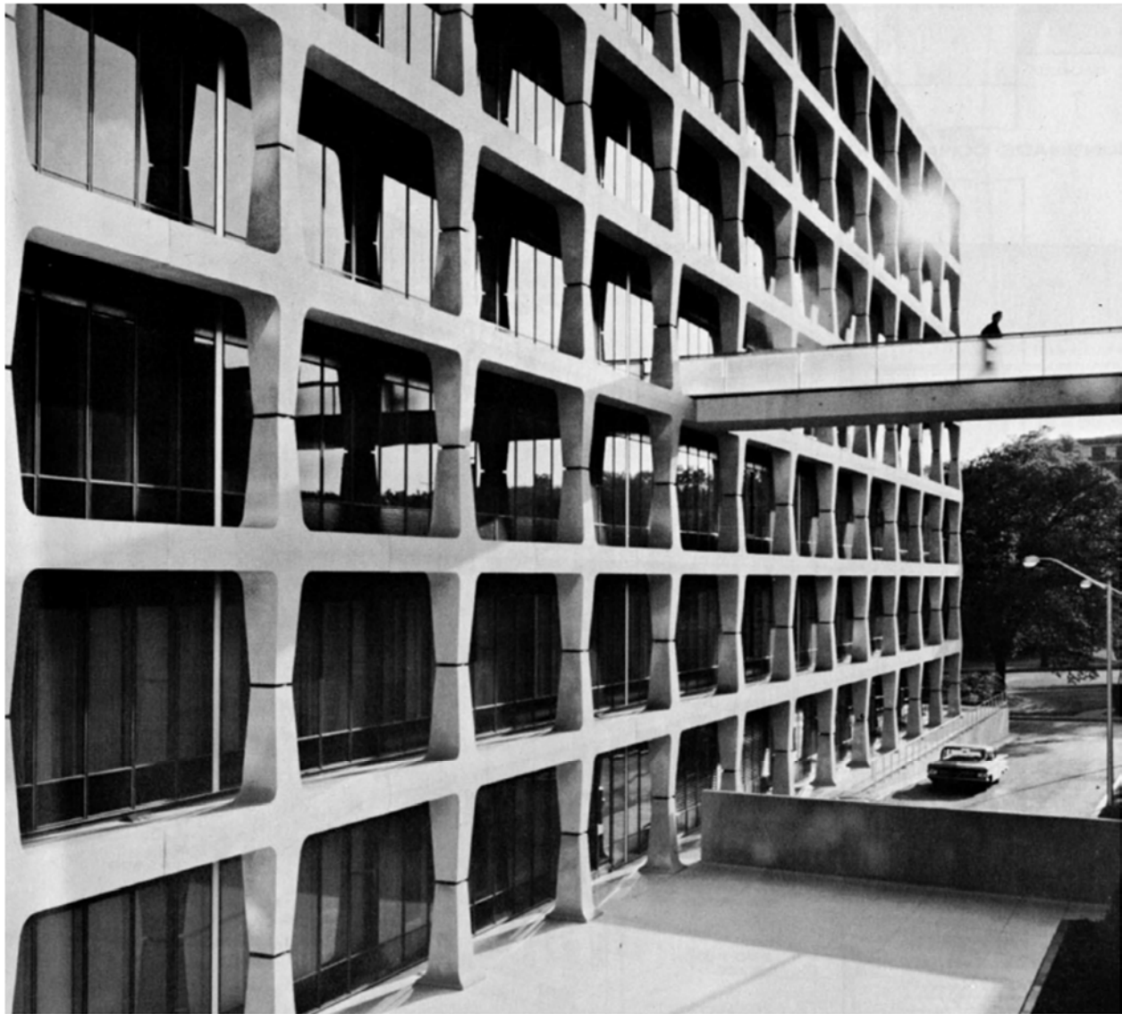
Figure 18. Looking southwest along the north elevation of the building, showing the historic condition of the skywalk. Source: "Peristylar Precast Structures by SOM," Progressive Architecture (September 1963): 133.
