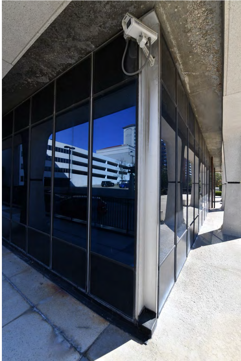
Figure 10. Inverted corner detail (northwest corner, first floor). Source: Finch, October 2023.
