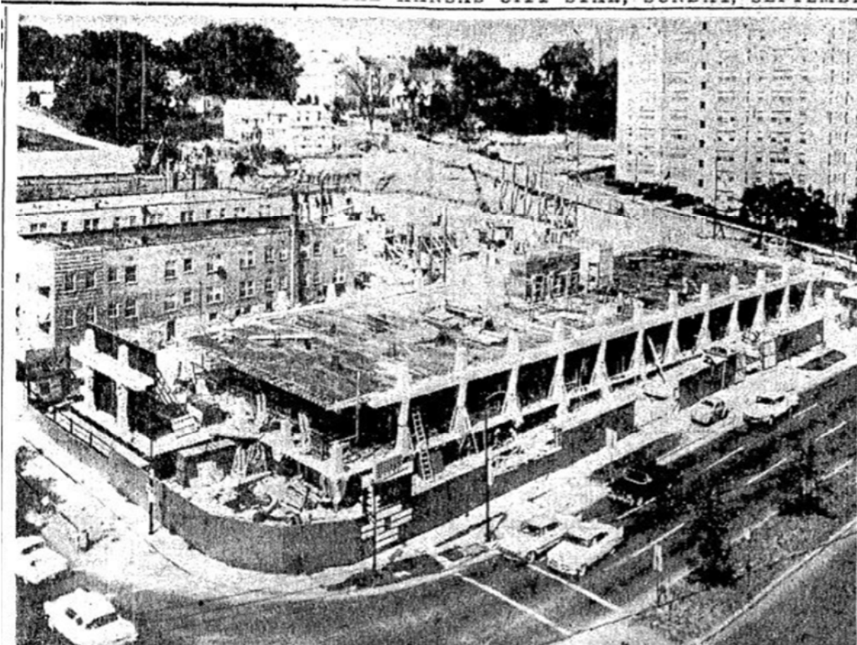
Figure 26. Construction photo, looking northeast (Source: Kansas City Star 10 September 1961: 84).
