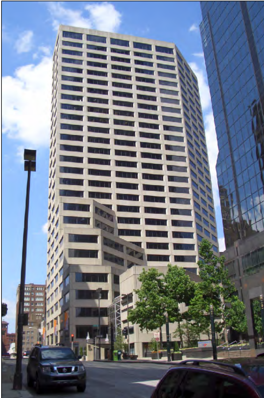
Figure 21. The 1977 City Center Square, 1100 Main Street, in 2008. SOM Architects. Source: Wikipedia, https://en.wikipedia.org/wiki/City_Center_Square#/media/File:City_Center_Square_Kansas_City_MO.jpg
