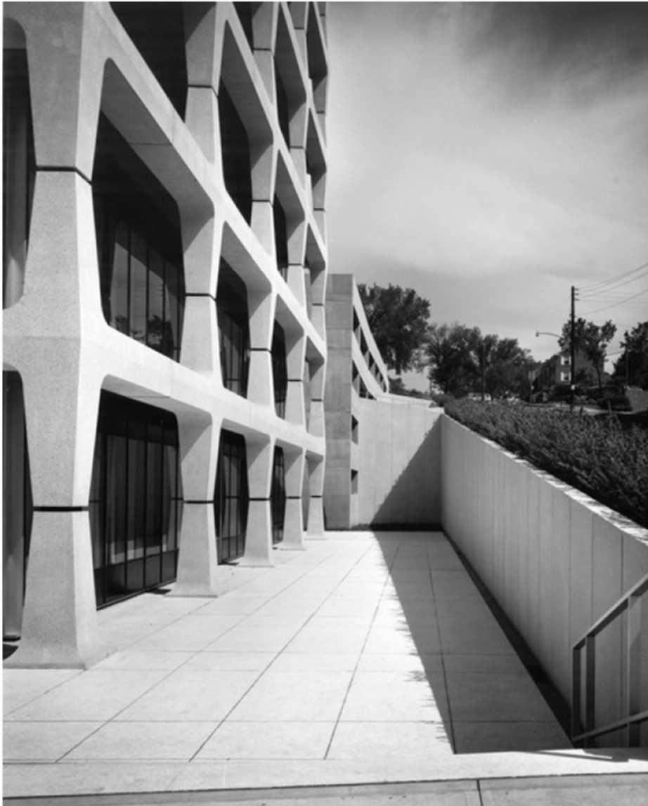
Figure 7. Looking north from the south sidewalk in 1962. Source: Ezra Stoller, photographer. ©Ezra Stoller | Esto, used with permission from SOM Library, Records and Information Services, Chicago.
