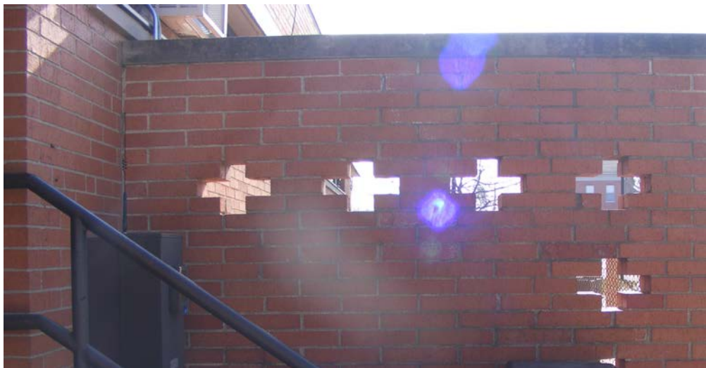
Figure 7. Detail of rear privacy wall near entry; view is south (Photo: Ruth Keenoy).
