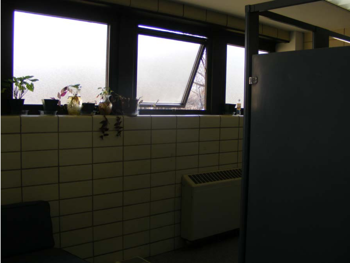
Figure 10. Wrapped windows retain original aluminum framing, as illustrated by the open window in this photograph (Photo: Ruth Keenoy).
