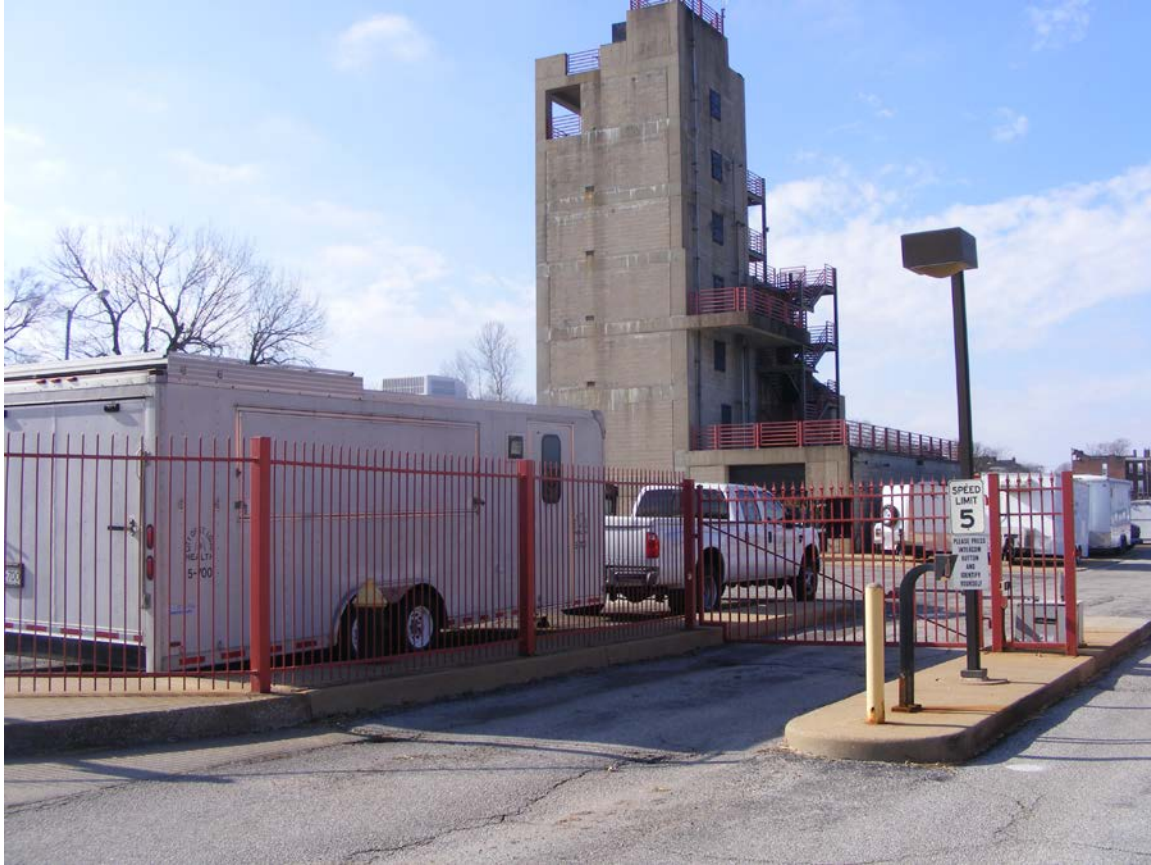
Figure 6. The parking lot, practice tower and associated entry gate/drive south of the former health clinic are outside of the property's National Register boundaries (Photo: Ruth Keenoy).
