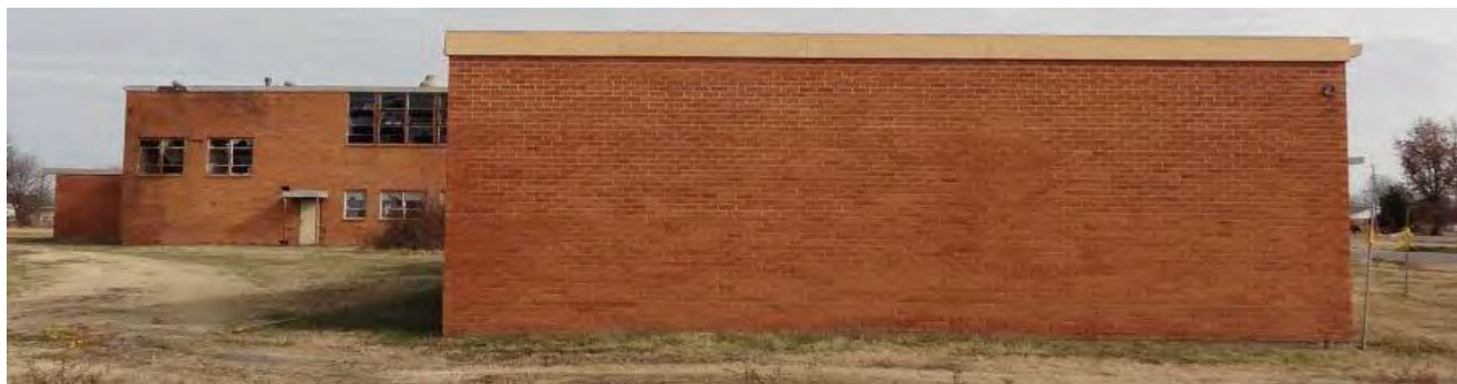
Figure 20. Showing the full west elevation of the library addition. Facing northeast. Photographed by the author, December 15-16, 2016.
