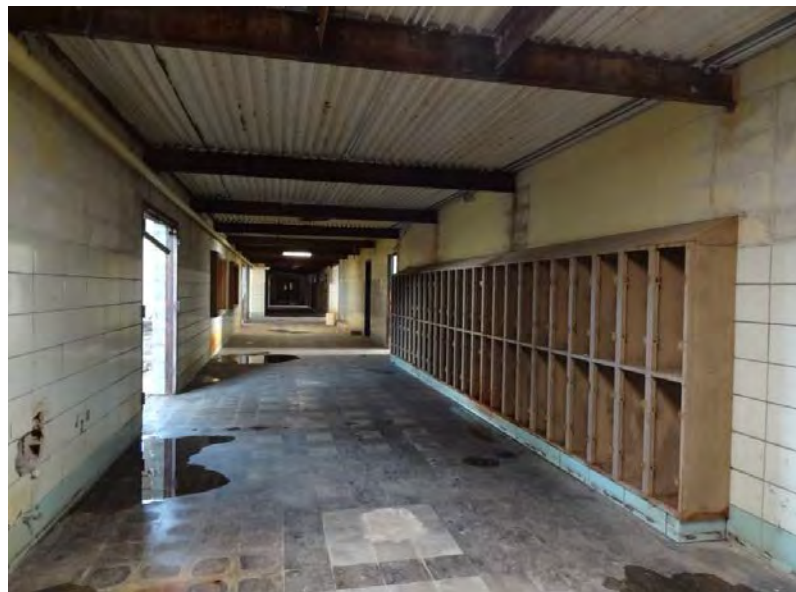
Figure 27. High school double-loaded corridor. Note wall tiling and lockers still largely intact. All lighting is from the expanses of windows located in the classrooms. Camera facing northeast. Photographed by the author, December 15-16, 2016.
