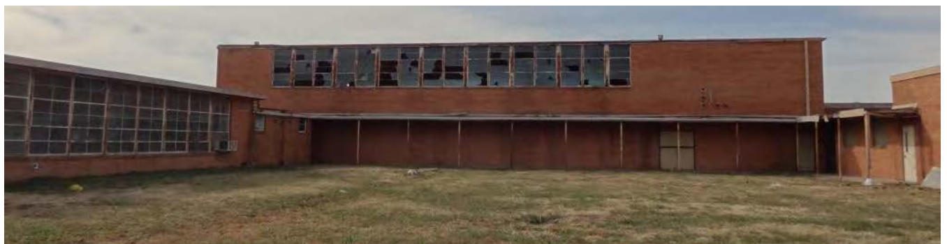
Figure 15. Northern elevation of east end of high school and eastern elevation of the two-story gymnasium. Camera facing southwest. Photographed by the author, December 15-16, 2016.
