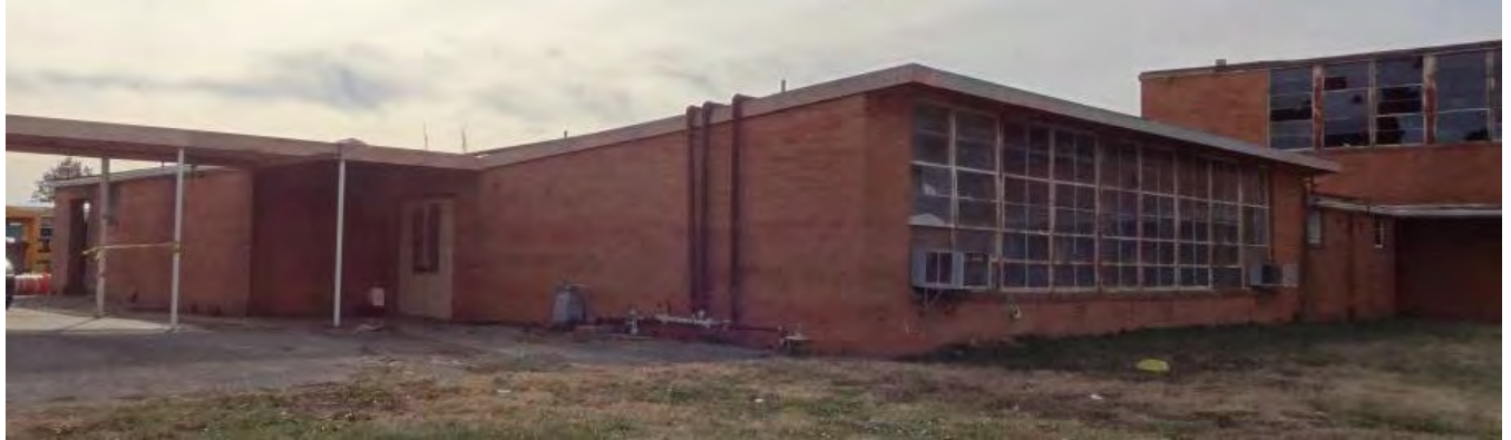
Figure 14. East elevation of the high school building, camera looking southeast. Photographed by the author, December 15-16, 2016.
