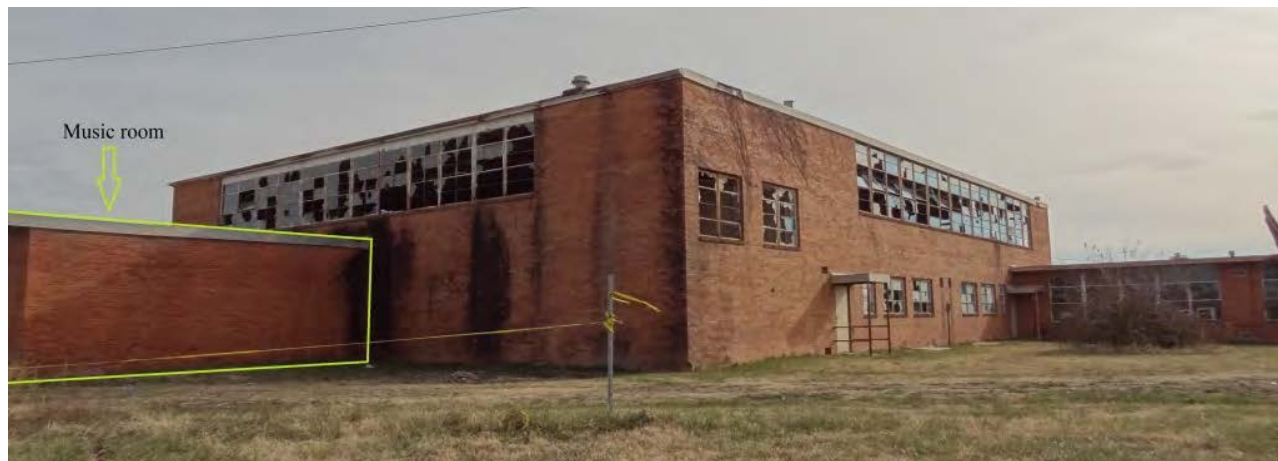
Figure 18. The west elevation of the music room, the north and west elevations of the gymnasium, and a portion of the one story western section of the high school (on the right). Facing southeast. Photographed by the author, December 15-16, 2016.
