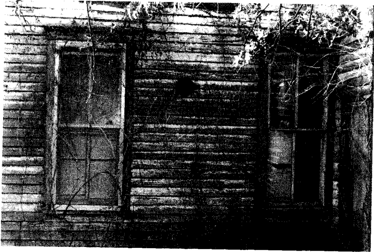
Photo 6: View of the southeastern part of Howard School, looking west. Original building is in center with two windows. Bathroom addition with door is to the extreme right. Note stovepipe flue between windows.
