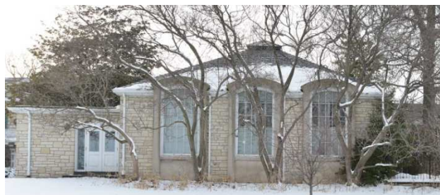
Figure 21: Resource 1, Block G, east elevation. Source: Brad Finch, F-Stop Photography, March 2015.
