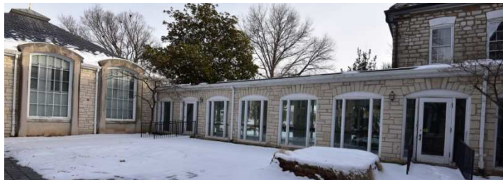
Figure 23: Resource 1, Block G, north and west elevations. Source: Brad Finch, F-Stop Photography, March 2015.
