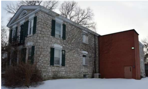
Figure 15: Resource 1, Block E, northeast corner. Source: Brad Finch, F-Stop Photography, March 2015.
