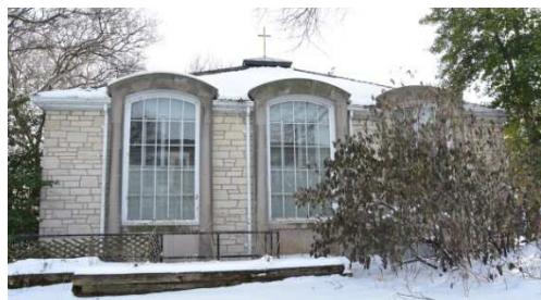
Figure 20: Resource 1, Block G, north elevation. Source: Brad Finch, F-Stop Photography, March 2015.
