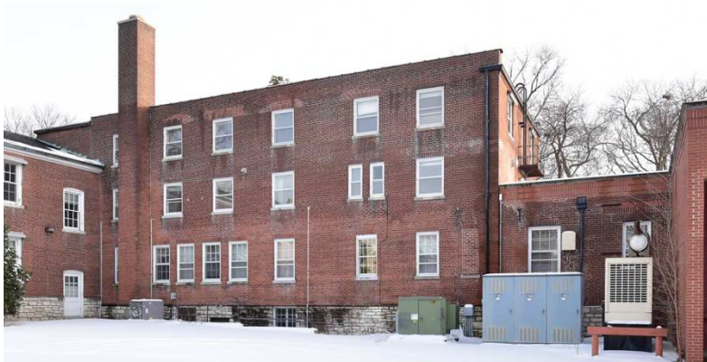
Figure 11: Resource 1, Block C, north elevation. Source: Brad Finch, F-Stop Photography, March 2015.
