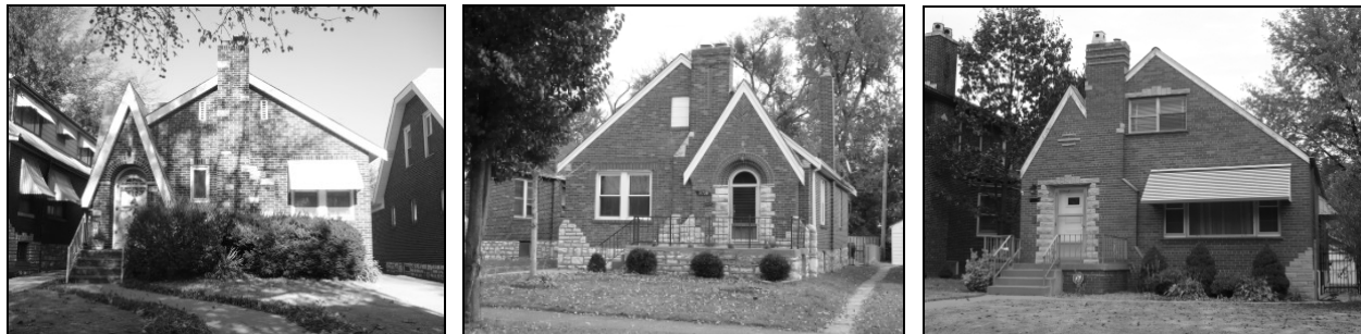
Figure 13: 3833 Dover (left; J. Myers, 1930); 5708 Arendes (no architect listed, 1939); and 3885 Federer Place (Bert Luer, 1955). Source: Holly Hills Survey, 2009. Source: Holly Hills survey, 2009.
