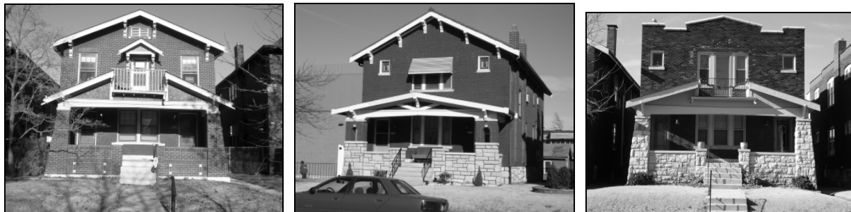
Figure 22: Examples of Craftsman-style two-family buildings. From left to right: 3953 Fillmore (E. Winke, 1928); 3905 Wilmington (architect unknown, 1928); 5925 Coronado (H. Tyler, 1928), with a vernacular shaped parapet roof and a Craftsman-style porch. Source: Holly Hills Survey, 2009.
