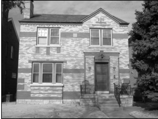
Figure 17: Left: Colonial Moderne at 4065 Holly Hills Blvd. (Henry Schaumburg, 1941). Source: Holly Hills Survey, 2009.
