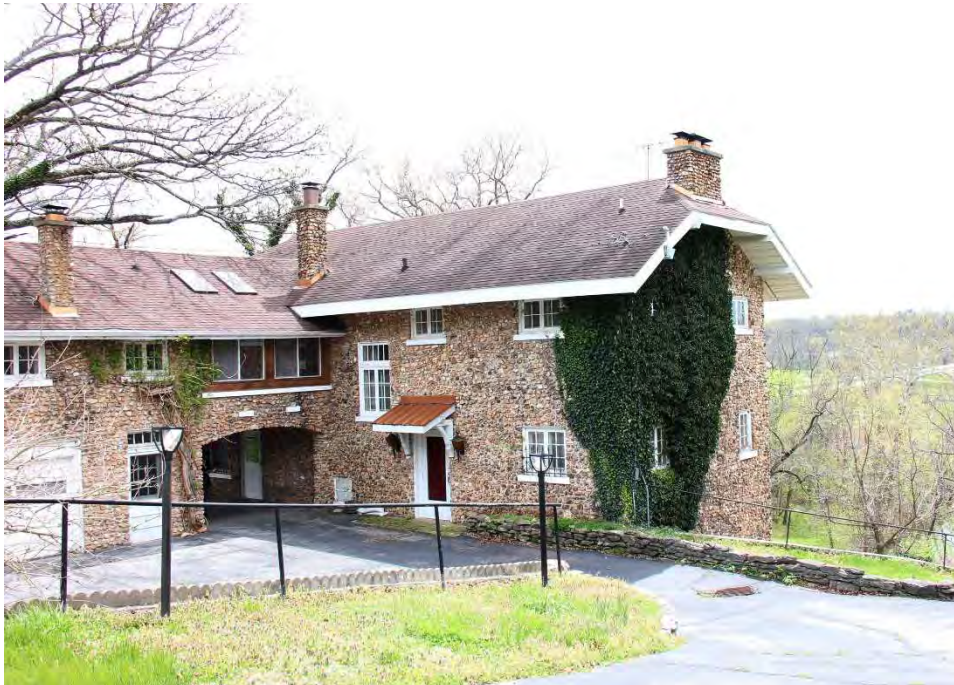
6. Inside corner of the house, north and west walls. Camera facing southeast.
