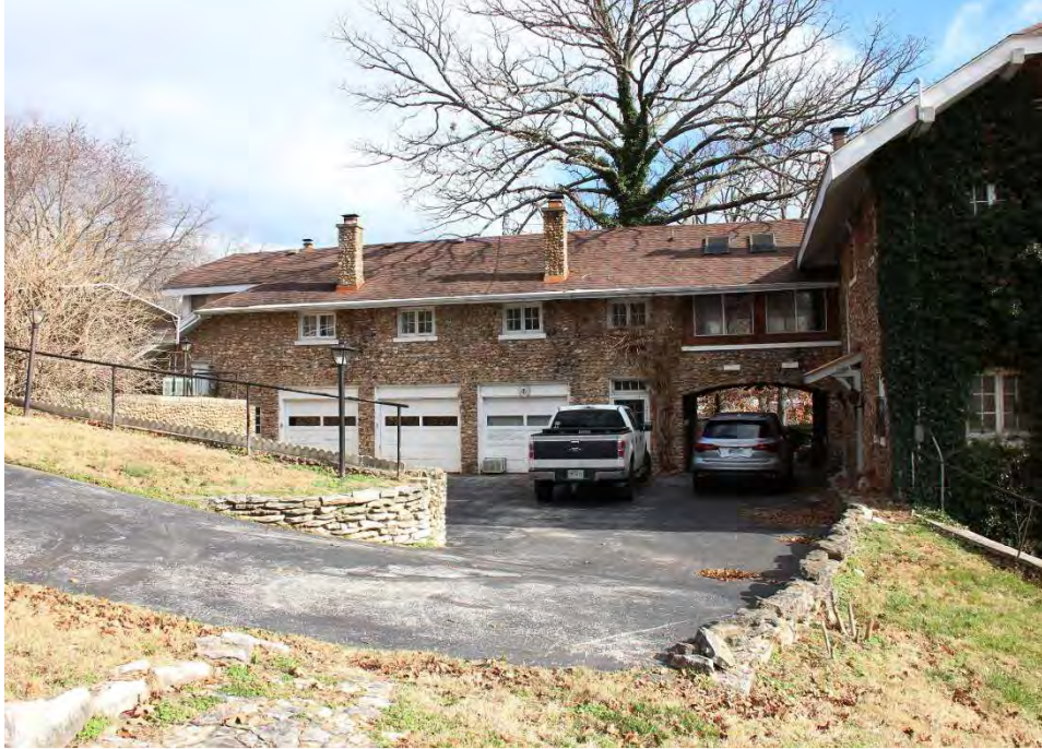
5. West wall of the house with breezeway. Camera facing east.
