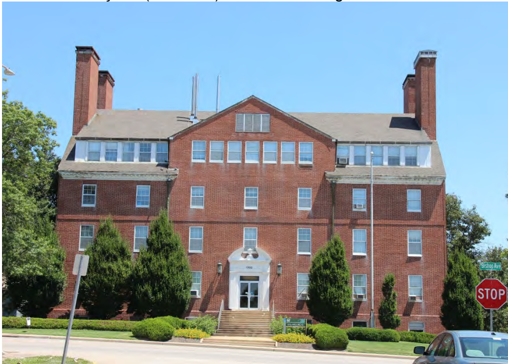
1 of 18: Façade (west wall). Camera looking east.
