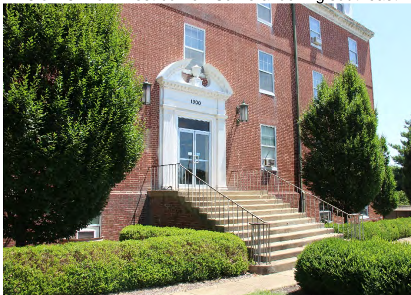
8 of 18: Northwest corner. Camera looking southeast.
