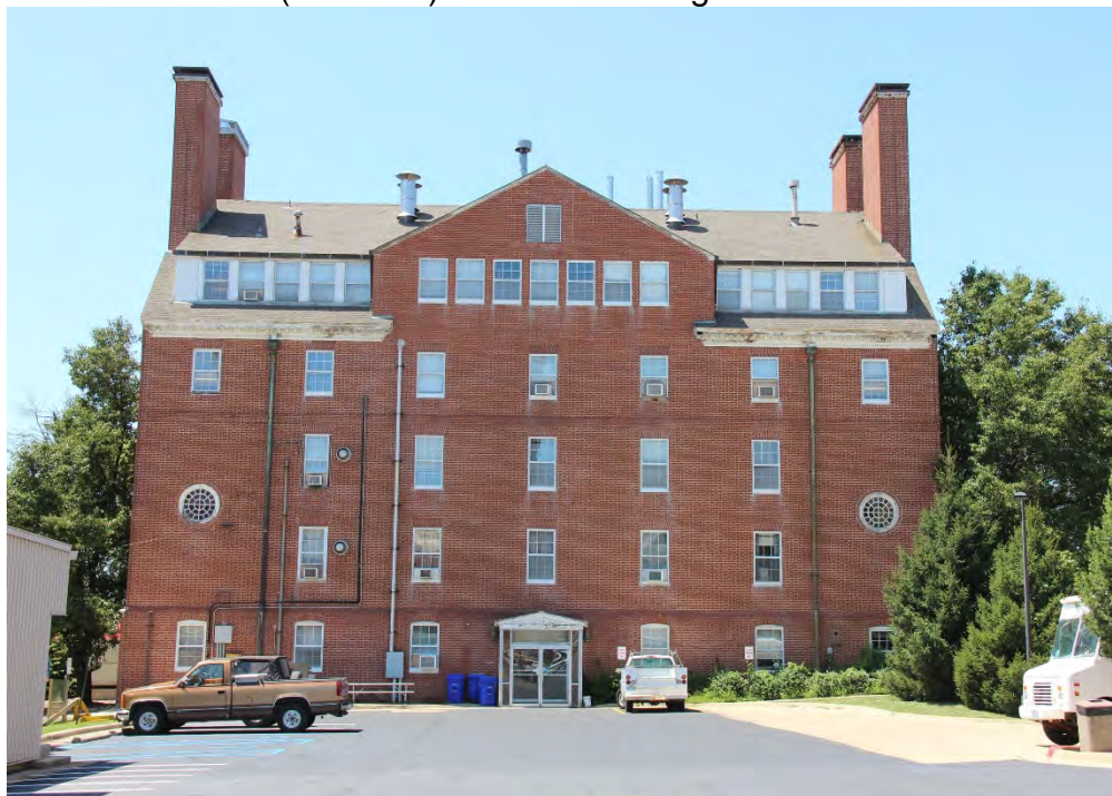
6 of 18: Back (east wall). Camera looking west.
