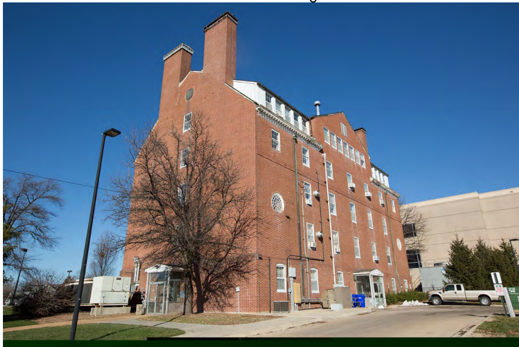
5 of 18: Southeast corner. Camera looking northwest.
