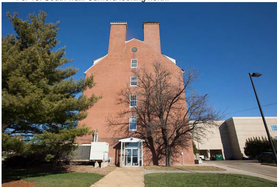
4 of 18: South wall. Camera looking north.
