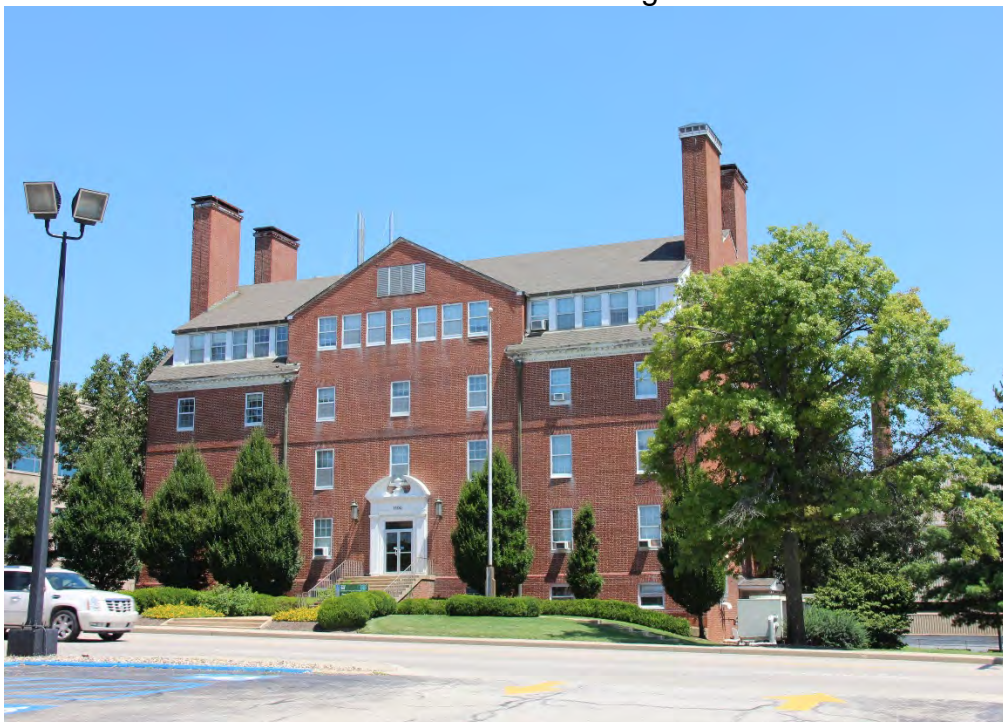
2 of 18: Southwest corner. Camera looking northeast.
