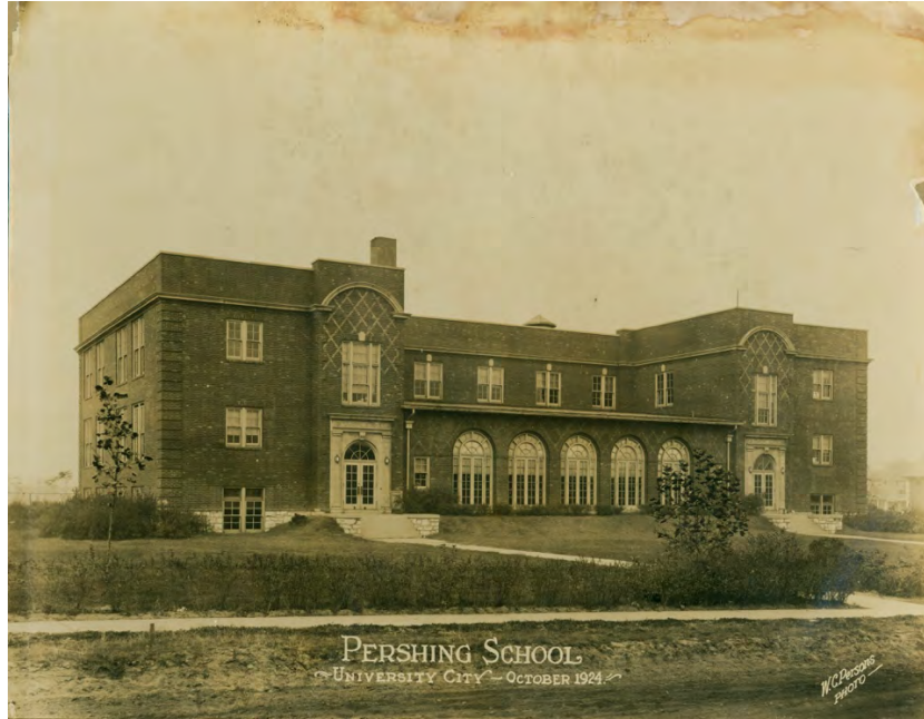
a. Pershing School in 1924 with Original Flat Roof.
