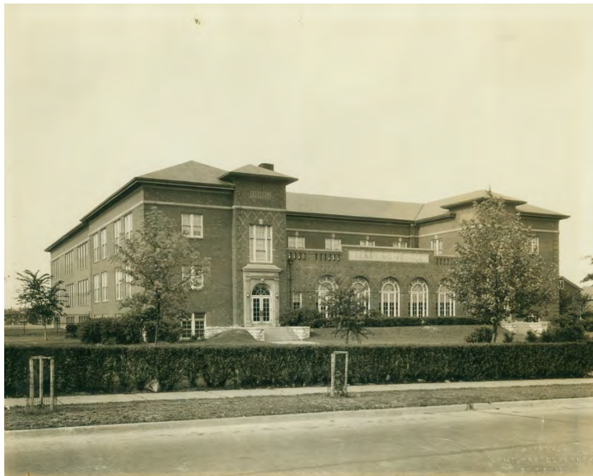
b. Pershing School, circa 1935, With New Hipped Roof.
