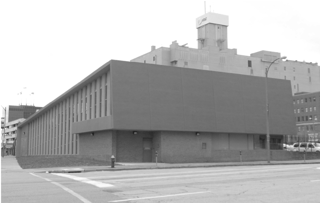
Figure 5: Jefferson Bank and Trust Company Building (1955; Bank Building and Equipment Corporation). (Source: Preservation Research Office photograph, 2013.)
