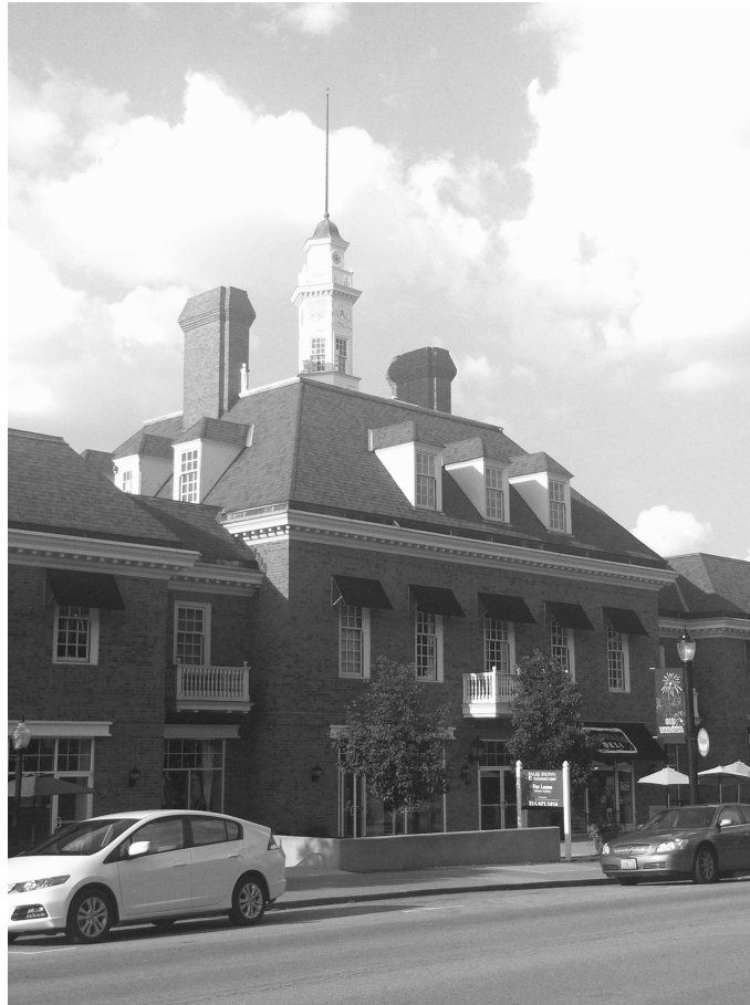
Figure 11: The Reliance Life Insurance Company Building (1963; Winkler & Thompson). (Source: Preservation Research Office photograph, 2013.)
