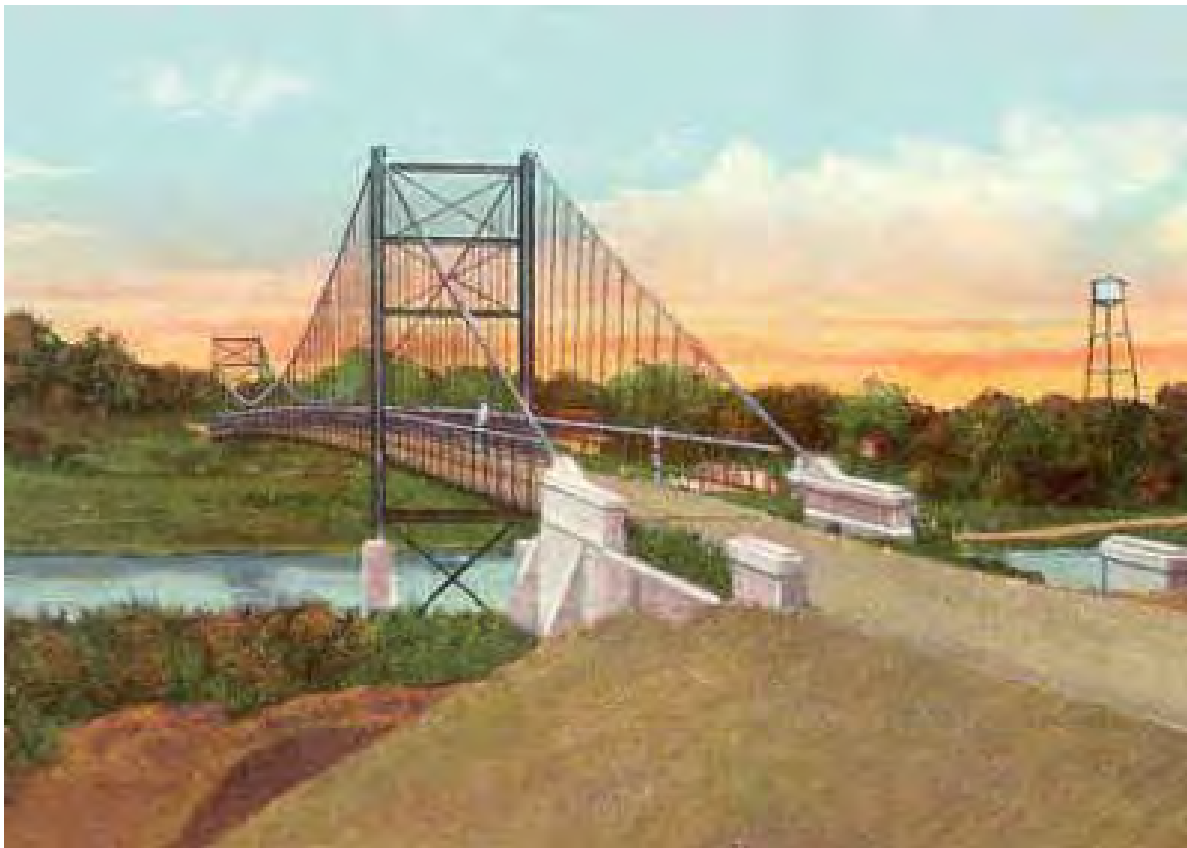
Figure 13 - Warsaw Upper Bridge, Benton County, Missouri
