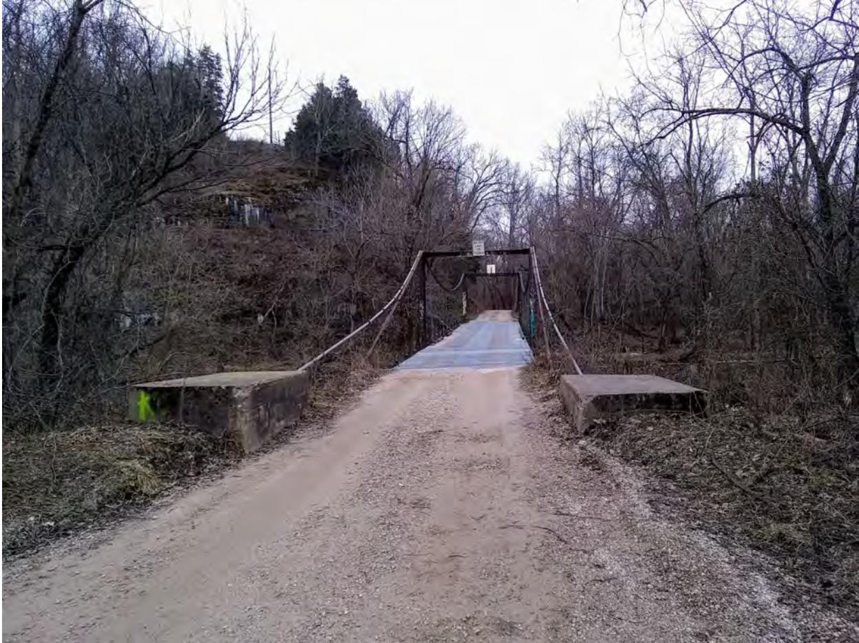
Figure 11 - Mill Creek Bridge (Miller County, Missouri) Source: Photo taken by Kelly Warman-Stallings, February 15, 2020
