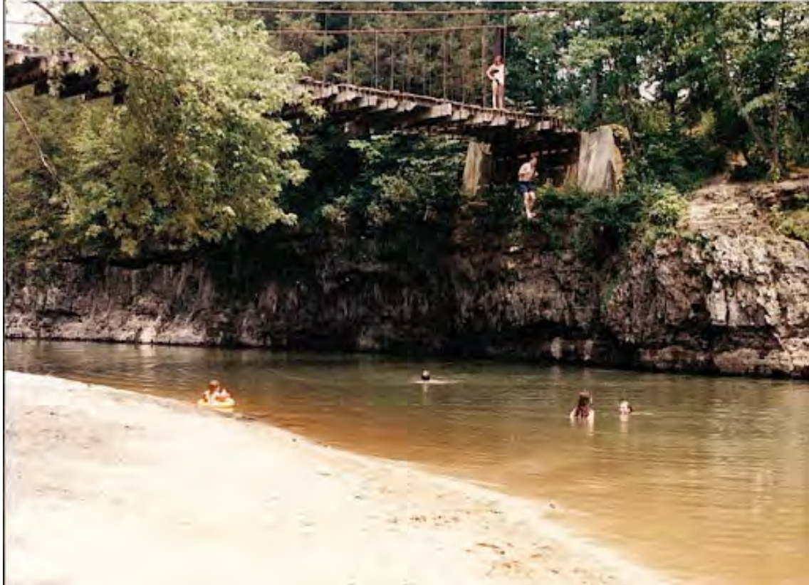
Figure 19 - Boeckman Bridge, Miller County, Missouri Source: Miller County Museum and Historical Society website. "Bridges of Miller County" article. Photo credit unknown. www.millercountymuseum.org/bridges.html
