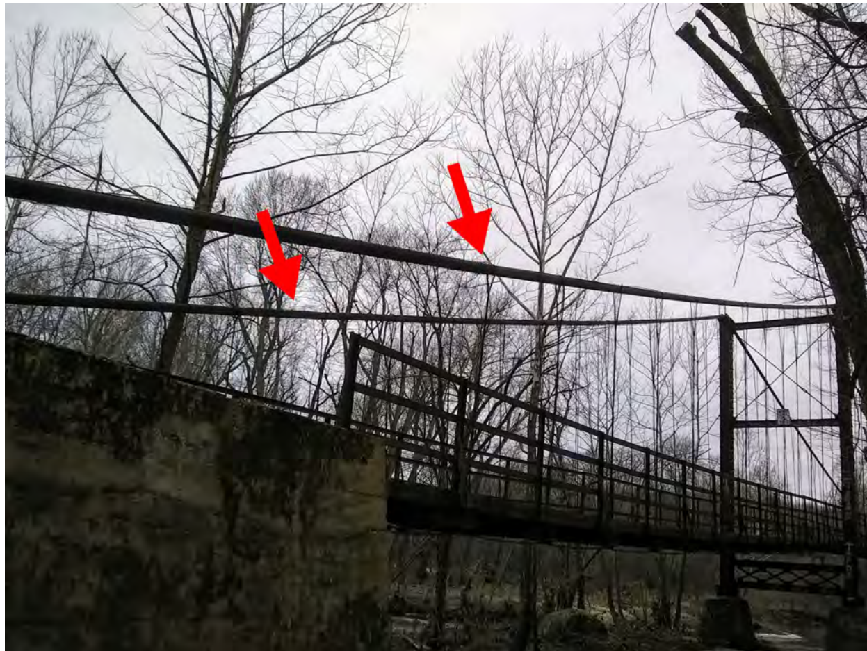
Figure 2 - Main Suspension Cables, highlighted with red arrows Source: Photo taken by Kelly Warman-Stallings, February 15, 2020
