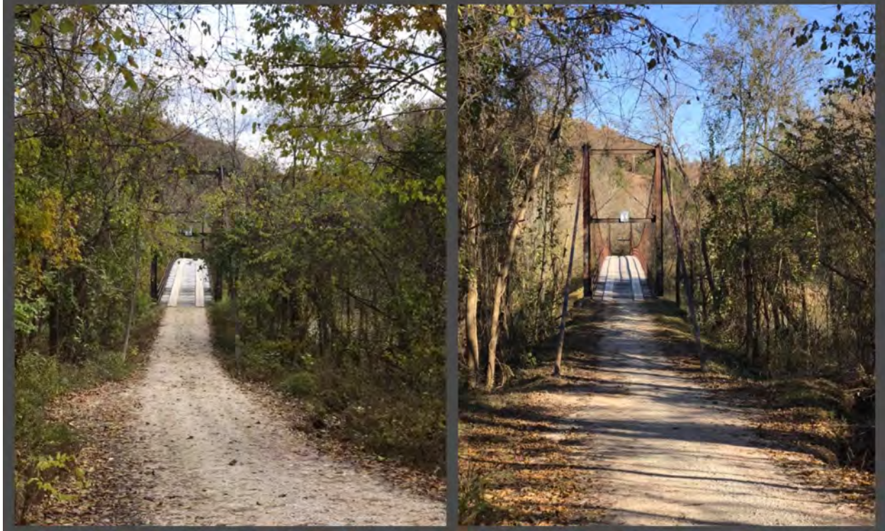
Figure 8 - West end of Grand Auglaize Bridge before clean-up (left), West end of Grand Auglaize Bridge after clean-up (right).
