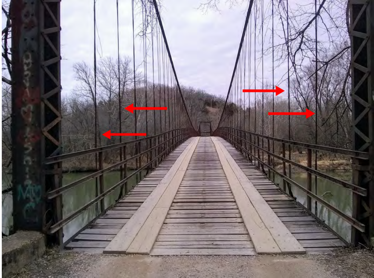
Figure 3 - Hanger Cables, highlighted with red arrows Source: Photo taken by Kelly Warman-Stallings, February 15, 2020
