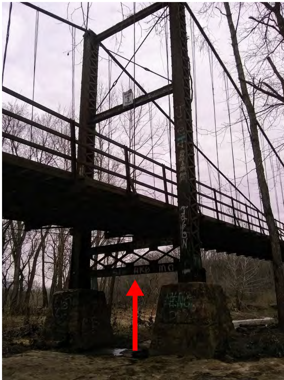
Figure 5 - East Tower, with highlighted red arrow
