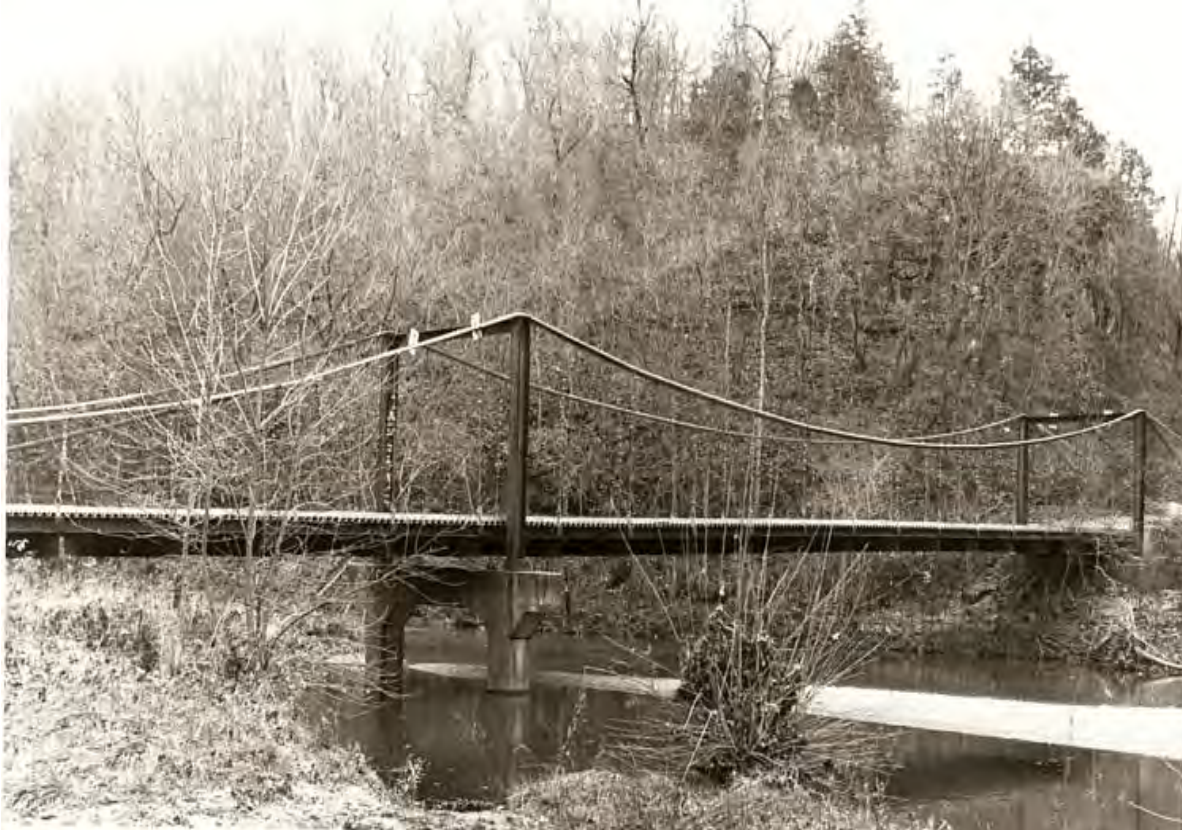
Figure 18 - Mill Creek Bridge, Miller County, Missouri Source: Miller County Museum and Historical Society website. "Bridges of Miller County" article. Photo credit unknown. www.millercountymuseum.org/bridges.html
