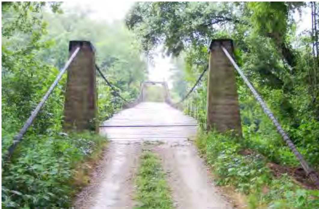
Figure 17 - Kliethermes Bridge, Miller County, Missouri
