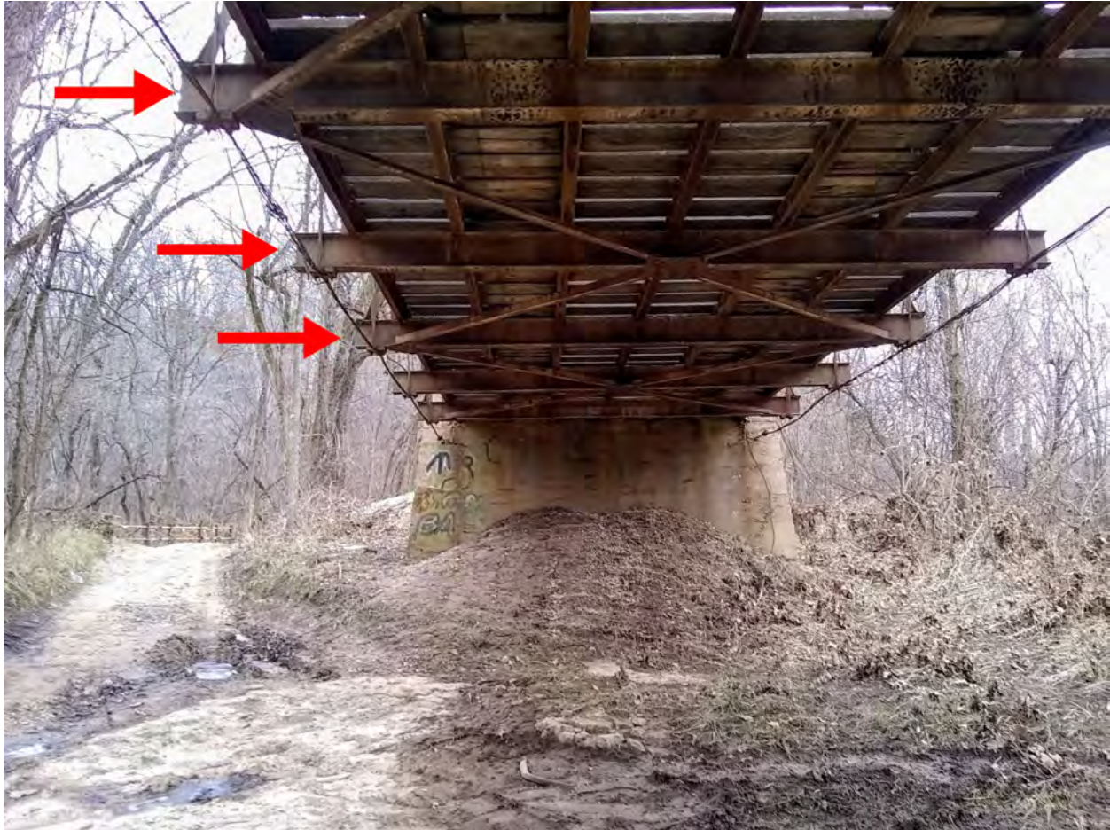
Figure 6 - Stringers, with highlighted red arrows
