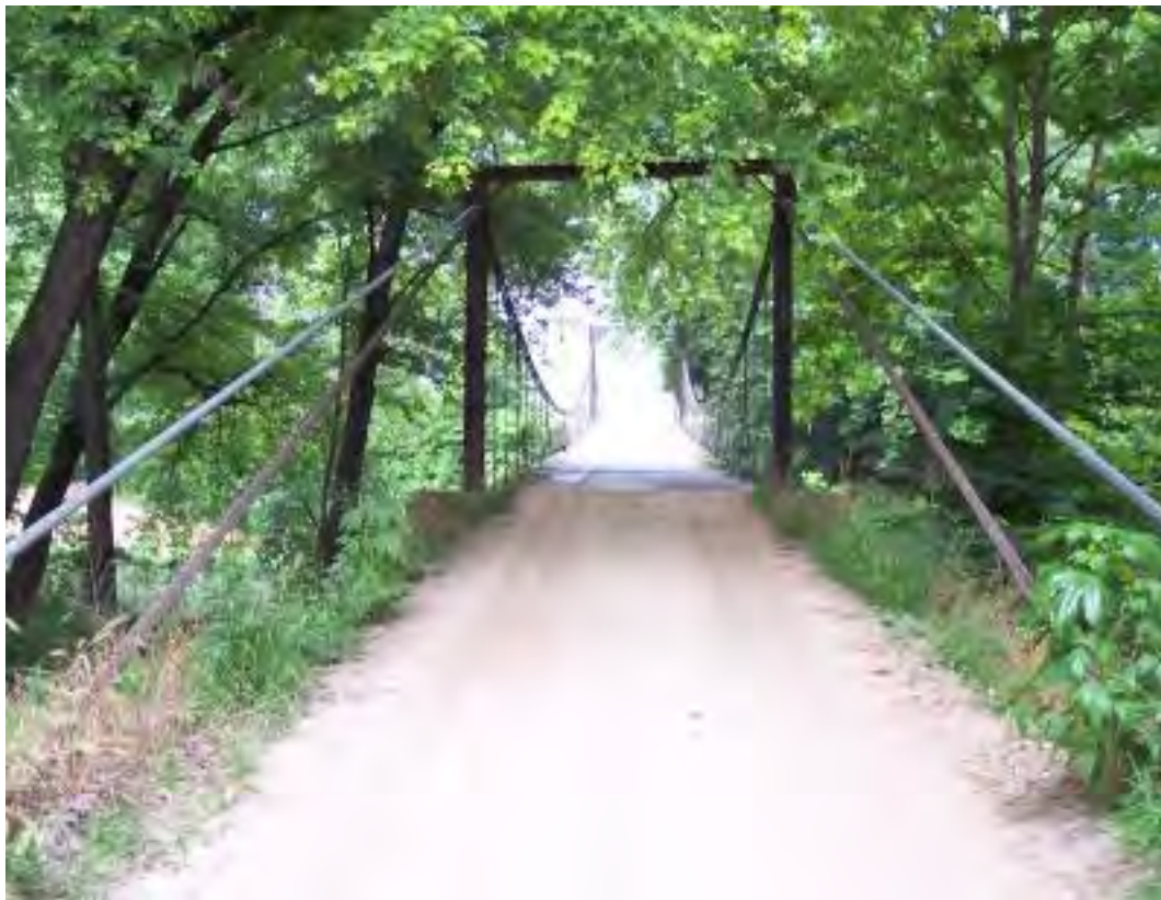
Figure 15 - Kemna Bridge, Miller County, Missouri
