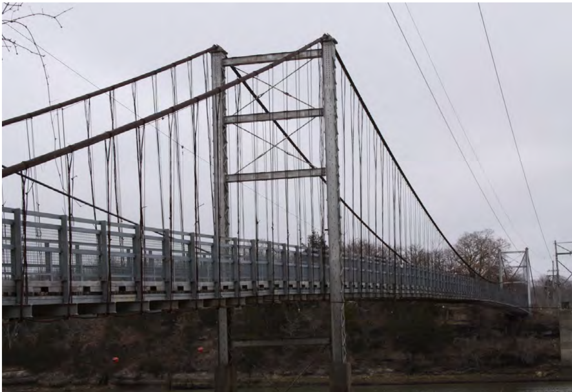
Figure 20 - Warsaw Upper Bridge (Benton County, Missouri)
