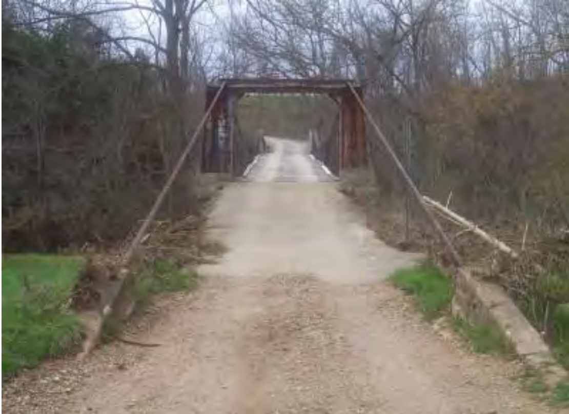
Figure 16 - Buechter Bridge, Miller County, Missouri
