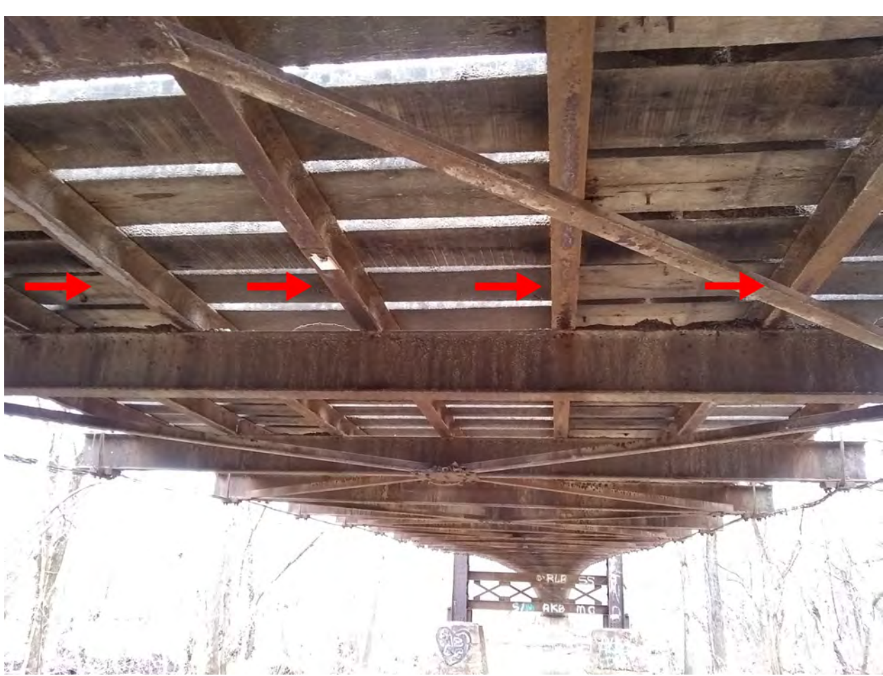
Figure 4 - Floor Beams, with highlighted red arrows
