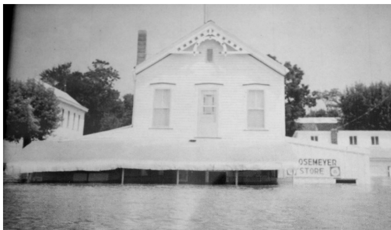
Figure No. 6: The Glosemeyer General Store during the 1993 flood, view north, photograph possibly by Linus Glosemeyer, on display at the Peers Store.
