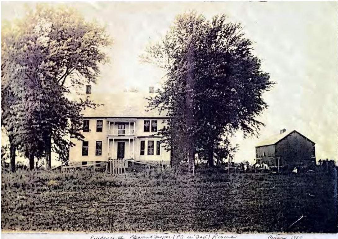
Figure 12. Top: House and barn ca. 1920. Bottom: House ca. 1920, with view of rear porch in background. (Rogers family photos in Meyer family collections.)
