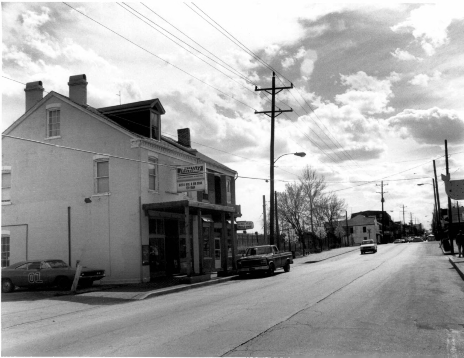
STREETSCAPE, 1100 BLOCK N. SECOND 1100-06, LEFT FOREGROUND CAMERA FACING SOUTHEAST
