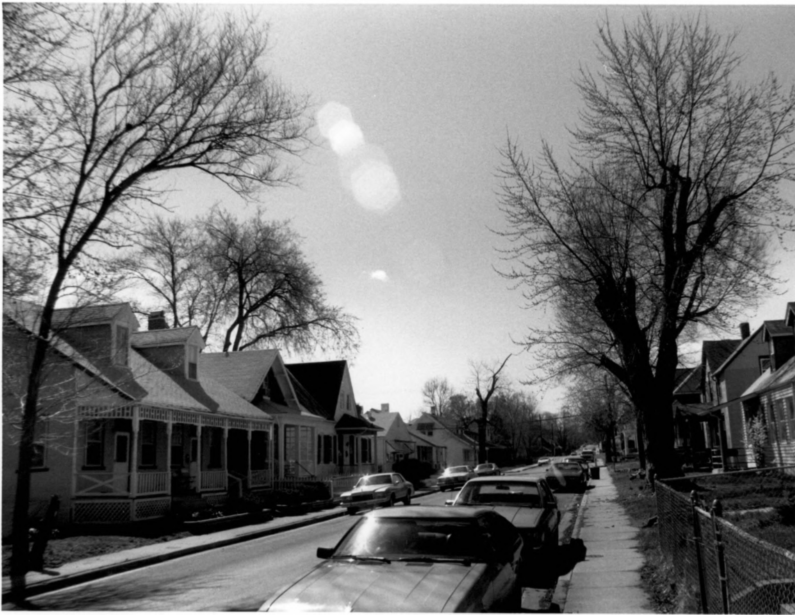
STREETScape, 1300 BLOCK N. THIRD 1320, LEFT FOREGROUND CAMERA FACING SOUTH
