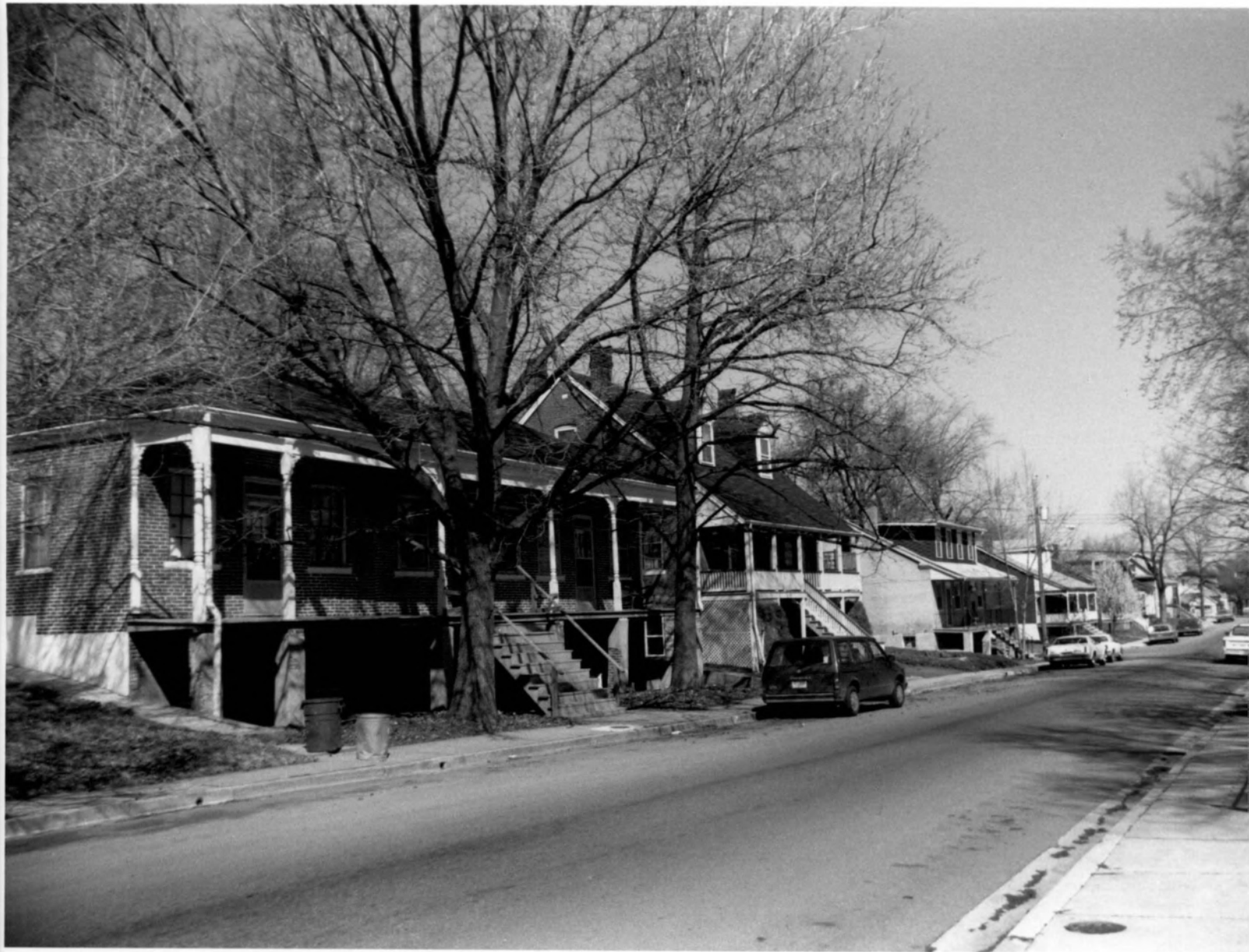
STREETScape, W.S. 1000 BLOCK N. THIRD 1013, LEFT FOREGROUND CAMERA FACING NORTHWEST
