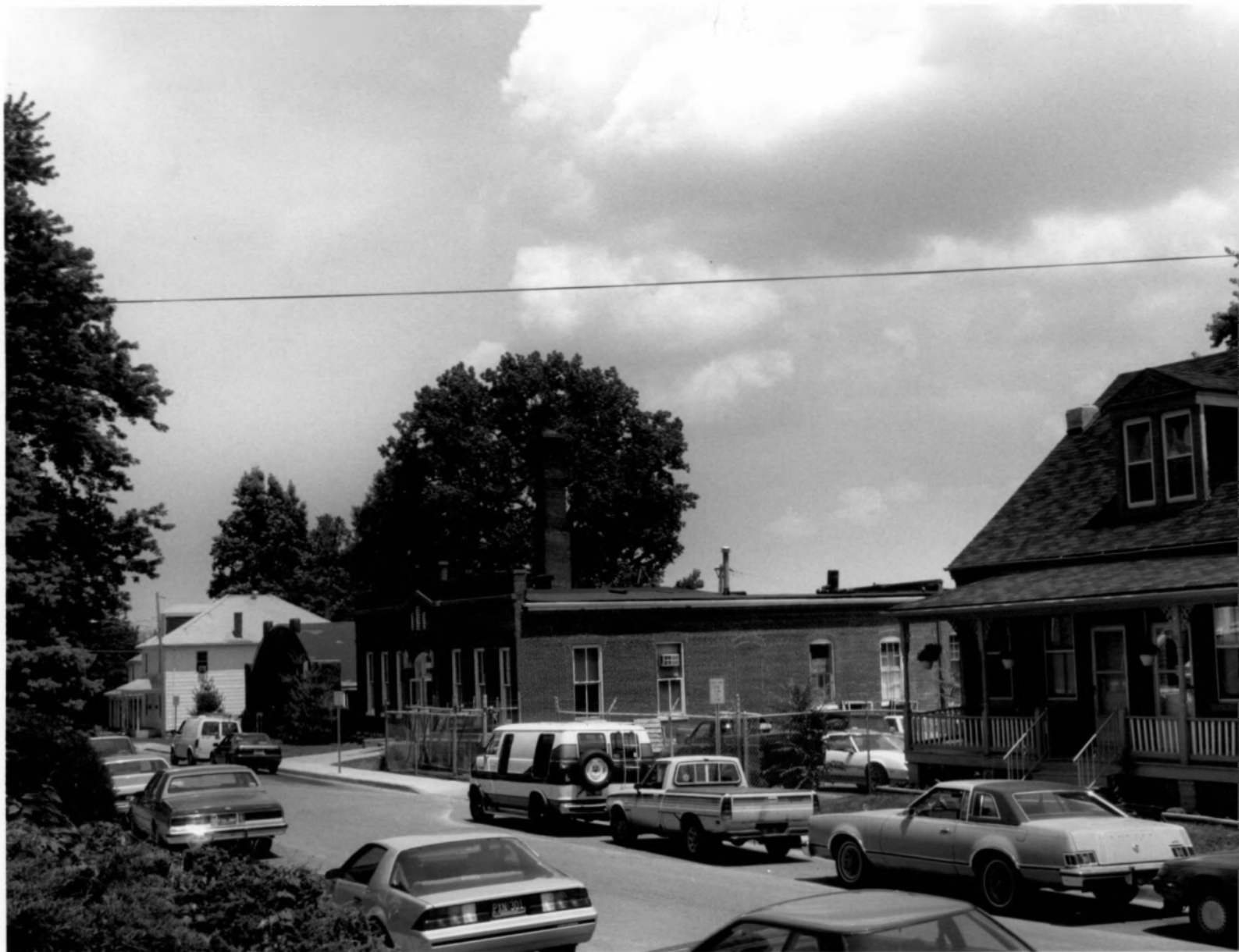
STREETScape, E.S. 700 BLOCK N. THIRD 706, FOREGROUND CAMERA FACING NORTHEAST
