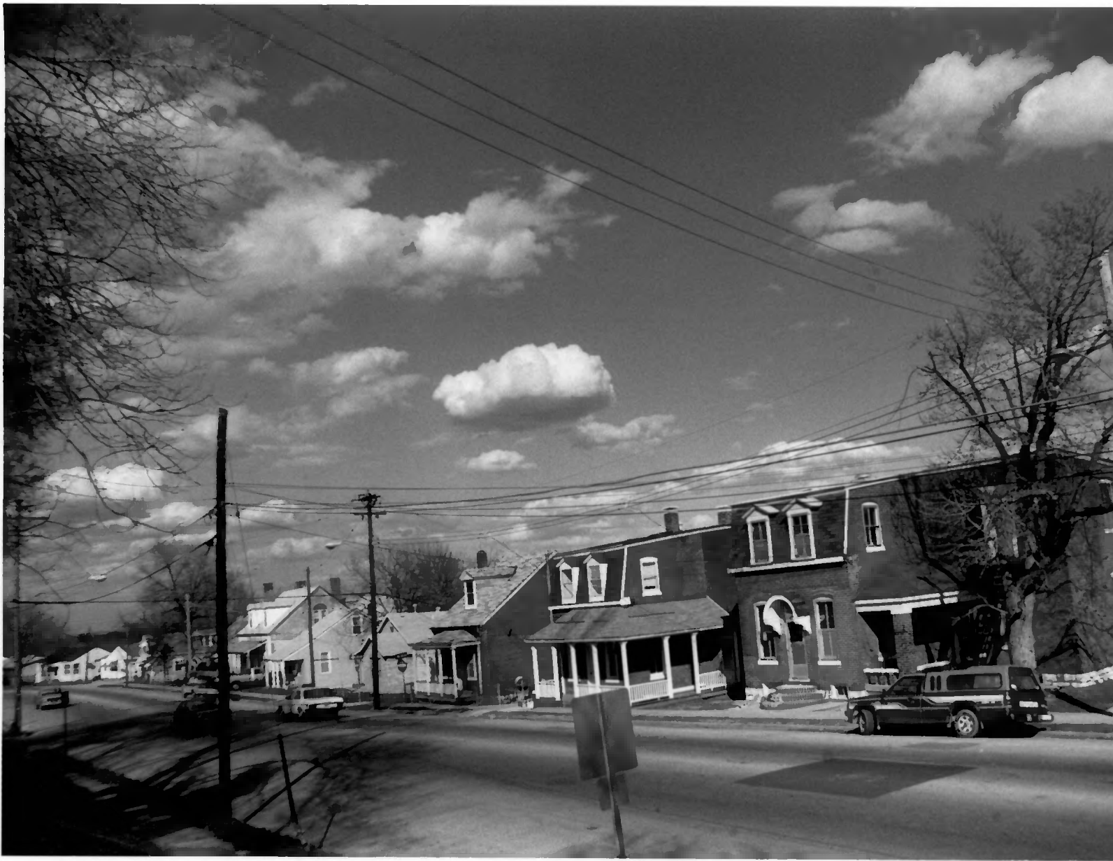
STREETSCAPE, E.S. 1200 BLOCK N. FIFTH 1216 N. FIFTH, FOREGROUND CAMERA FACING NORTHEAST
