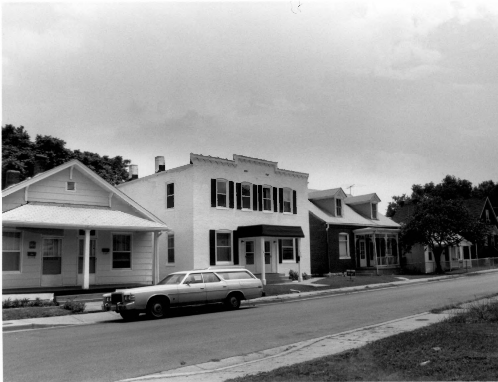
STREETScape, E.S 1400 BLOCK N. THIRD 1428, LEFT CAMERA FACING SOUTHEAST
