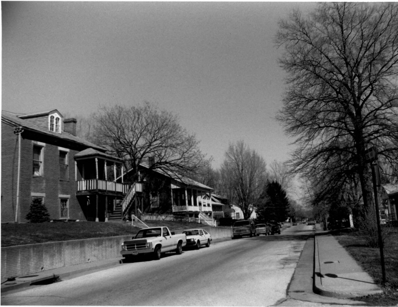
STREETSCAPE, W.S. 1000 BLOCK N. FOURTH 1003, LEFT FOREGROUND CAMERA FACING NORTHWEST
