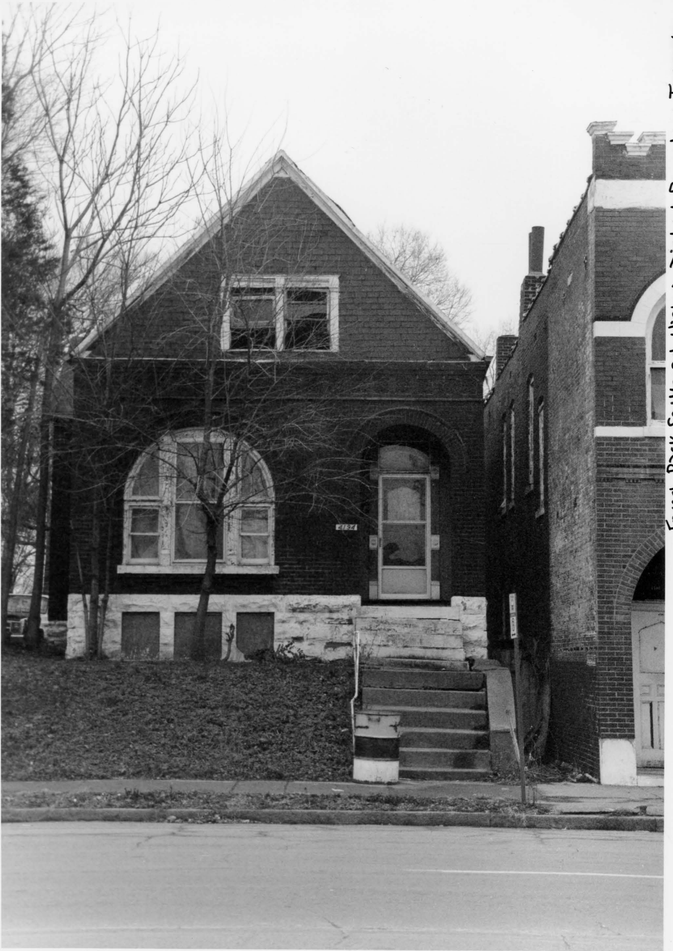
Forest Park Southeast Historic District Boundary Increase St. Louis (Independent City), MO #7
