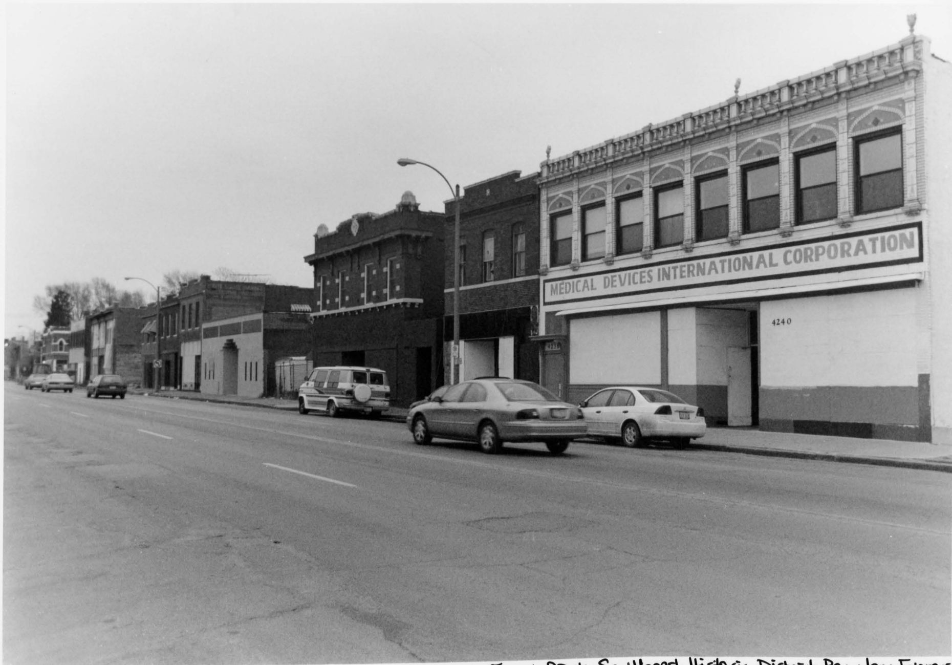
Forest Park Southeast Historic District Boundary Increase St. Louis (Independent City), MO #9
