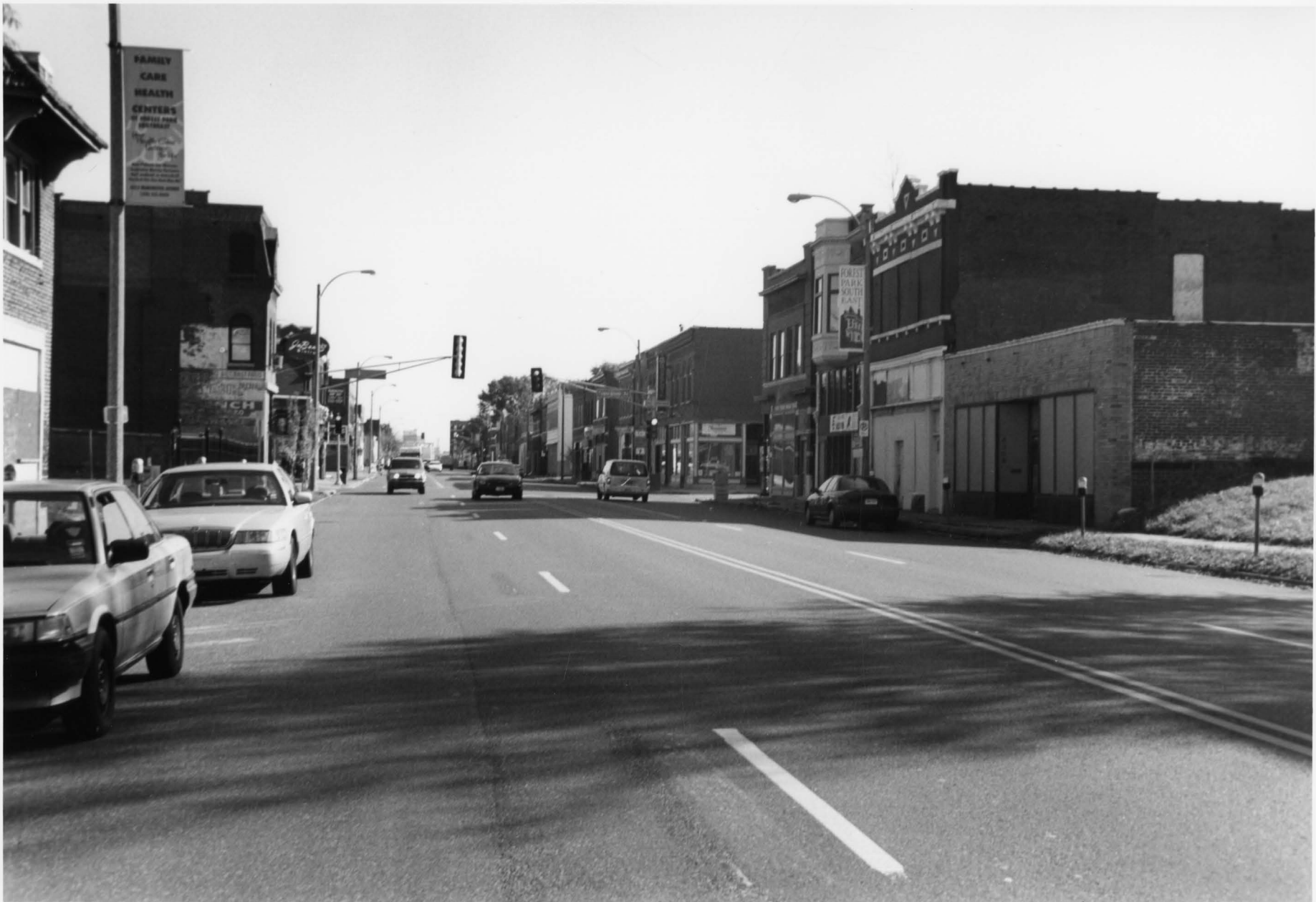
Forest Park Southeast Historic District Boundary Increase St. Louis (Independent City), MO.
