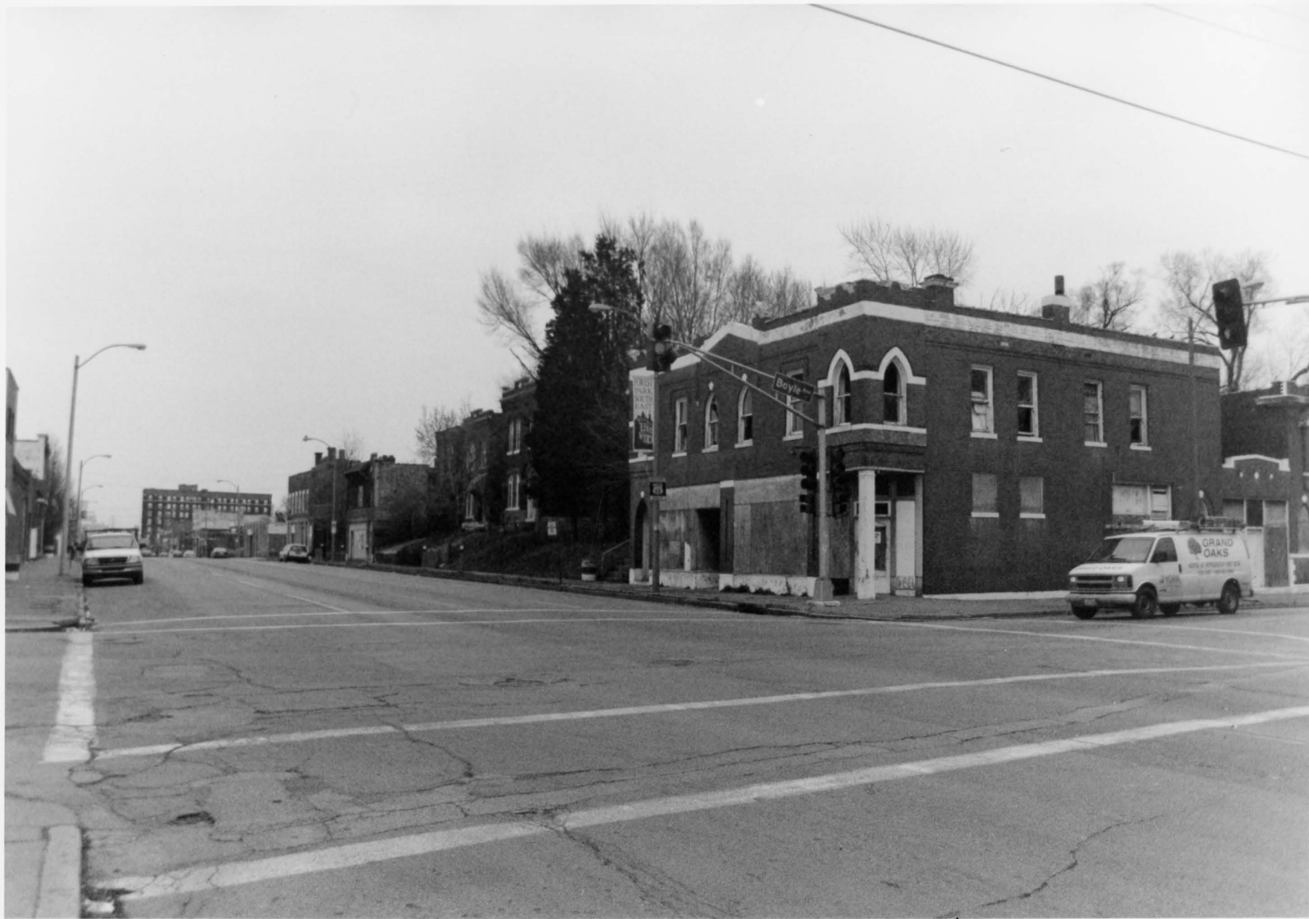
Forest Park Southeast Historic District Boundary Increase St. Louis (Independent City), MO # 8
