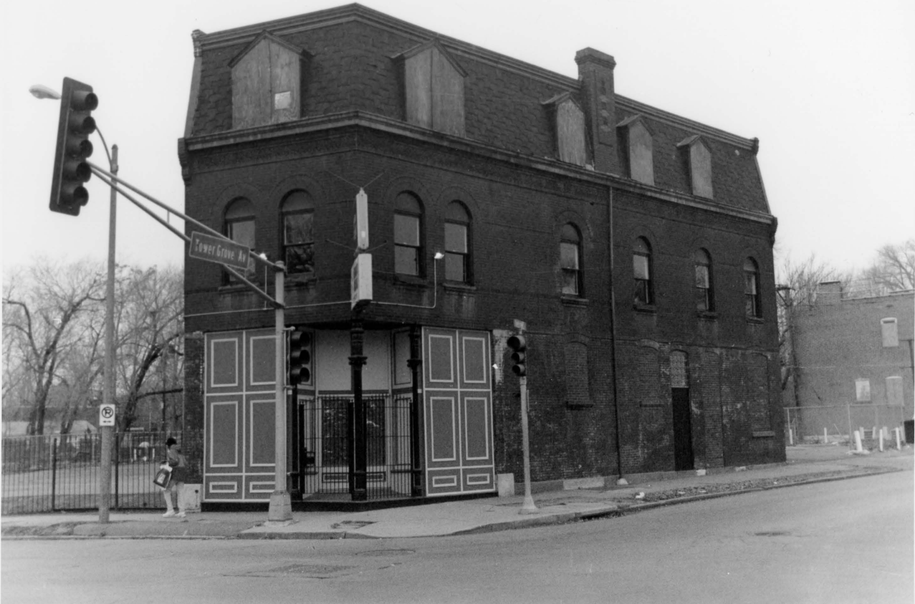
Forest Park Southeast Historic District Boundary Increase St. Louis (Independent City), MO #2
