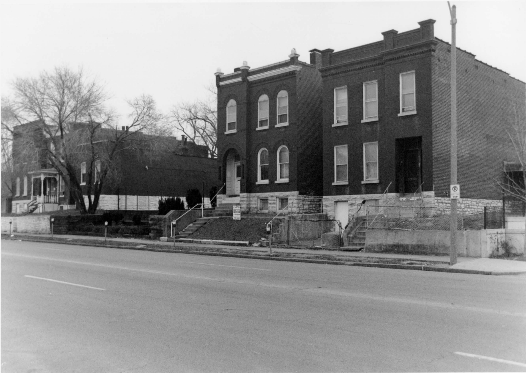
Forest Park Southeast Historic District Boundary Increase St. Louis (Independent City), MO #13
