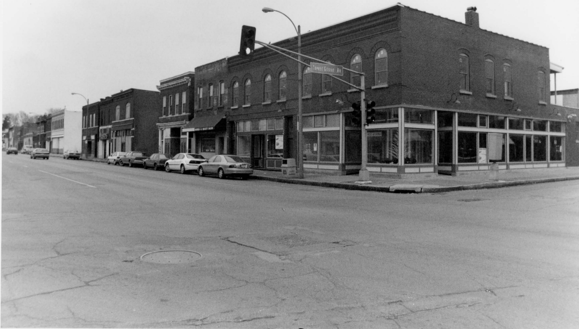
Forest Park Southeast Historic District Boundary Increase St. Louis (Independent City), MO # 11
