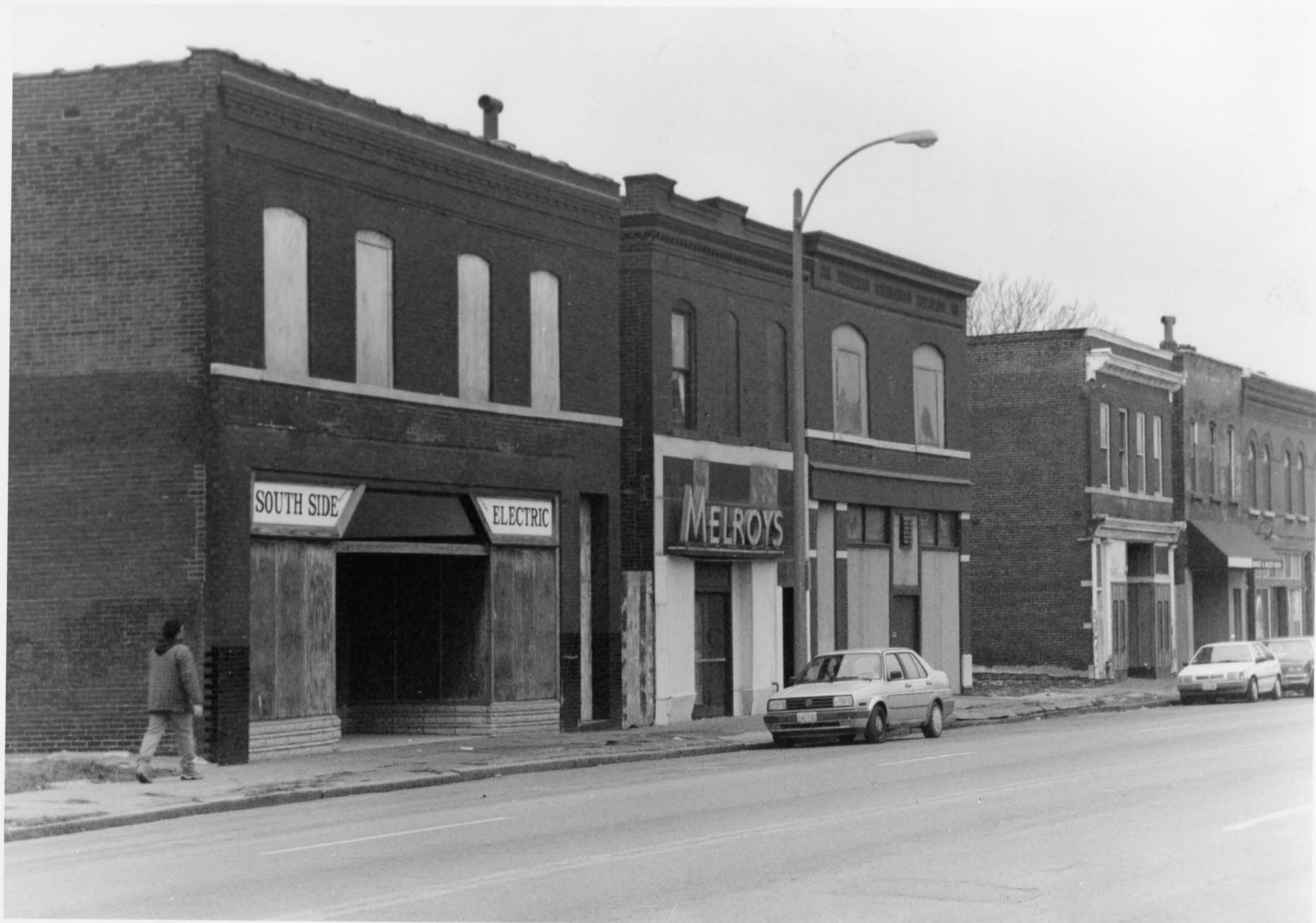
Forest Park Southeast Historic District Boundary Increase St. Louis (Independent City), Mo #10
