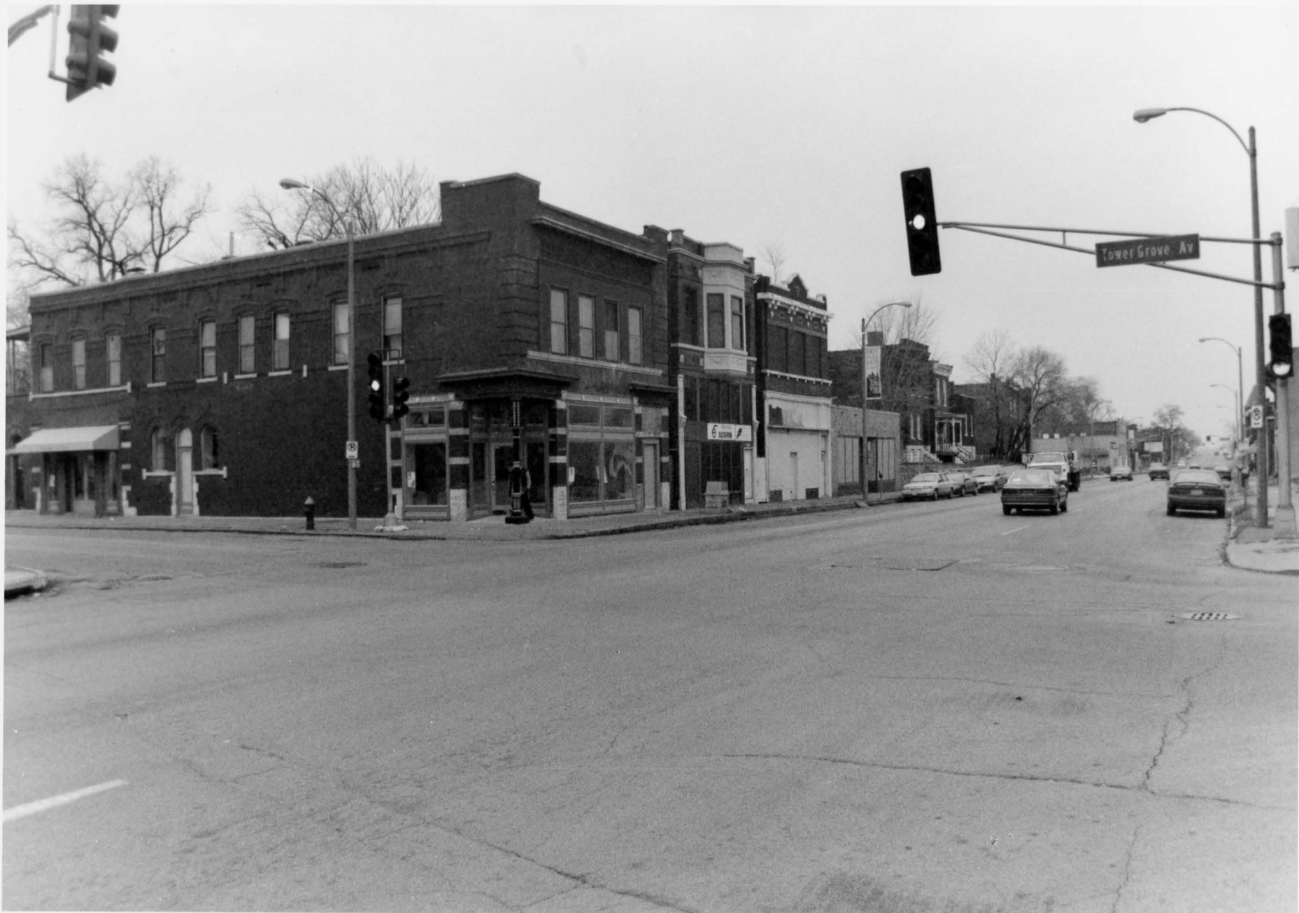
Forest Park Southeast Historic District Boundary Increase St. Louis (Independent City), MO #12
