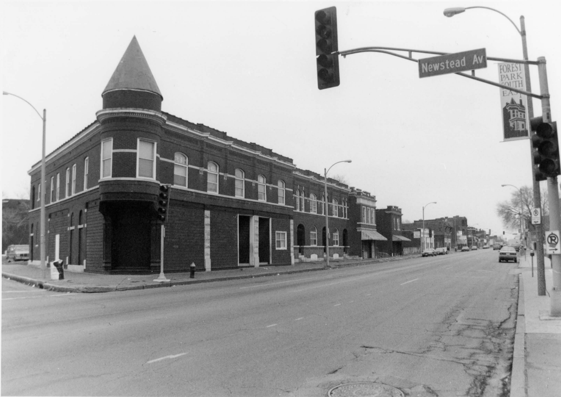
Forest Park Southeast Historic District Boundary Increase St. Louis (Independent City), MO #1
