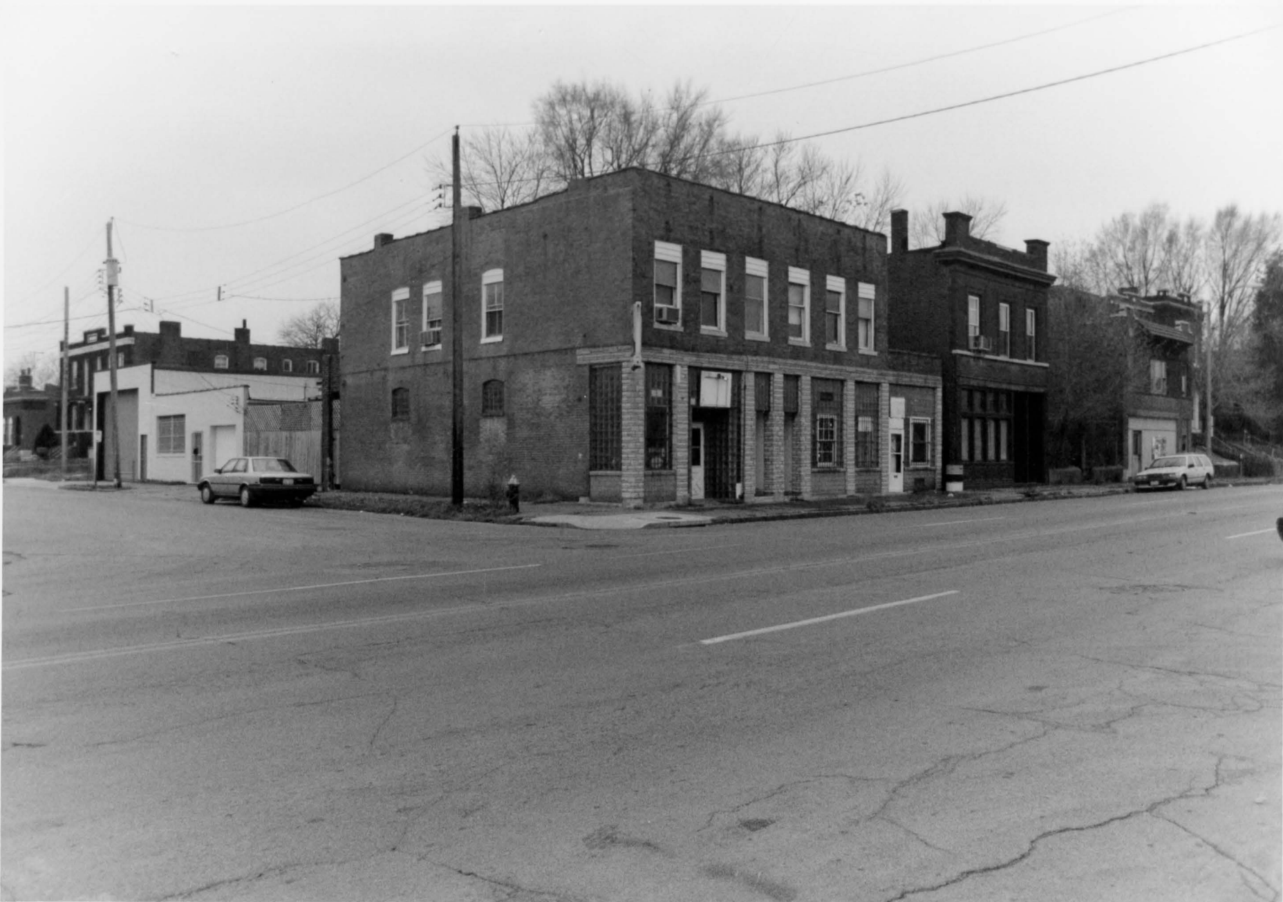
Forest Park Southeast Historic District Boundary Increase St. Louis (Independent City), MO #5
