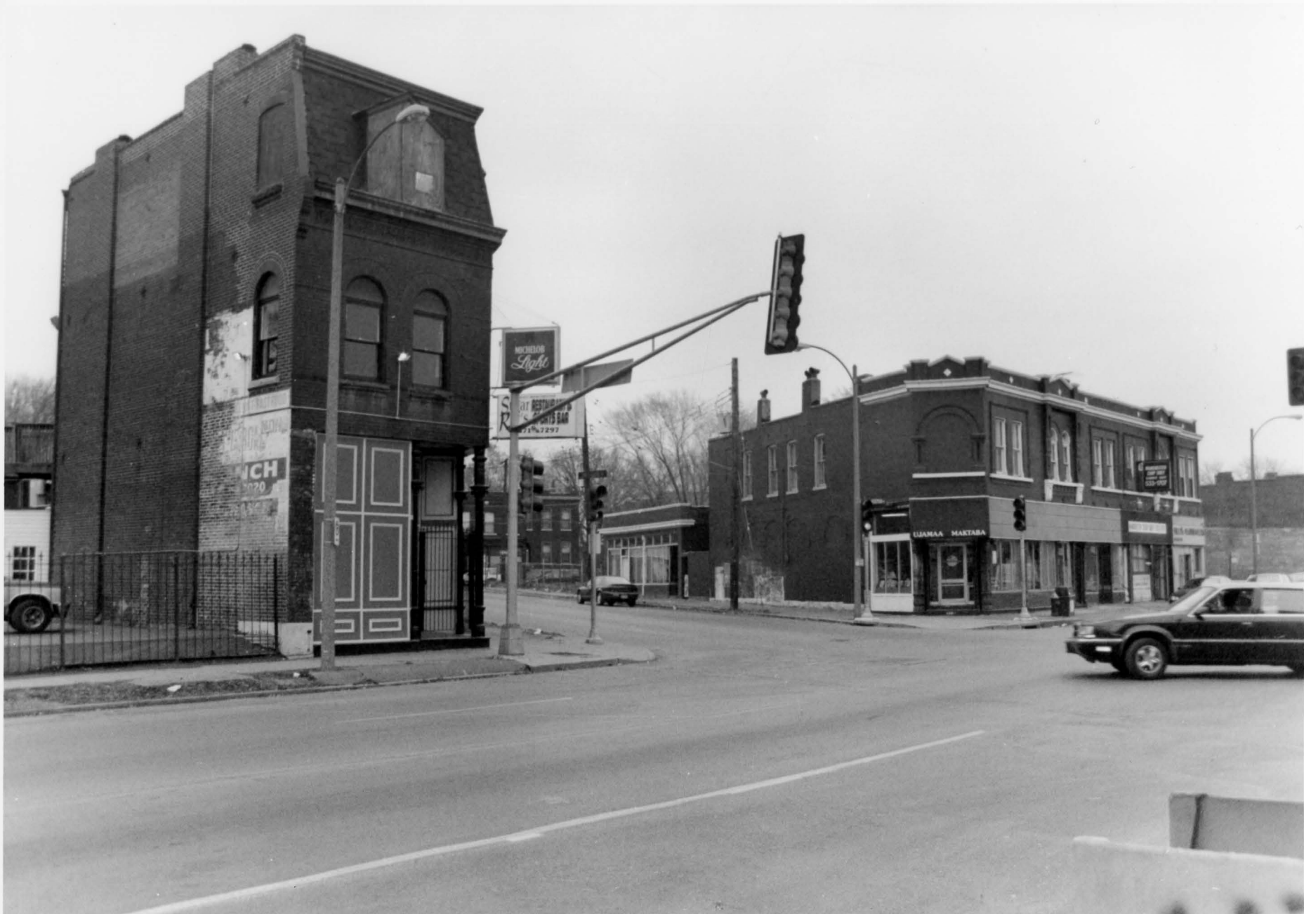
Forest Park Southeast Historic District Boundary Increase St. Louis (Independent City), MO #3
