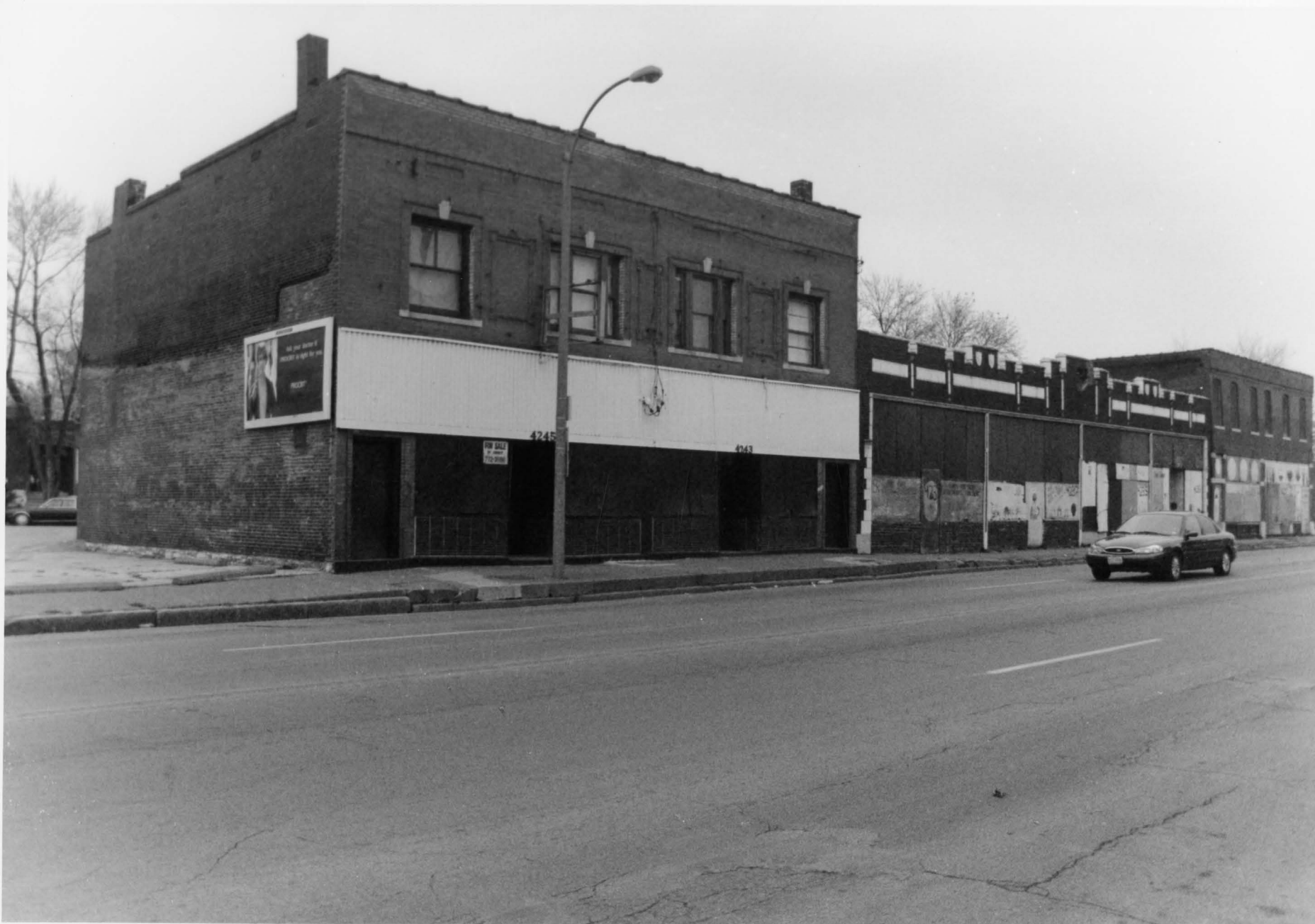
Forest Park Southeast Historic District Boundary Increase St. Louis (Independent City), MO #4
