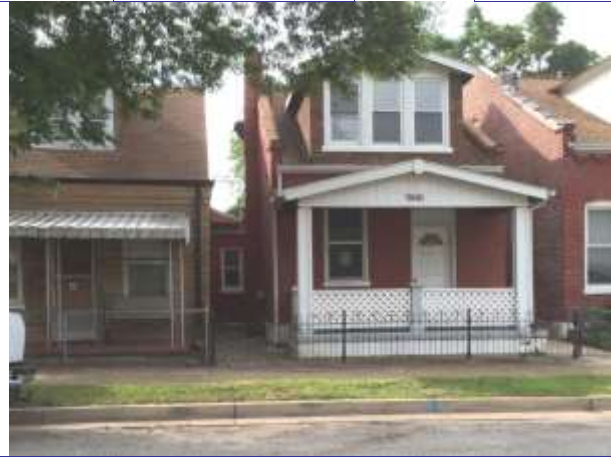
Front: note flounder wall exposed at left
