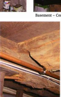
Floor Joists Notched Over Beam
