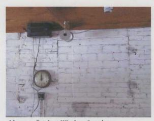
Masonry Patch at Window Opening
