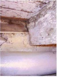
Joist Bearing at Perimeter Sill
