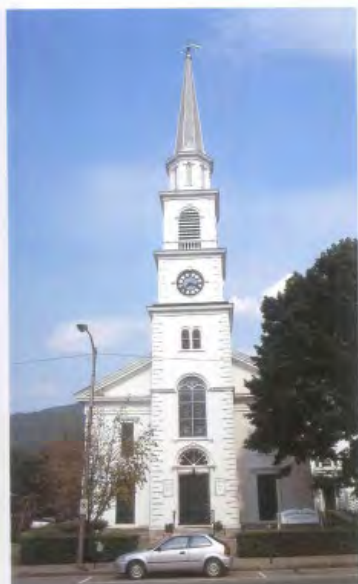
Above: Center Congregational Church, 193 Main Street, Brattleboro, VT, 1843.
