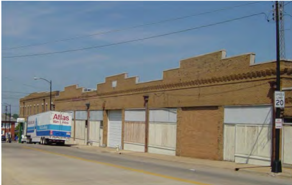
Figure 6. Details of the Front Cornice. (Photos by Deb Sheals 2023.)
