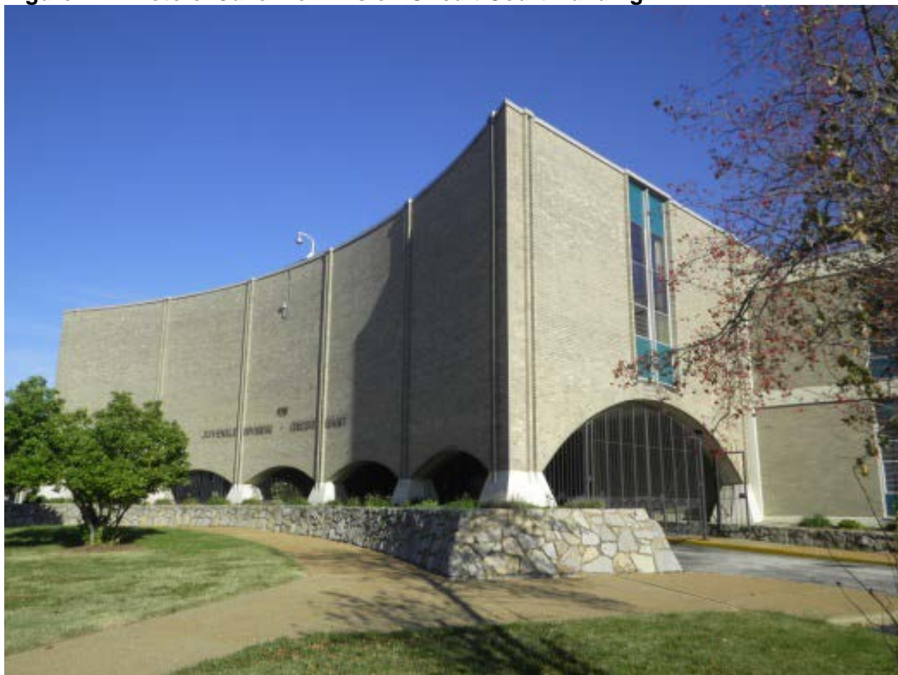
Figure 14: Photo of Juvenile Division Circuit Court Building 63
