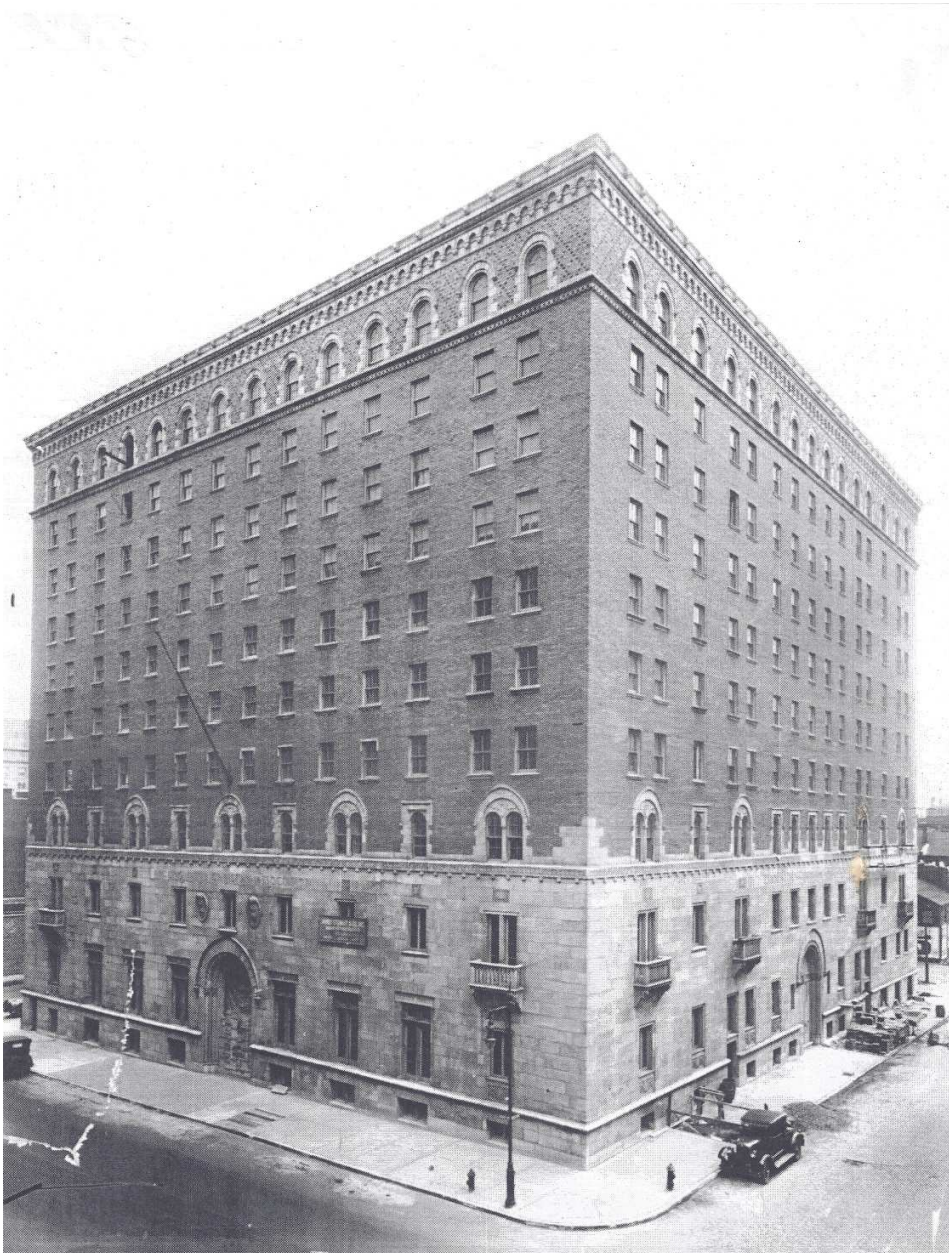
Figure 5: The Downtown YMCA Building under construction, 1926. Source: Collections of the St. Louis Mercantile Library Association.
