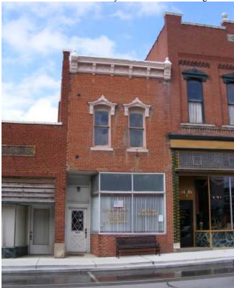
Figure 14. 421 Main Street (LN-AS-001-018) is an example of an Italianate commercial style building.
