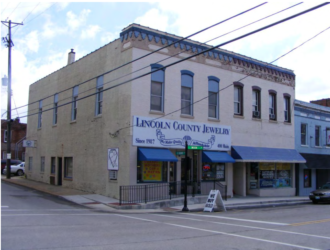
Figure 17. 400 – 430 Main Street appears as a single building initially but a closer look clearly demonstrates two separate businesses/buildings.
