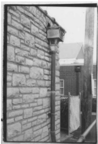
Stone addition with copper guttering, #9
