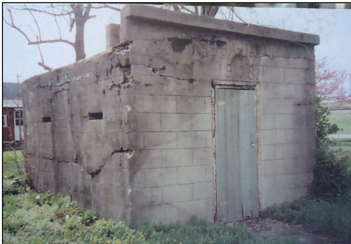
Figure 6: Historical Society photograph of building, circa 1970s. Note the condition and the exterior-most metal door (not original).
