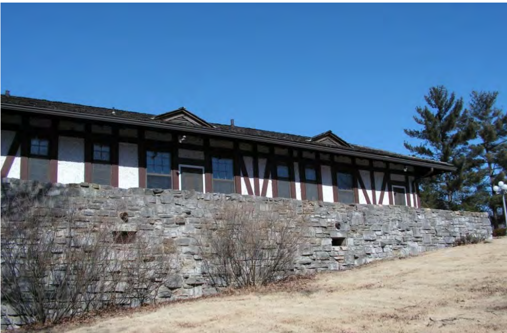
Figure 7: Current comparison photo of roof.
