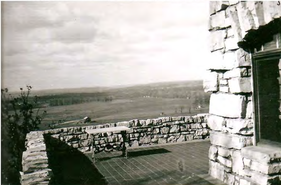
Figure 4 Circa 1935 Southwest corner of terrace
