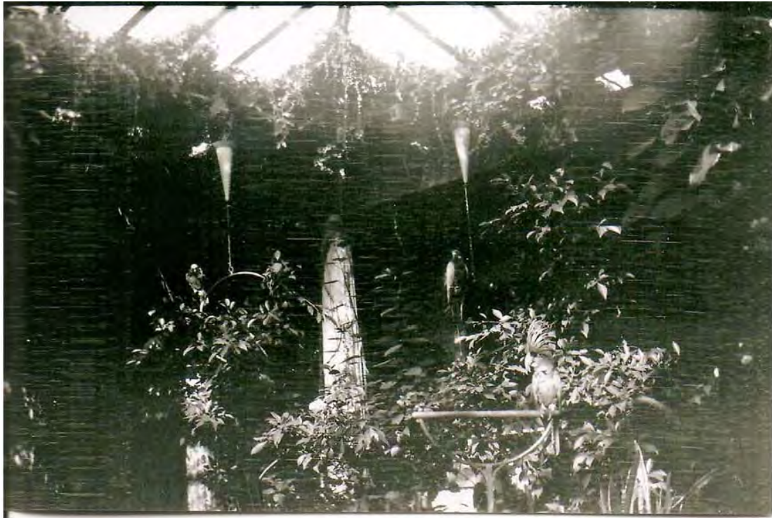
Figure 8 Circa 1935 Atrium with glass roof
