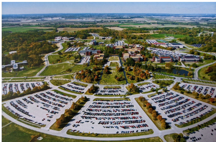
Figure 20: Southern Illinois University Edwardsville. Master plan and original buildings. Marlene Ann Birkman, "Gyo Obata, Architect, Clients, Reflections", (Victoria, Australia; Images Publishing, 2010), pages 13.
