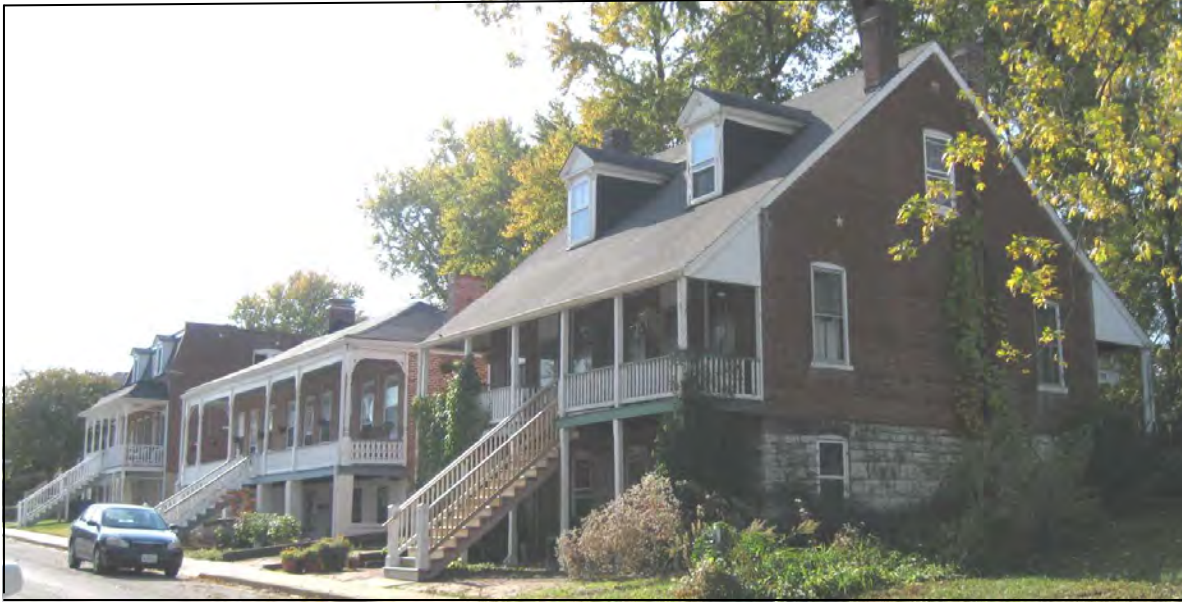
FIGURE NO. 9: 1017-1001 North Third Street in the Frenchtown Historic District.
