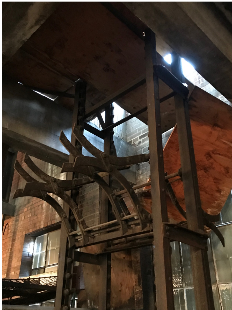
Figure 8: Oil barrel elevator at the first floor. Source: Preservation Research Office photograph, 2018.
