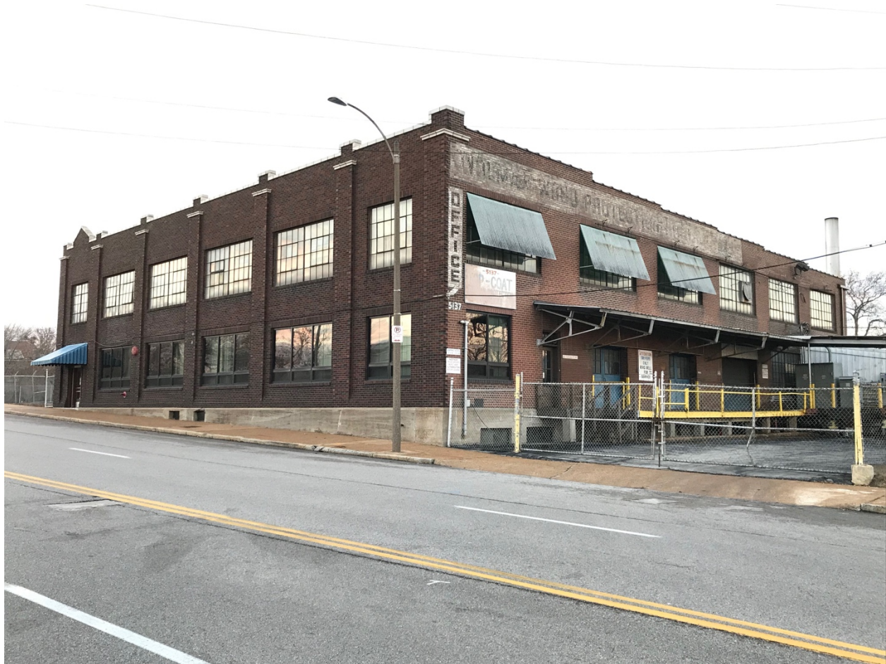
Figure 12: National Refining Company Warehouse at 5137 Southwest Avenue in St. Louis. Source: Photograph by the preparer, December 2018.
