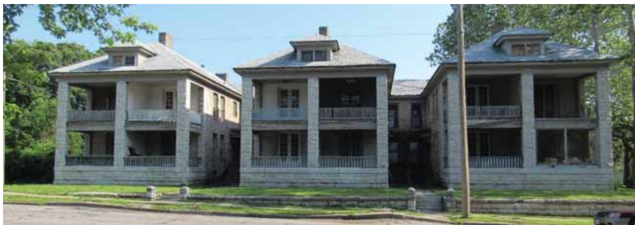
Figure 17. Front (south) facade of Cleveland Apartments 2021. (Emrie)
