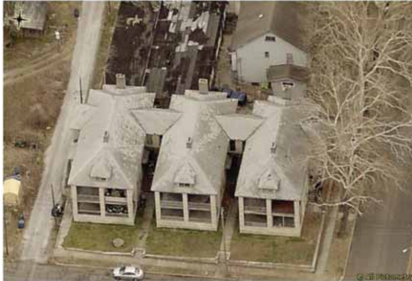
Figure 5. Beacon photo of Cleveland Apartments. Mar 4, 2020. (courtesy Neal Construction)
