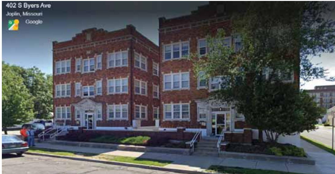
27. Ridgeway Apartments at 402-402 South Byers Avenue, Joplin, MO. (Google Earth 8/16/2021)
