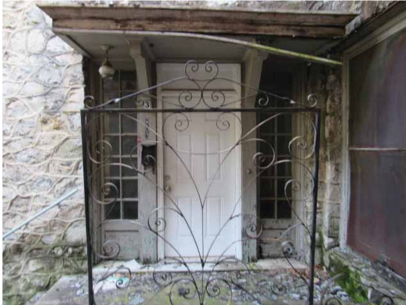
Figure 11. Entry door with sidelights. Original door replaced with modern door and transom light removed. (Emrie)
