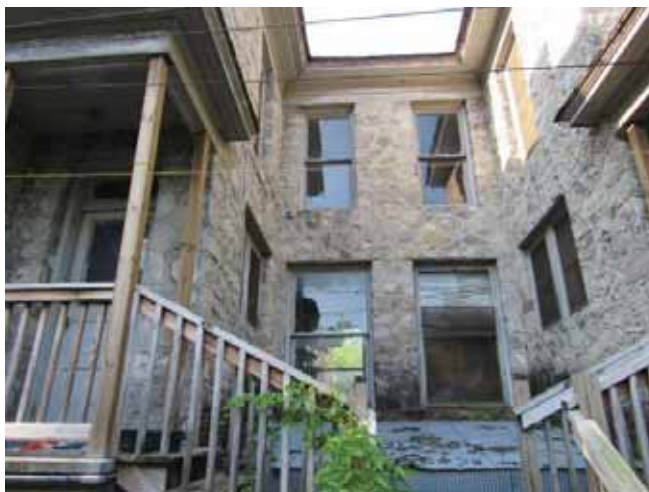
Figure 10. One over one wood frame double hung window. Carthage stone masonry. (Emrie)
