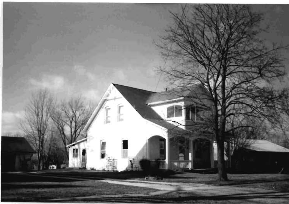
North Jefferson Typical 1½ story brick structure with 6/6 square windows, segmentally arched headers
