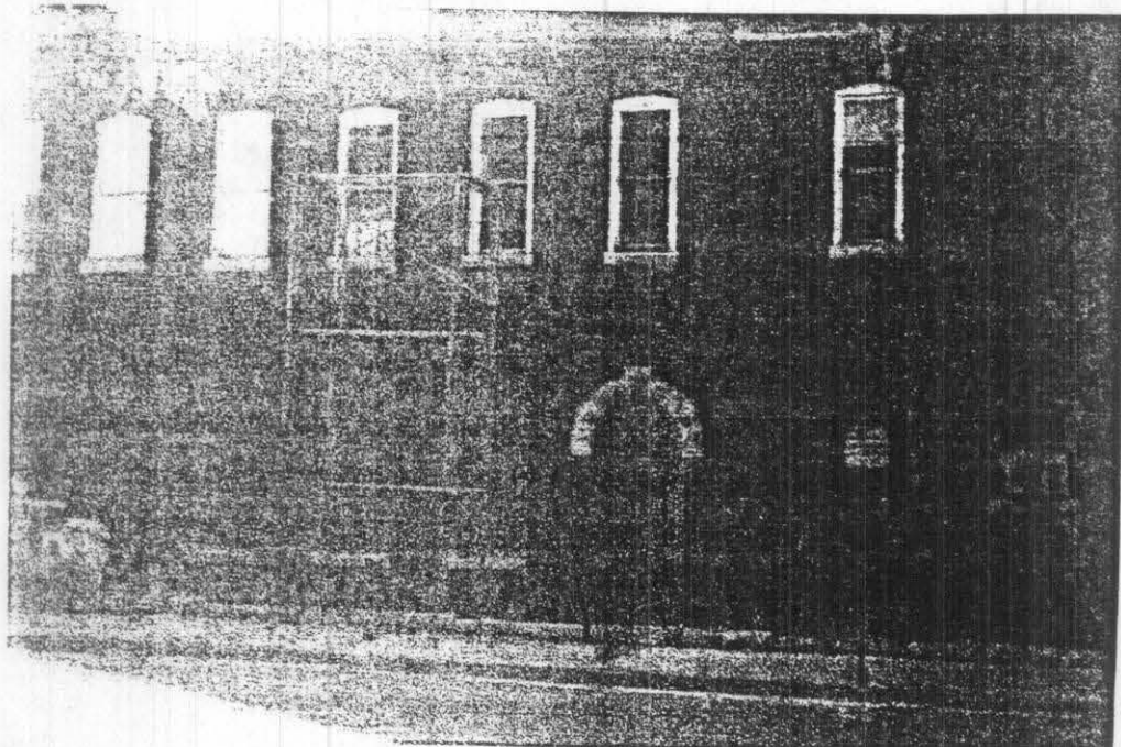
Facing north, south elevation
