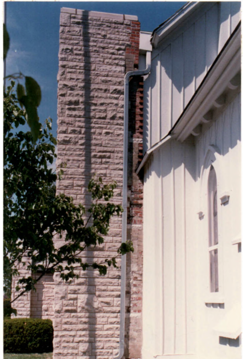
14. Joining of 1870 nave and 1927 transept. Note truncated remains of original Side Porch.
