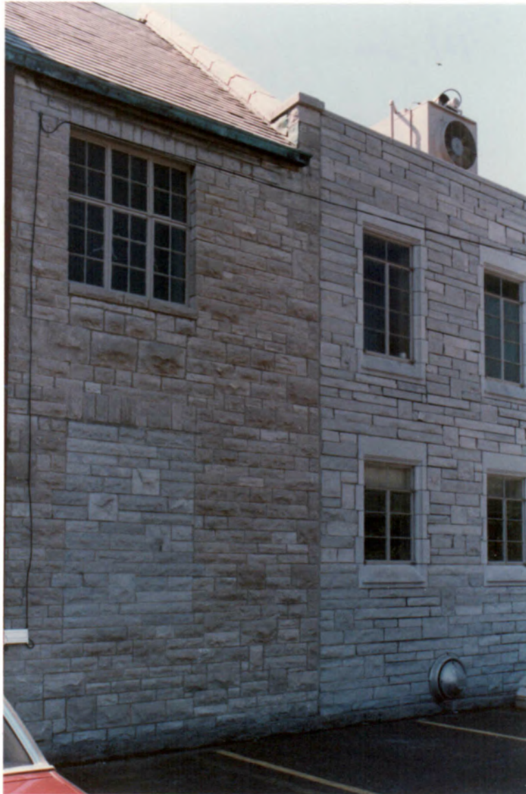
15. Joining of 1927 office/education wing with 1958 Parish Hall (east side, rear).
