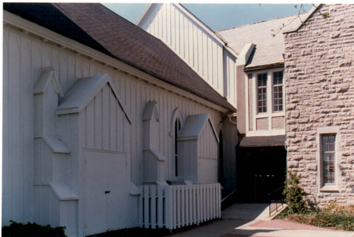
4. View NNW. Utility structures in wall to be removed in current renovation.
