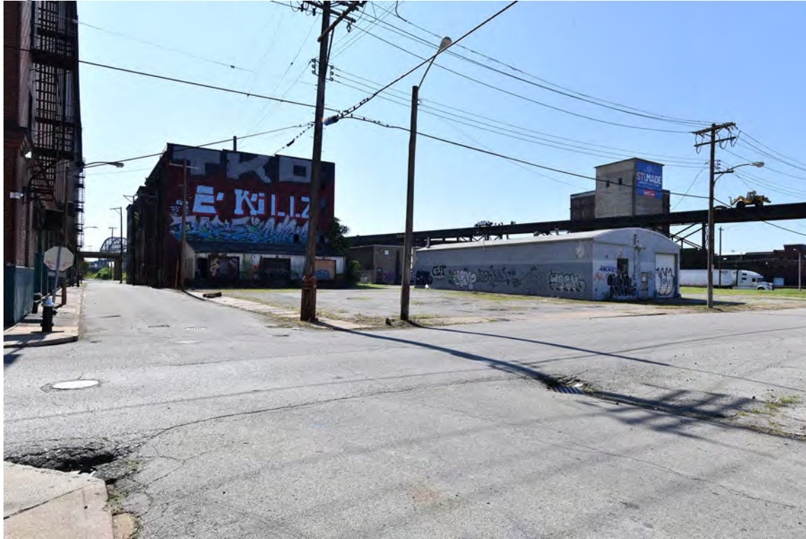
Figure 19. Resources 8 and 12, view SE, Finch, 2023.
