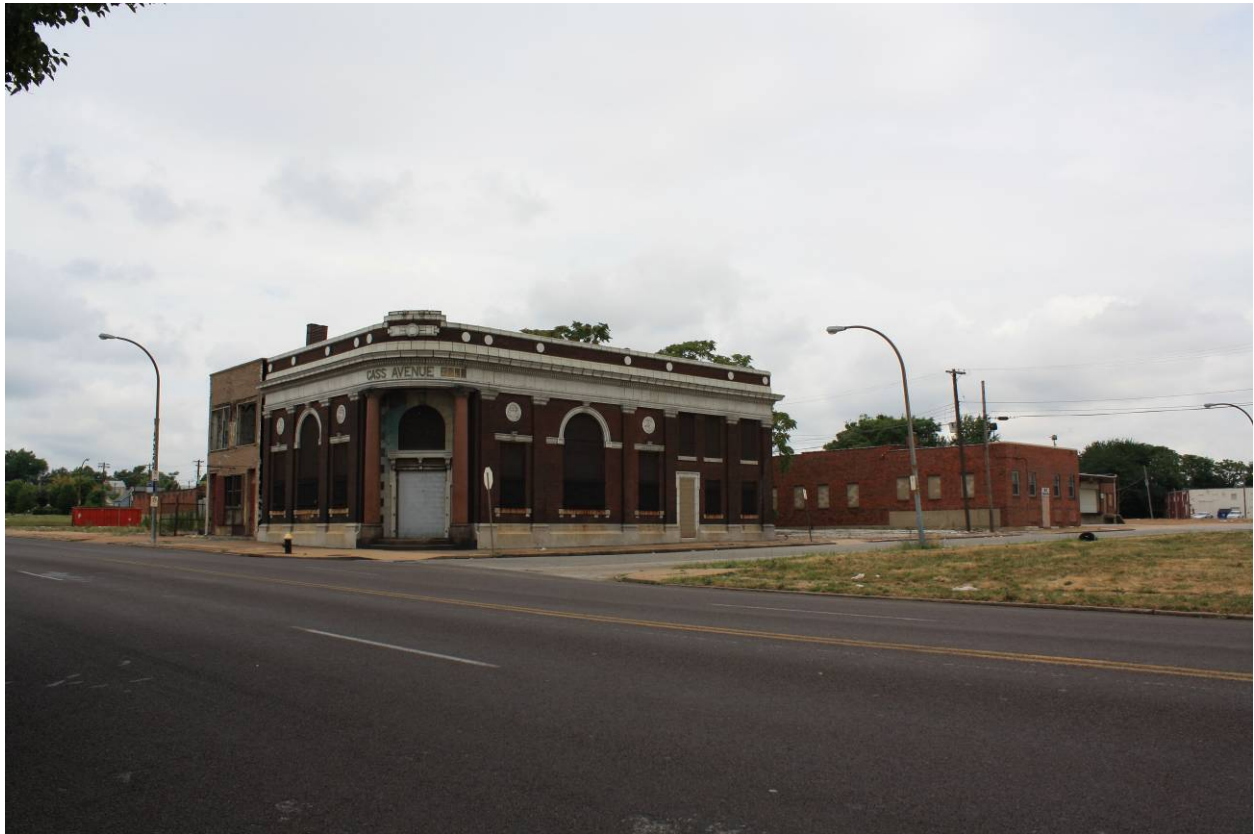
Figure 7: Current Photo of 1501 Cass 2 nd Bank Location
