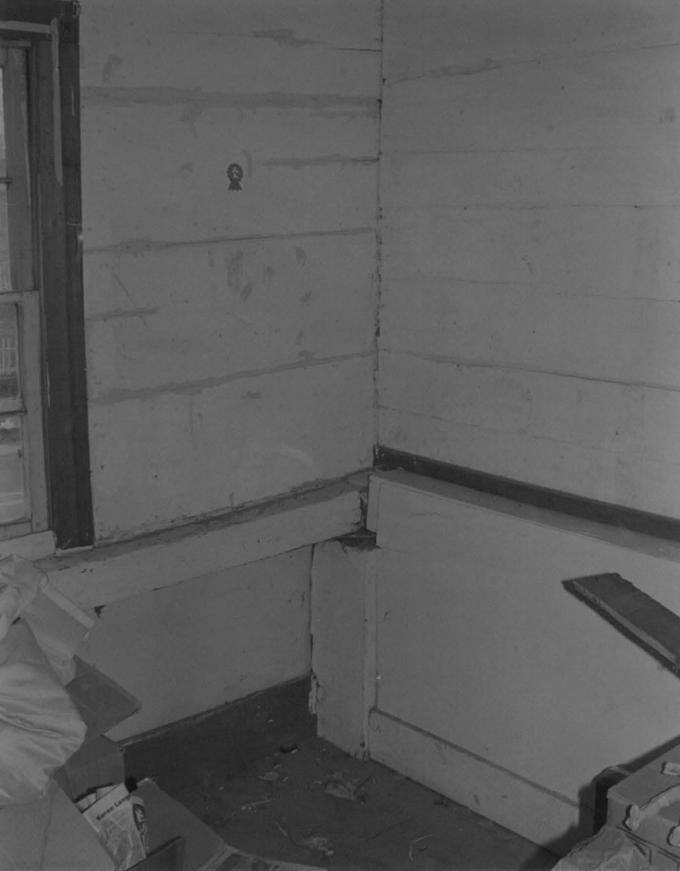
77. Second floor passage, Long-White house, looking NW at corner where blocks A and B are joined. Note post and lintels and plank walls.
