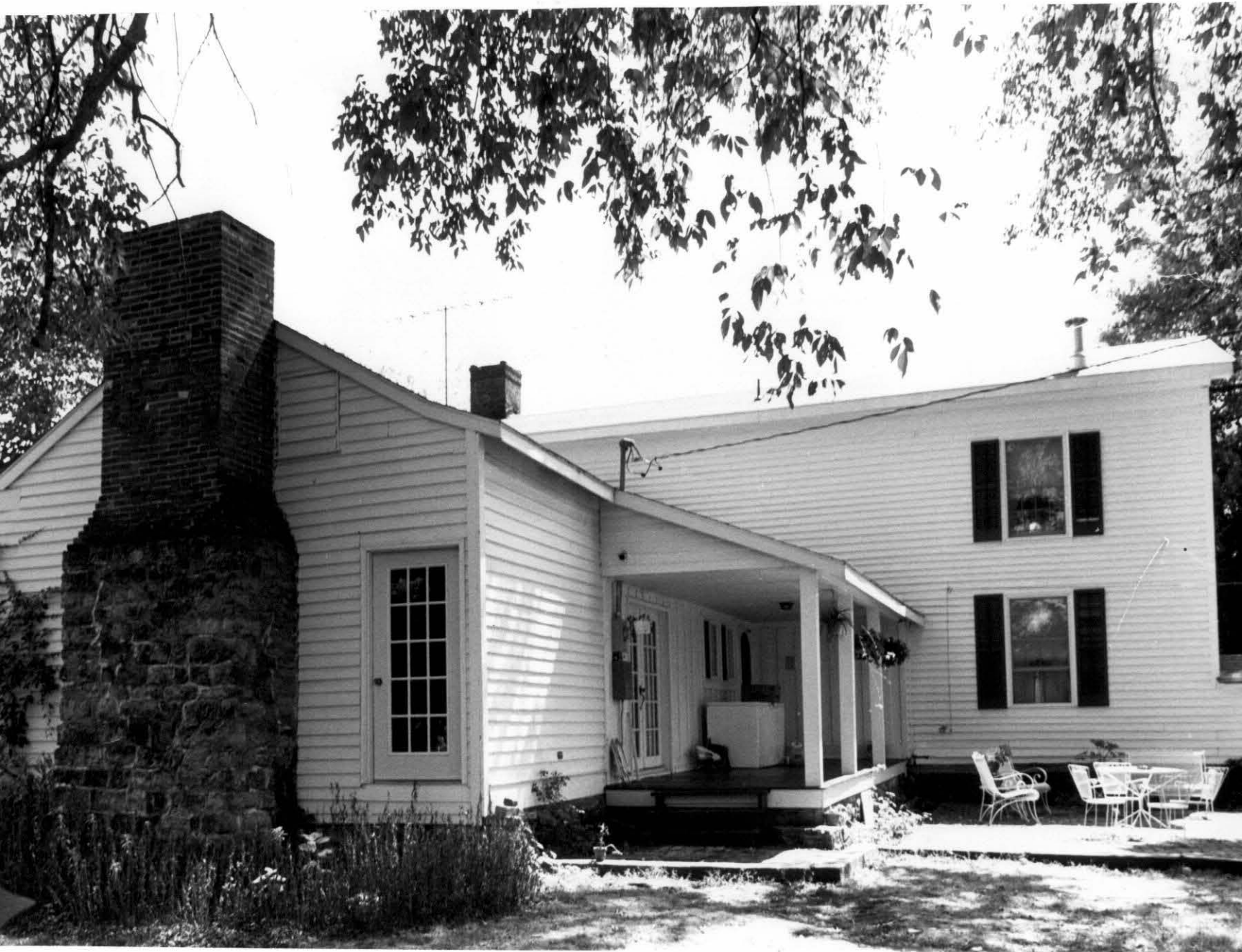
44. Rear ell of Carr-Simms looking ENE. Note stone fireplace and brick chimney.
