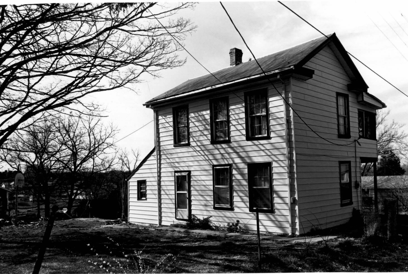
81. Morris house, #22, facade view, looking NW.
