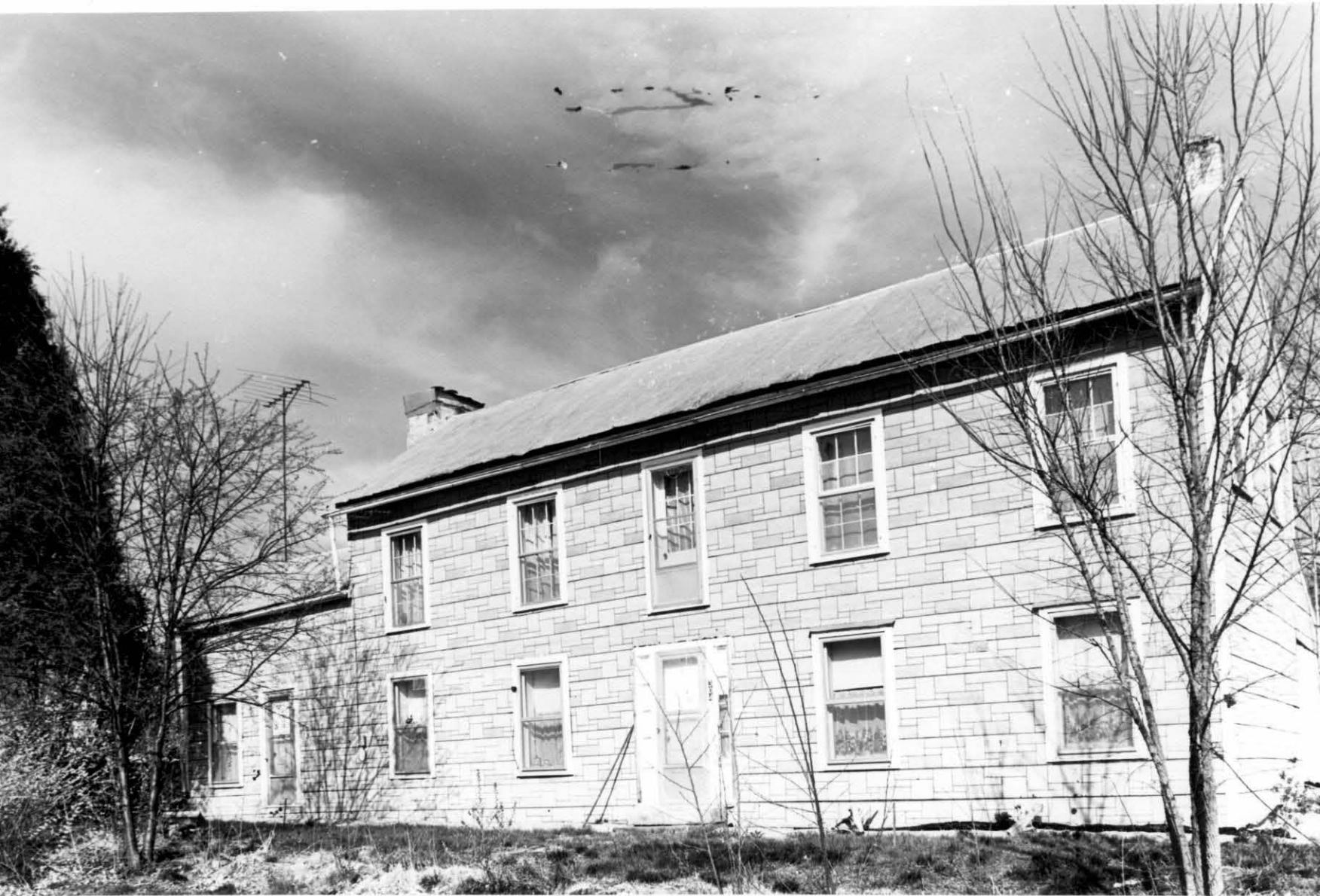
100. Craighead-Henry facade looking NE.
