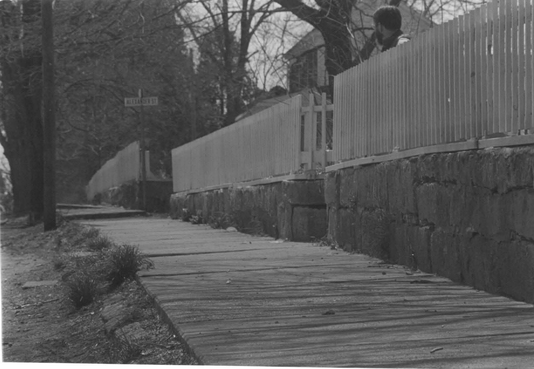
31. Retaining wall, closeup, W. G. Eversole.
