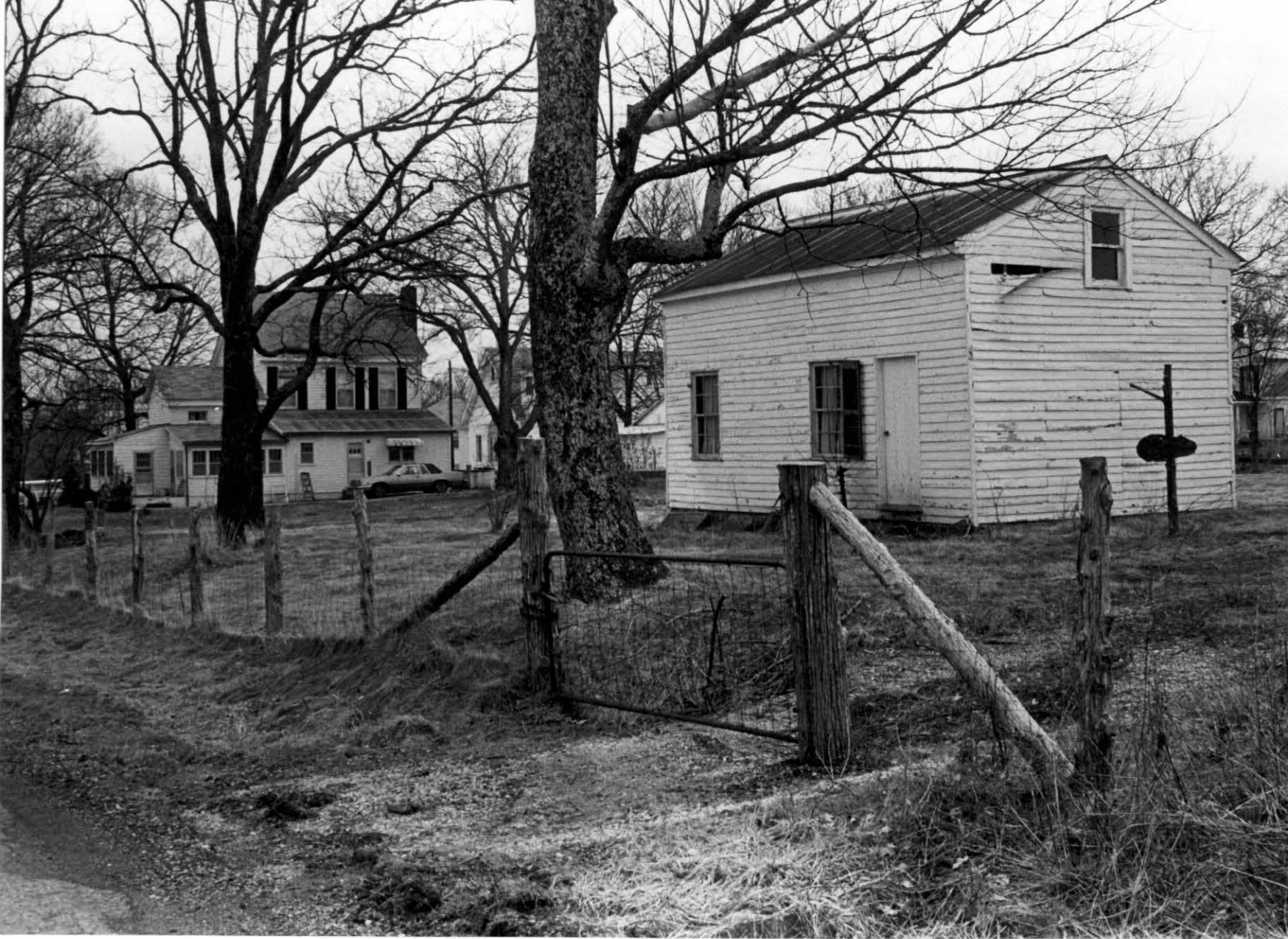
33. Slave house, #6, W. G. Eversole, looking SE. Methodist Church middle background, George Eversole house extreme right.
