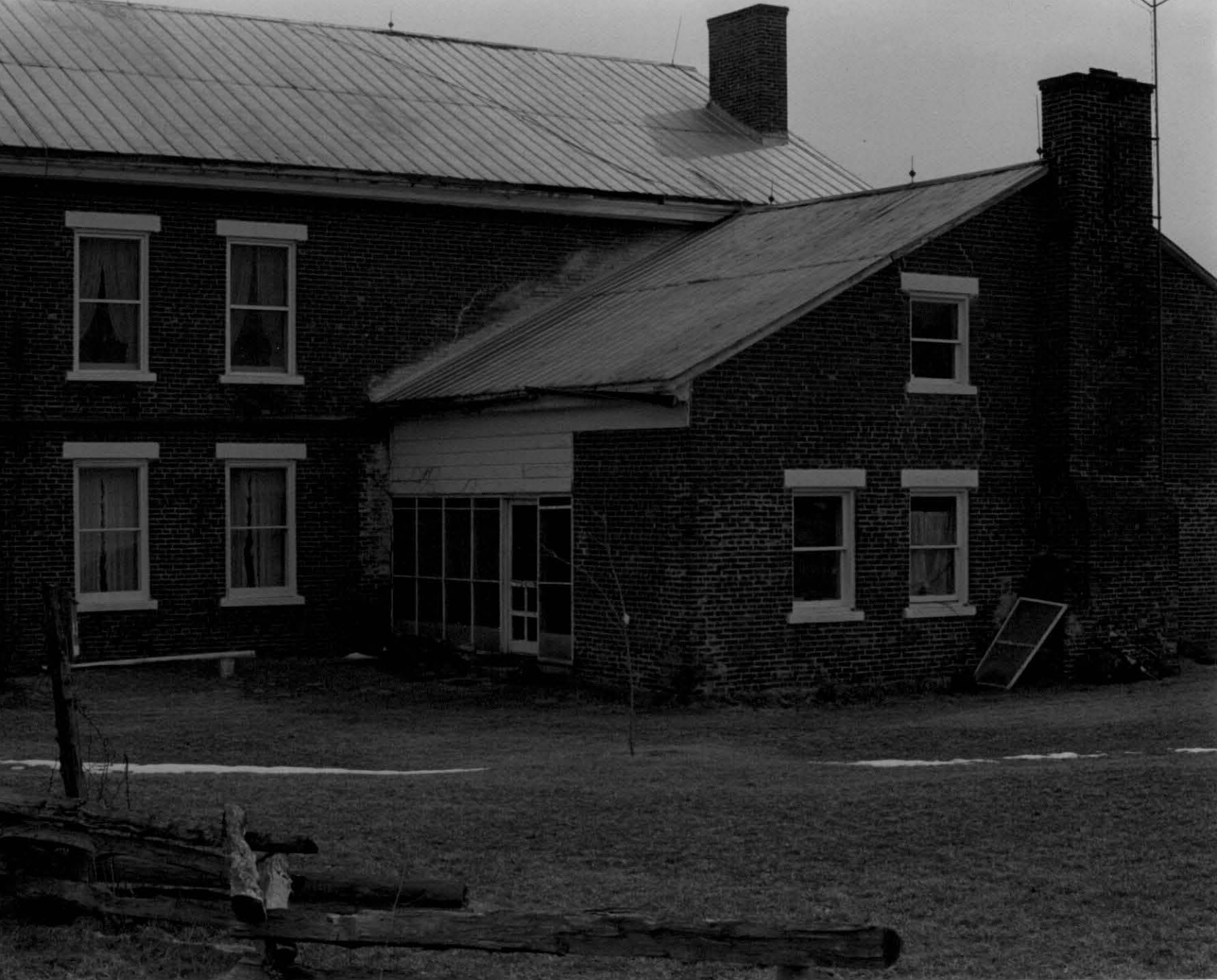
5. Ruggles ell, looking SE. Note upper porch wall of plank. Cool room with window at near ell corner.
