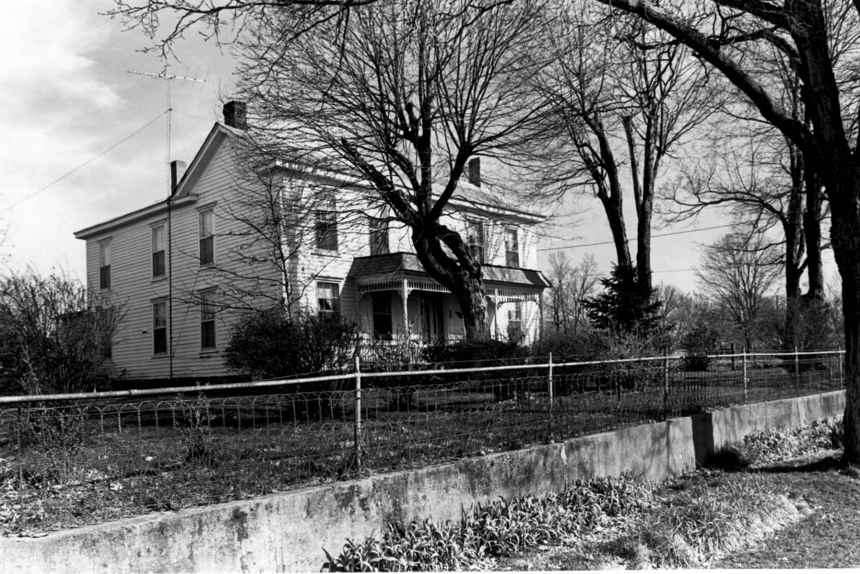
94. Bean house looking SE.
