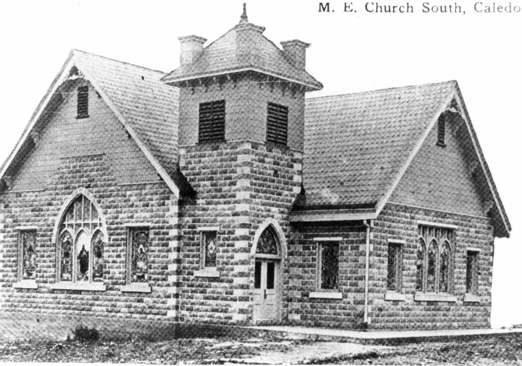
65. New Methodist Church as it appeared when constructed in 1910. Looking SE.
