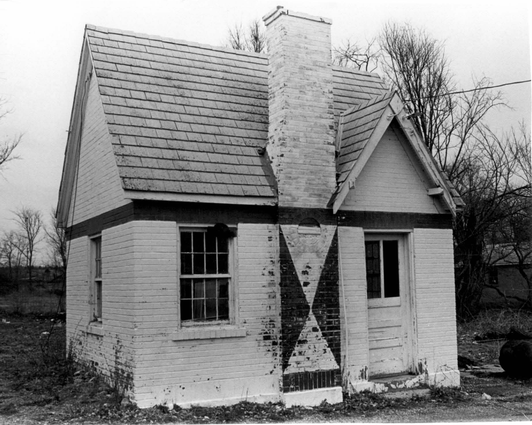
19. Conoco service station, #4, looking WNW.
