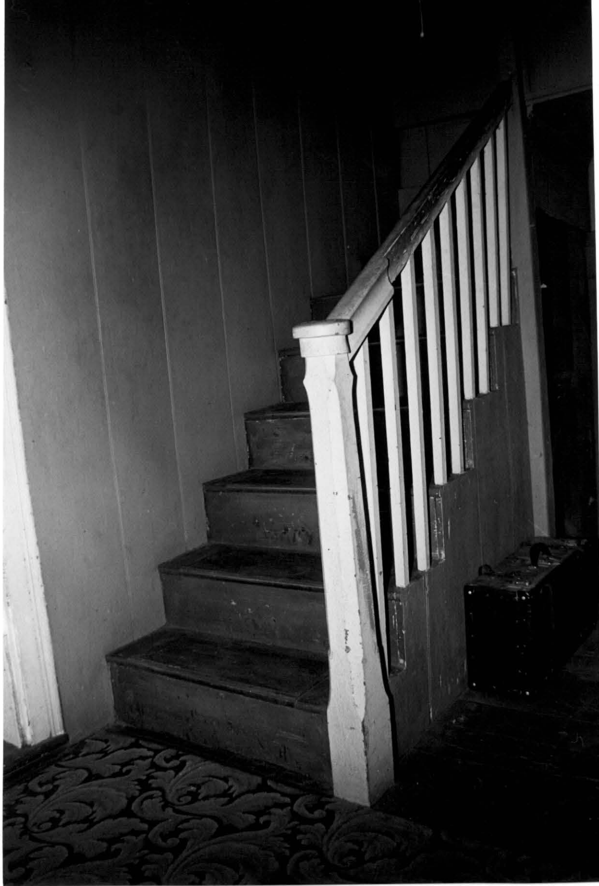
103. Staircase of central passage, Craighead-Henry, lookint ENE.
