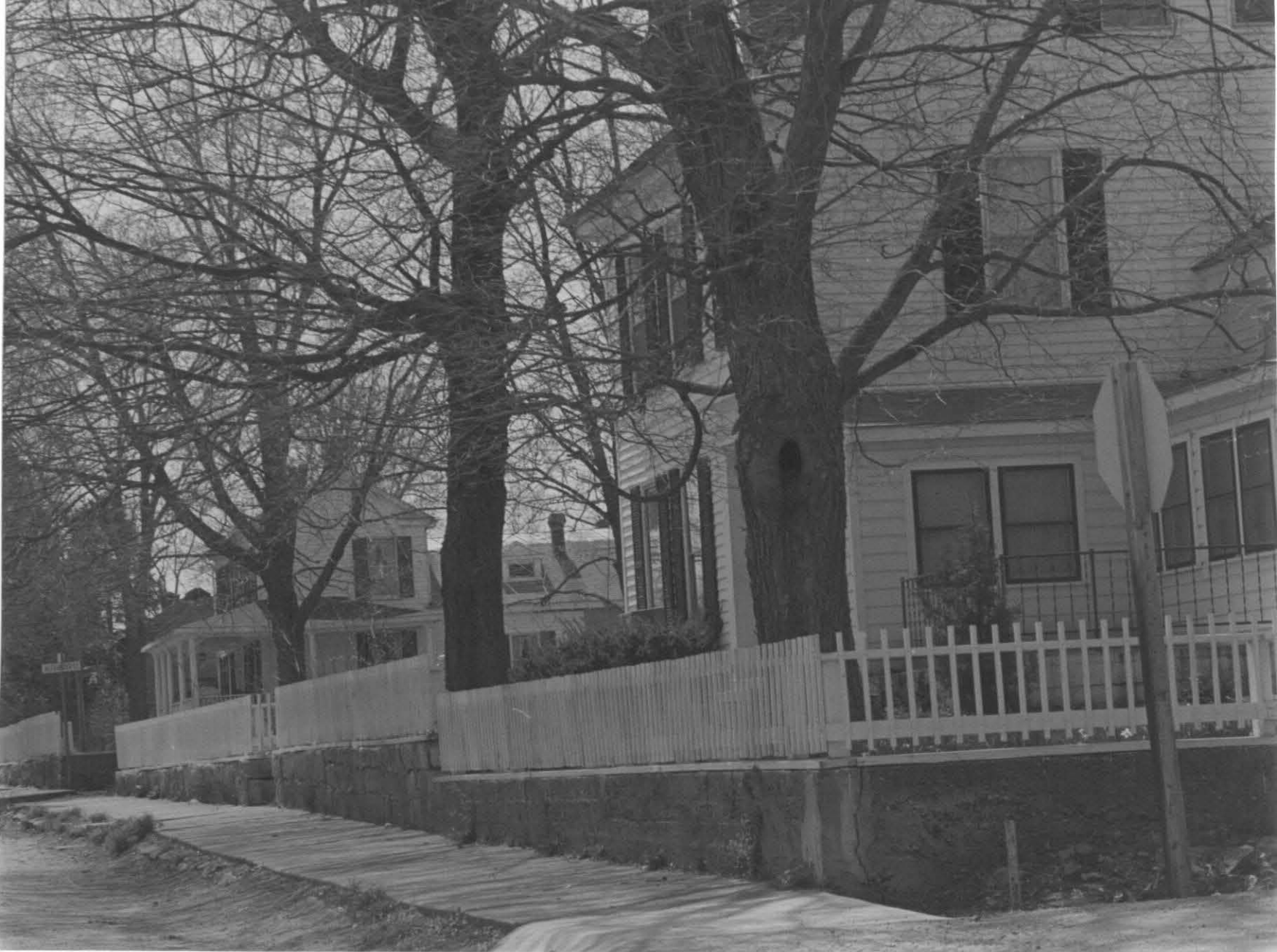
30. Retaining wall, W. G. Eversole, corner Main Street and Webster Road
