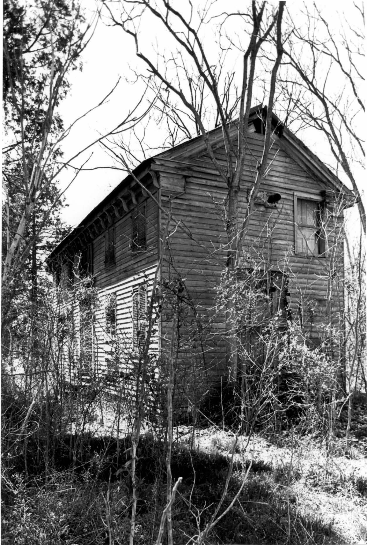
39. Ferson Carr house looking SSW. Note original wall piercing for disappeared chimney. Original upper end wall window replaced by door.
