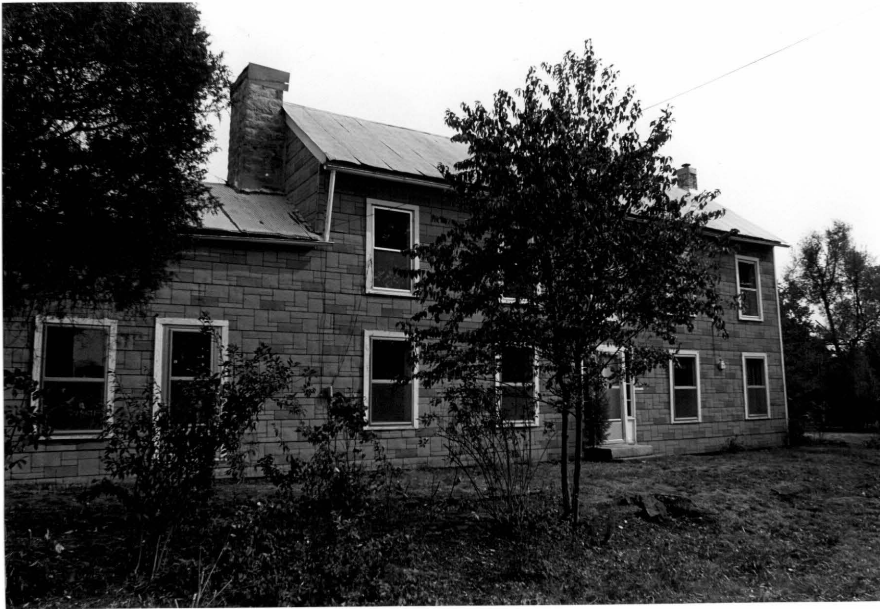
97. Craighead-Henry facade looking E.
