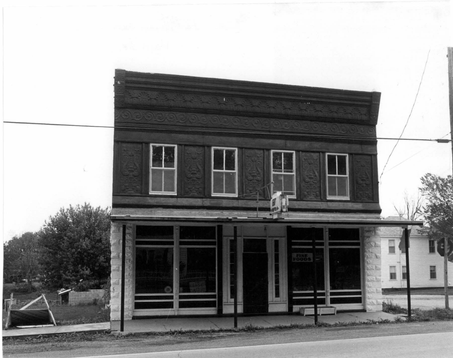
61. Facade, #18, looking ESE. Methodist parsonage right background.
