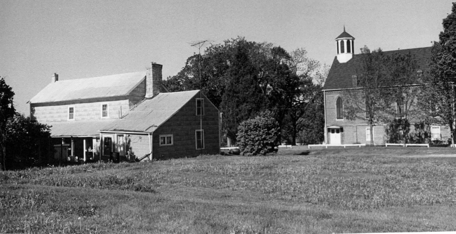
96. View across lot 13 looking SW. Craighead-Henry, #28, at left, Presbyterian Church, #23, at right.
