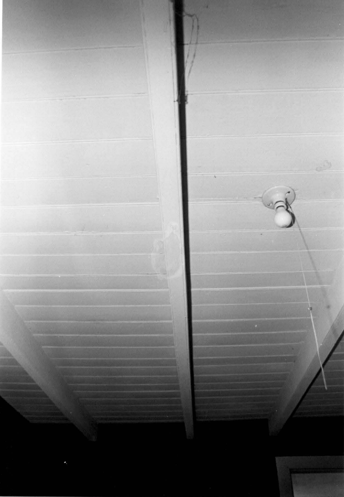
102. Craighead-Henry, ceiling of north first floor log pen looking S, showing beaded plank ceiling and joists.
