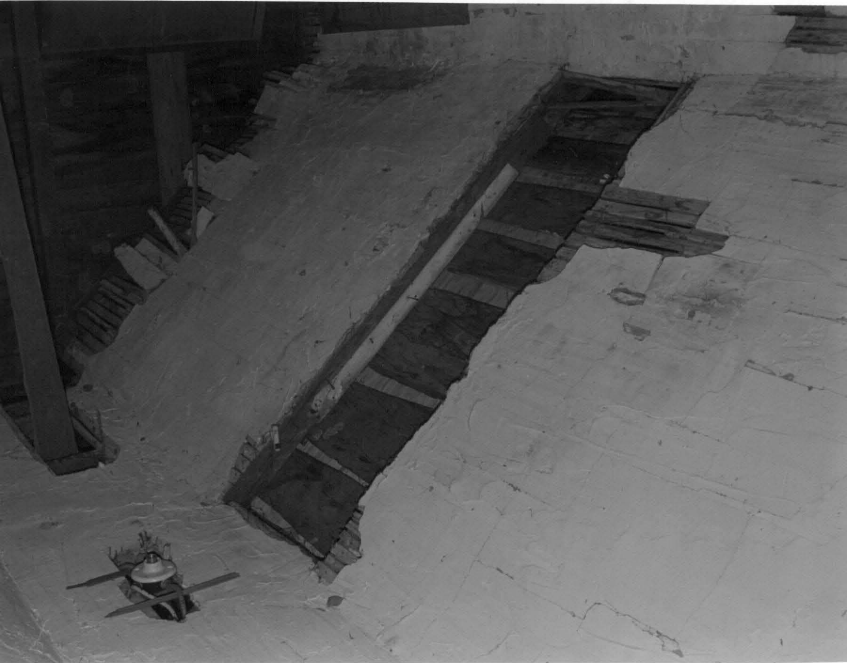
75. Opening in attic ceiling for dormer, block A, Long White house, looking NW.
