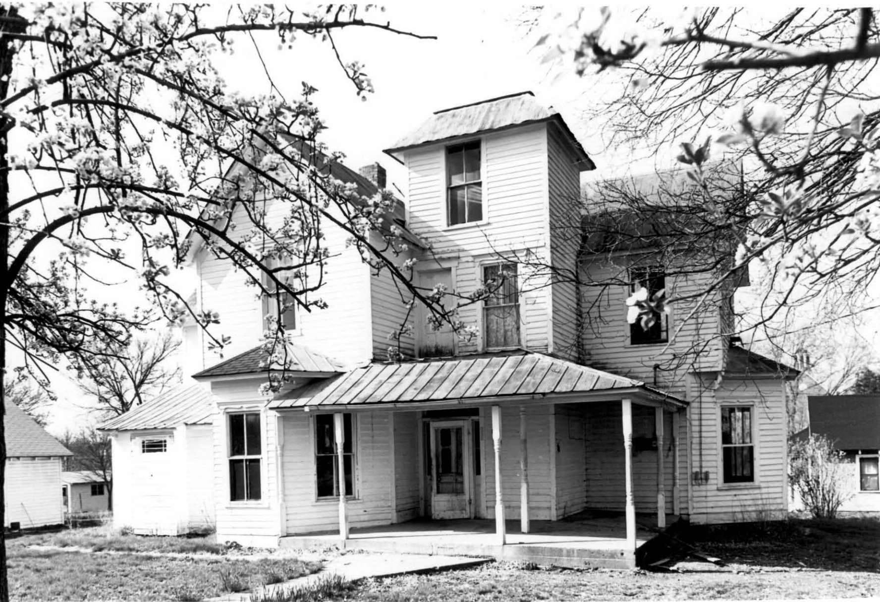
89. Vandiver house, #25, looking NNW. Non-contributing structure #5 at right. Presbyterian Church, right background.
