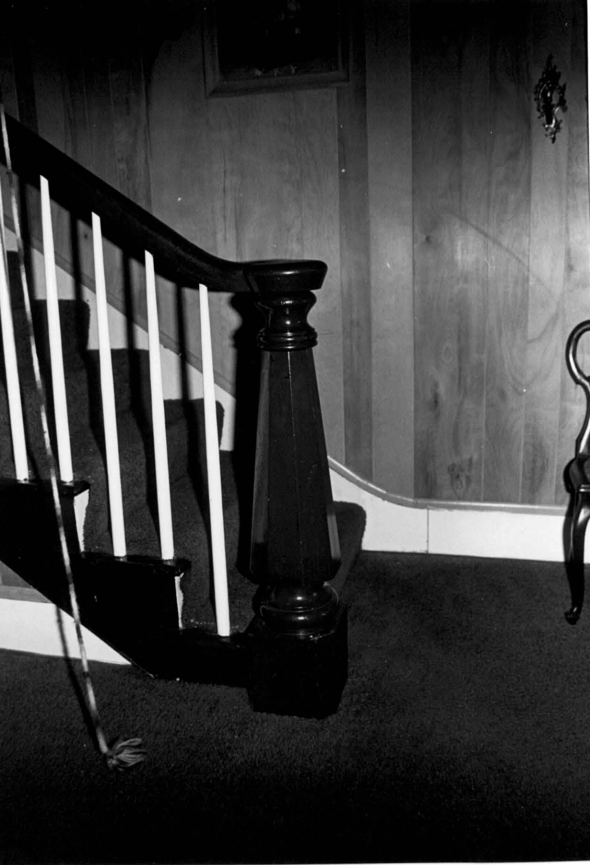
28. Newel post and hand-turned spindles, W. G. Eversole.
