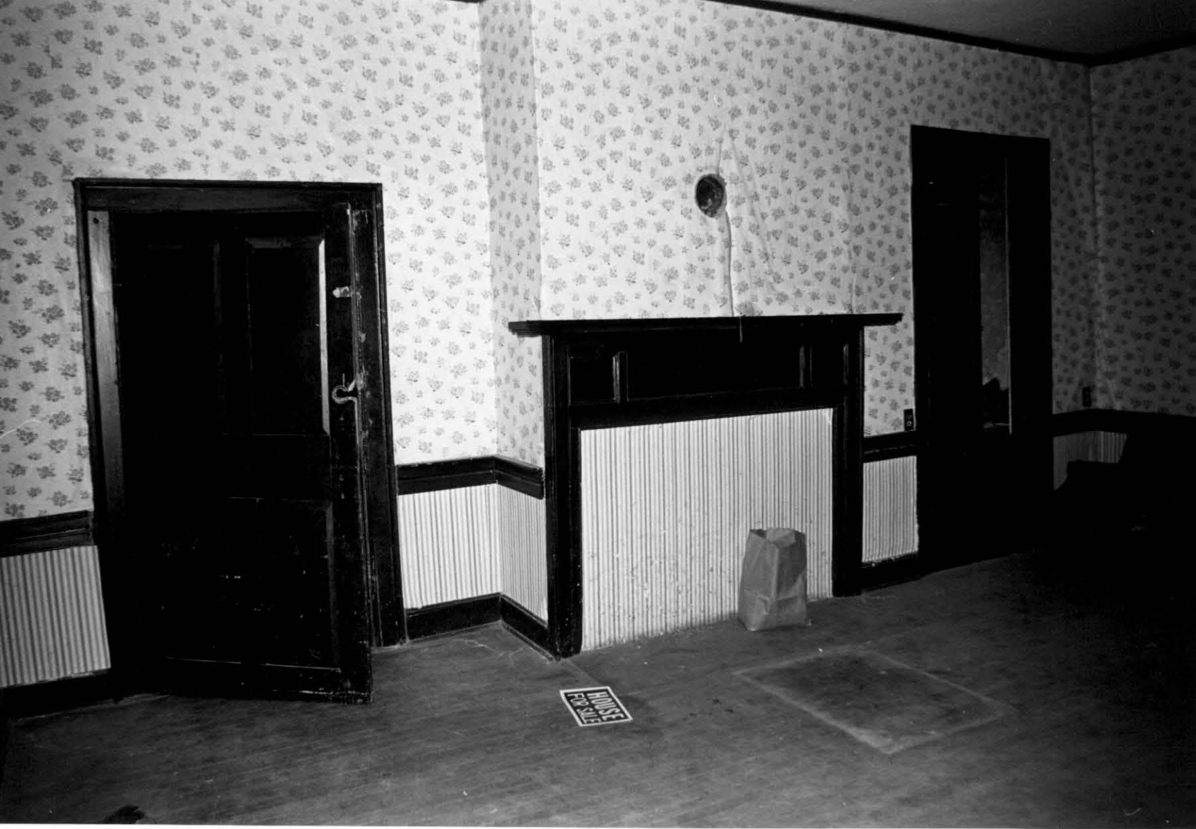
78. Door, mantel, and cupboard, block A, first floor, Long-White house, looking SW.
