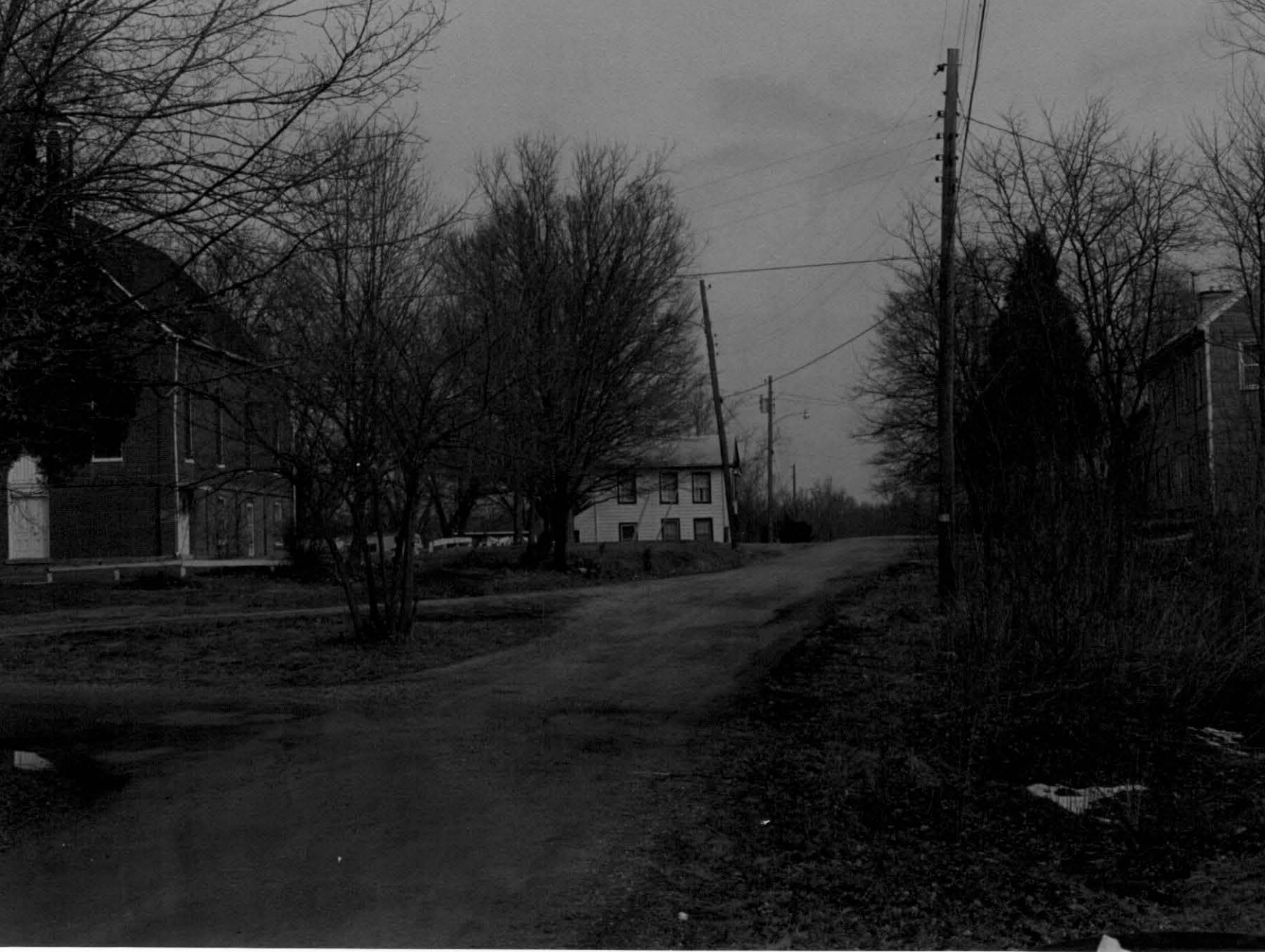
80. College Street looking north past intersection of Henry Street. Presbyterian Church, #23, at left. Morris house, #22, at center, Craighead-Henry, #28, at right.
