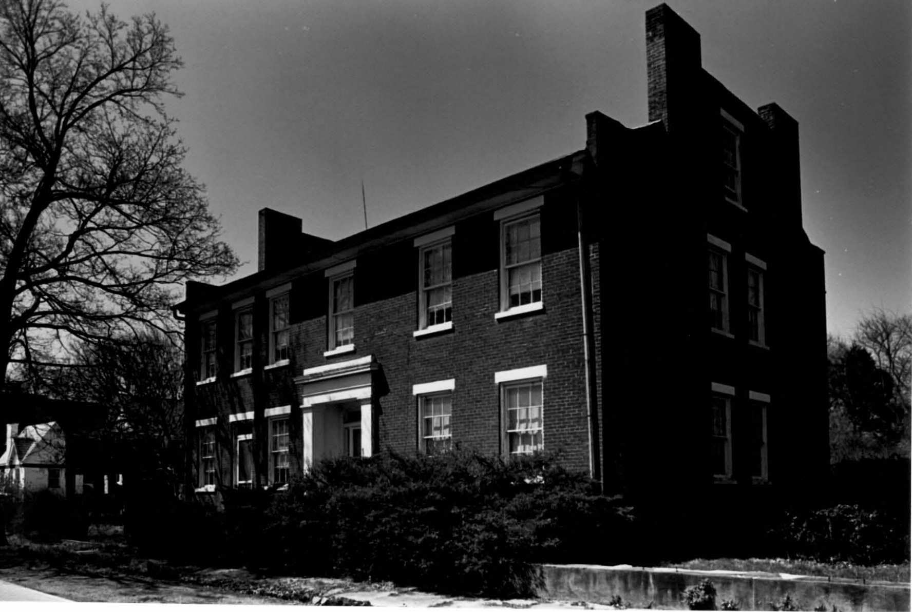
14. Jane Thompson house looking SW. Conoco station left background (intervening house razed in 1982).
