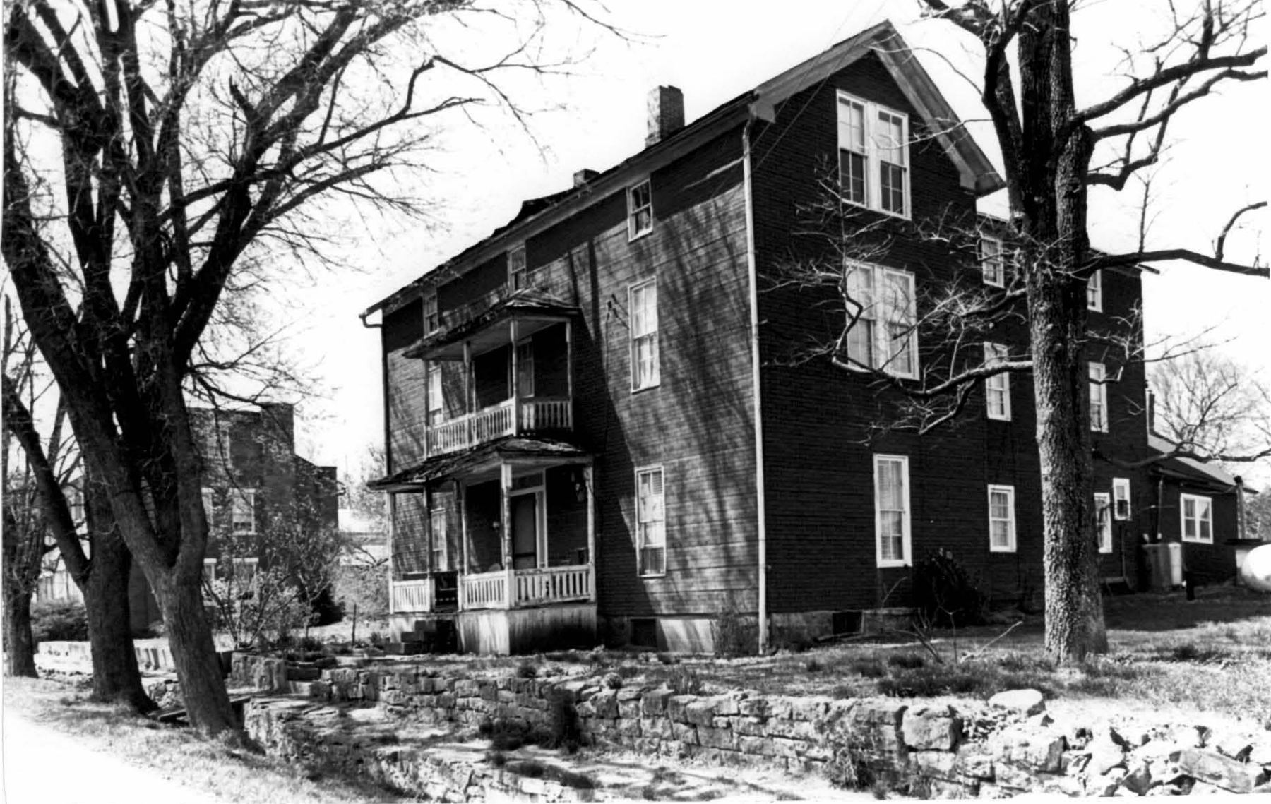
11. Ramsey house, #2, looking SW. Jane Thompson house in background. Note line of trees, lower retaining wall, sidewalk, and upper retaining wall.
