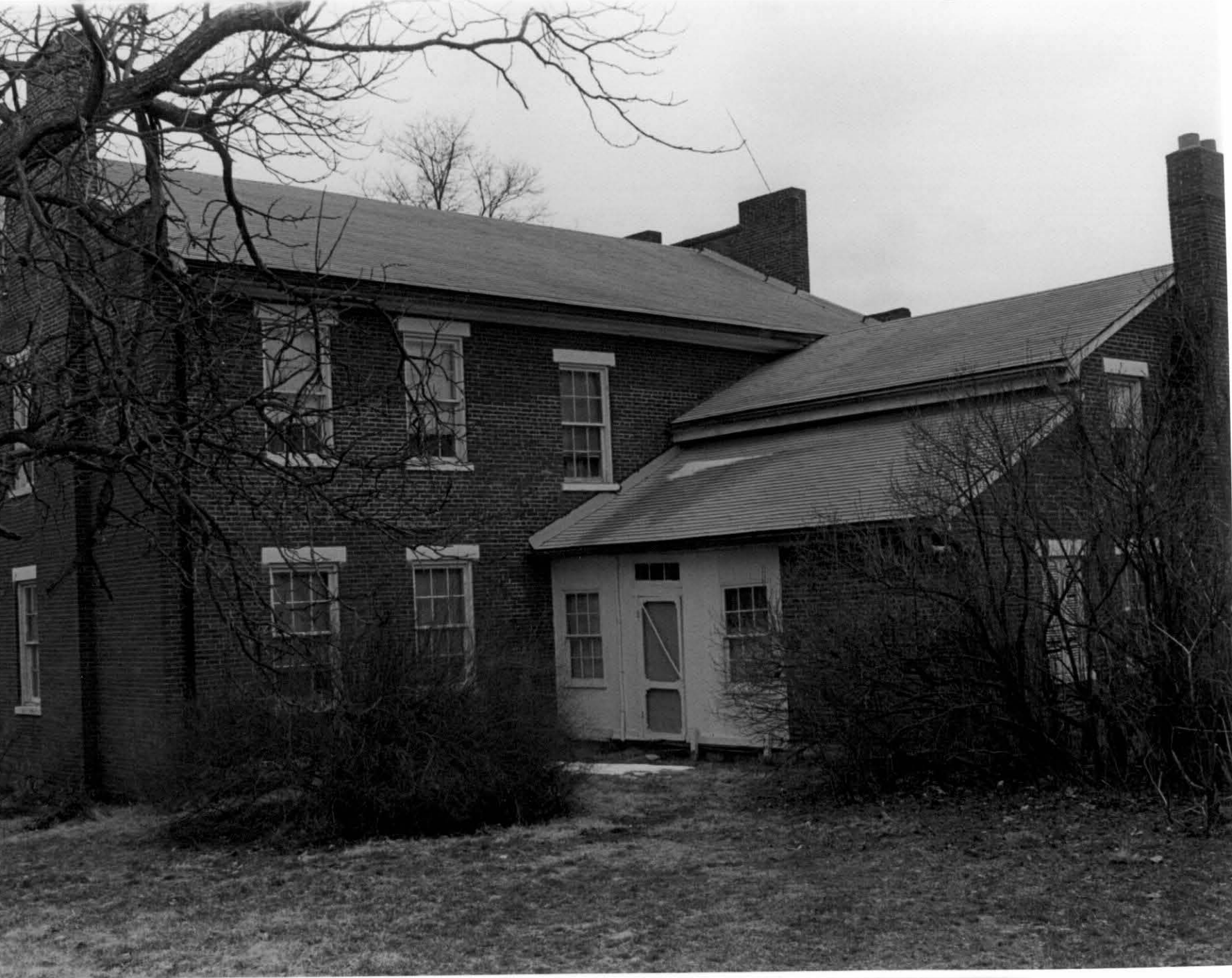
16. Jane Thompson ell, looking SE. Note porch plank wall, porch door transom, and shuttered cool room window. Compare with Ruggles ell, photo #6.
