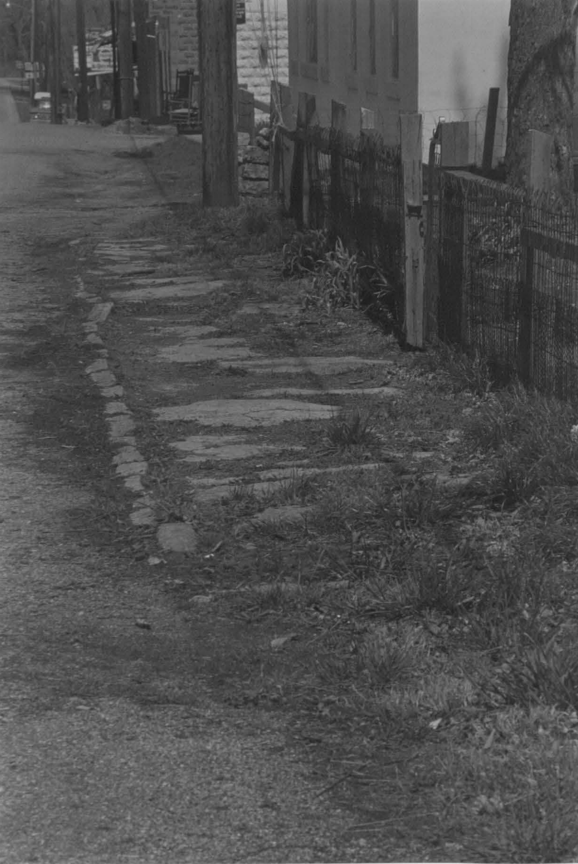
74. Flagstone walk and curb, Long-White house.
