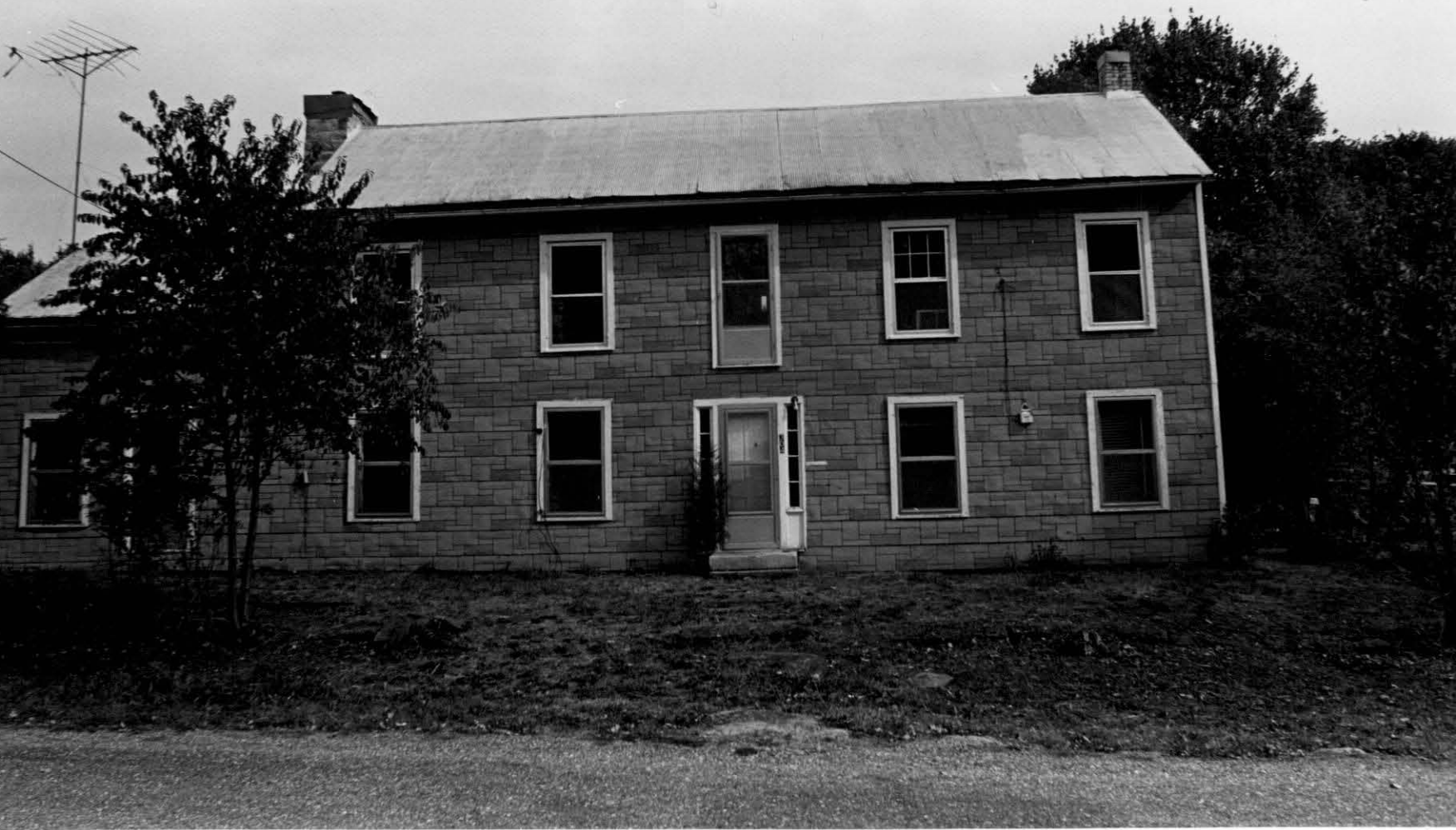
98. Craighead-Henry facade looking SE.
