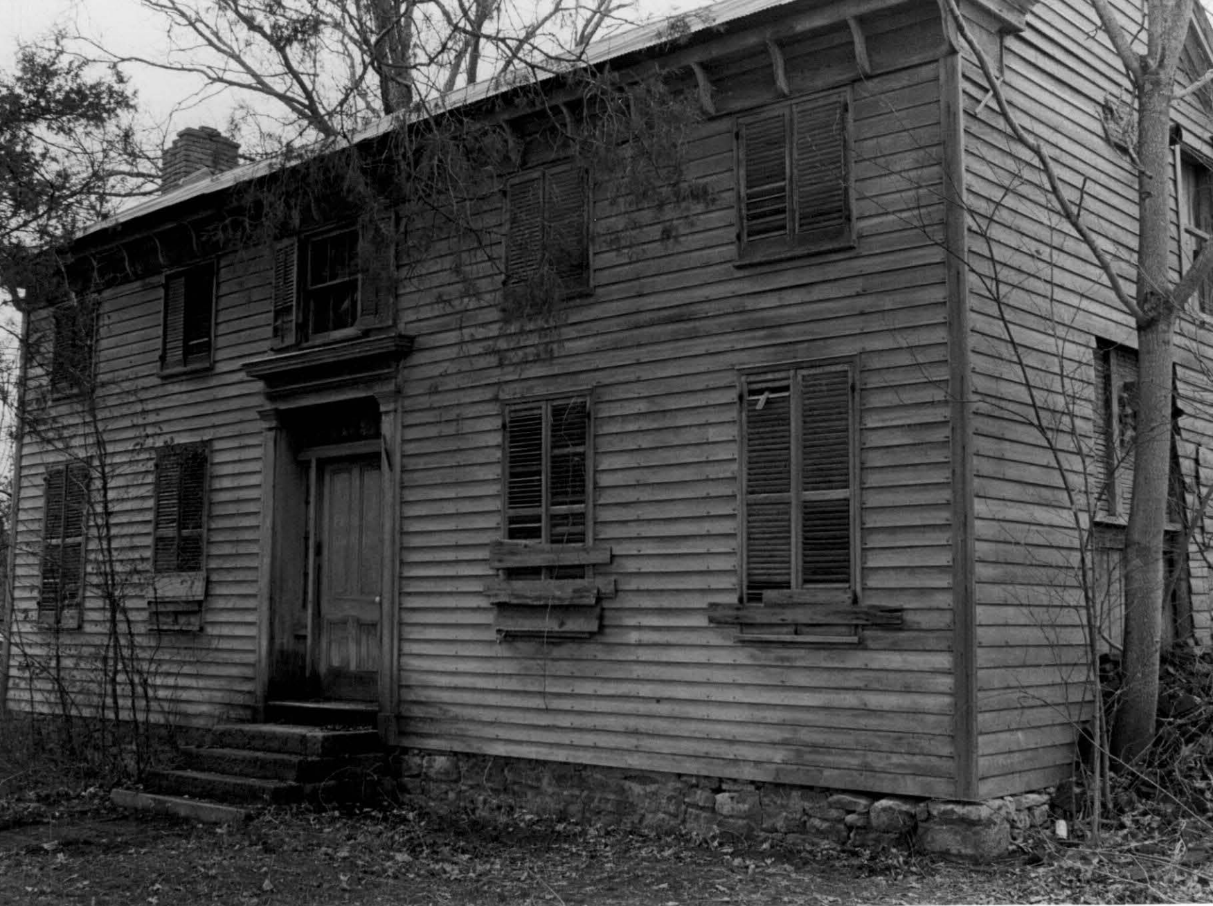
37. Ferson Carr house, #9, looking SW.
