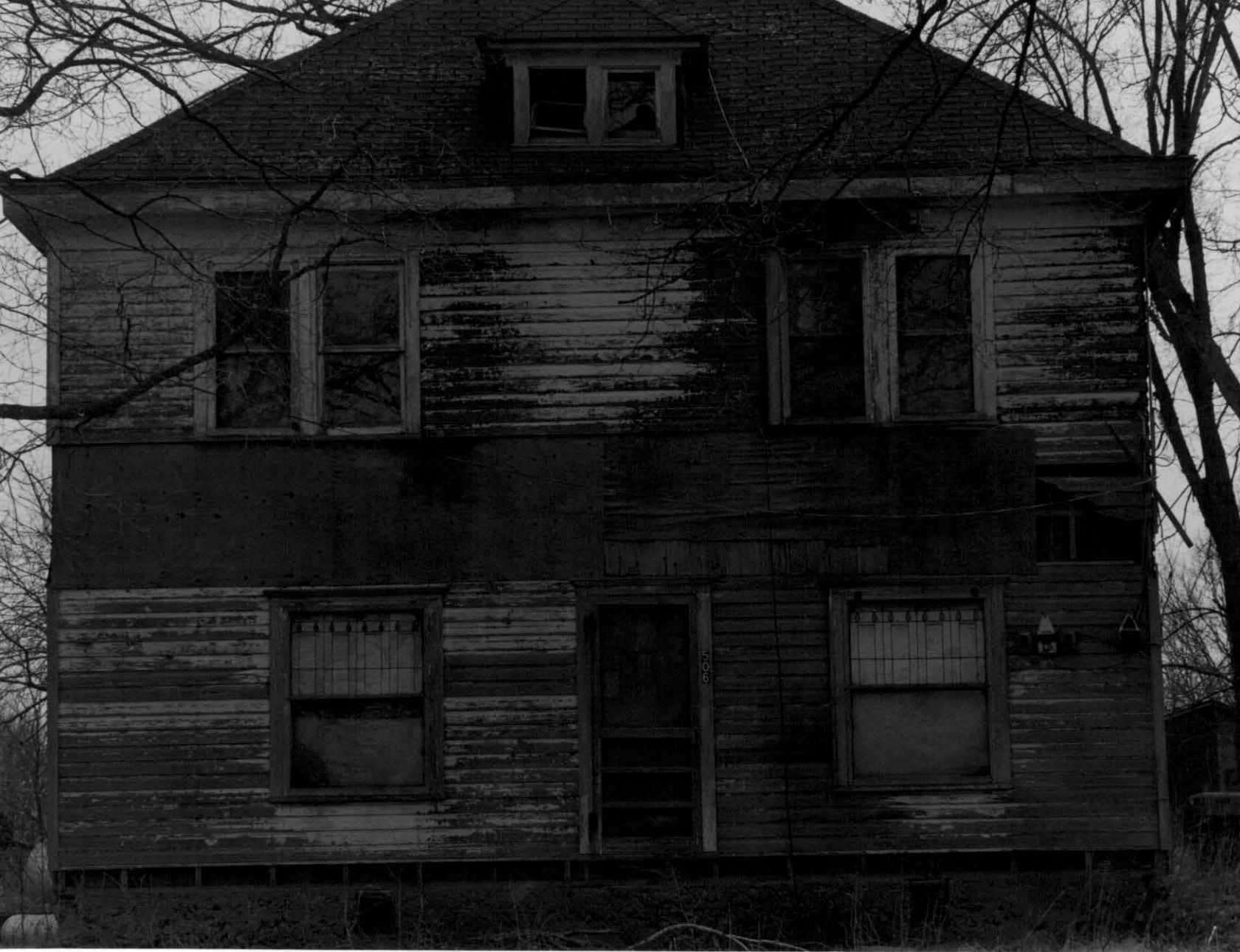
111. Tom Goodykoontz house, #31, facade view looking E.
