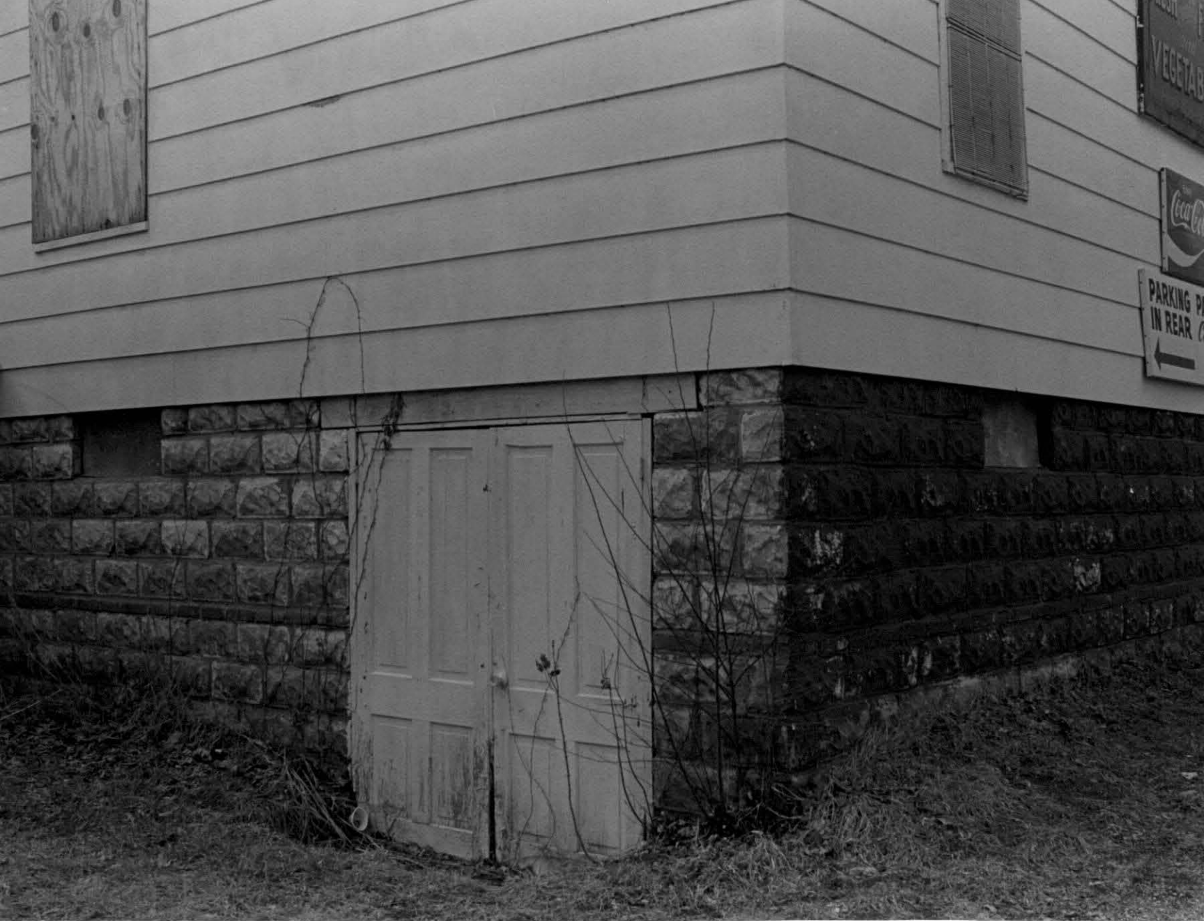
55. NE (rear) corner of Al and Dee's market, originally foundation of Caledonia Bank, built of the common concrete block with brick stringcourse.
