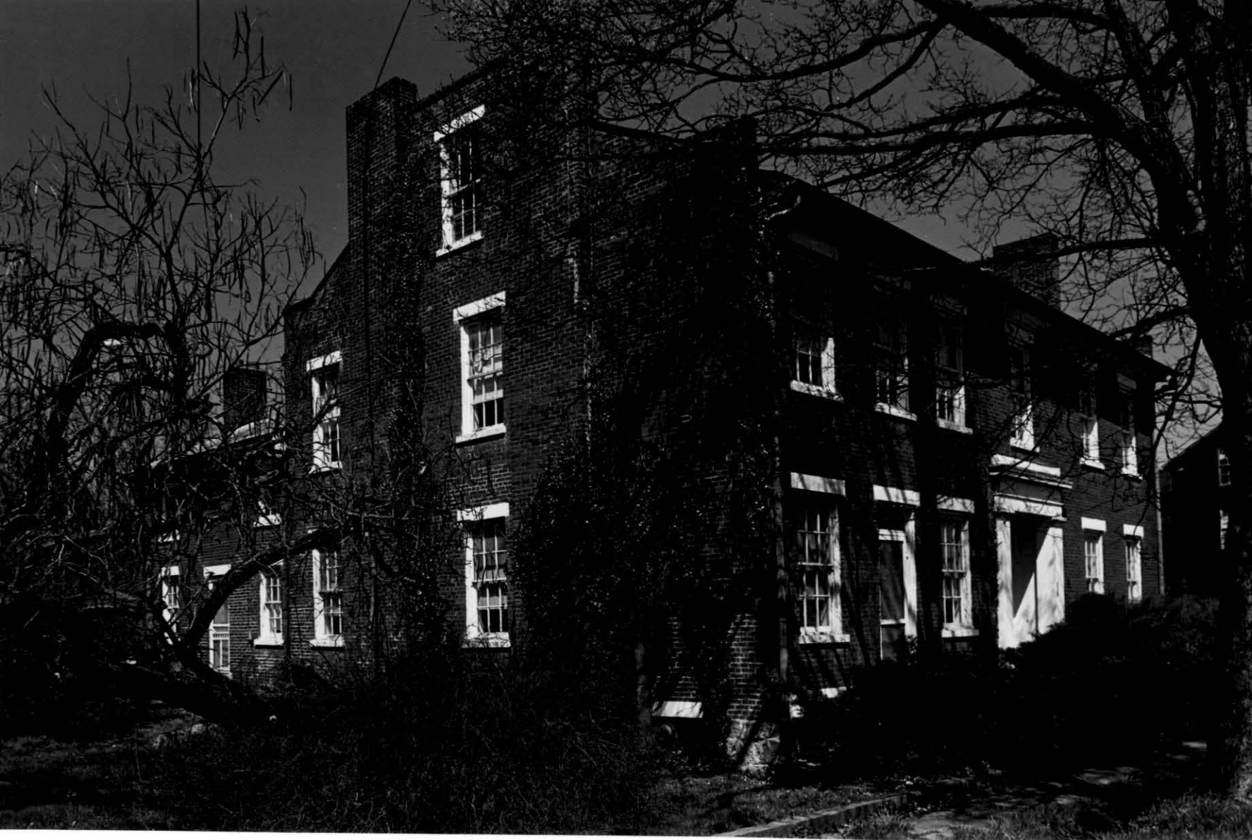
13. Jane Thompson house, looking NW. Note low retaining wall and minimal setback.
