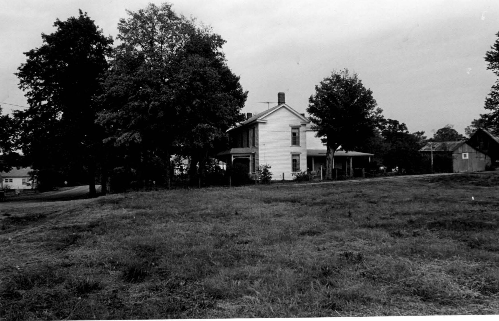
95. Bean house looking NNE across vacant lot 13.
