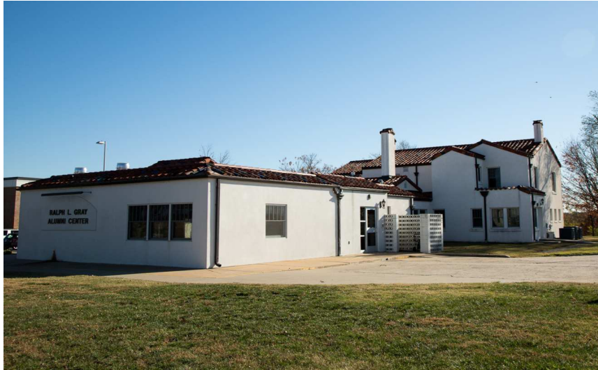
Figure 15: North and west elevations facing southeast.
