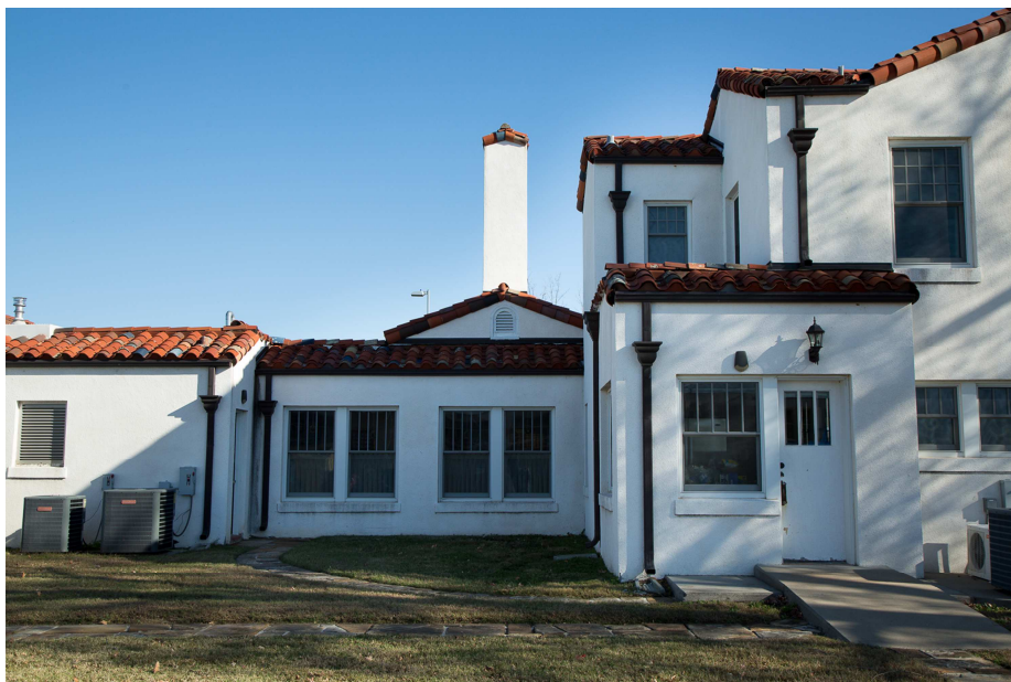
Figure 13: West elevation facing east.
