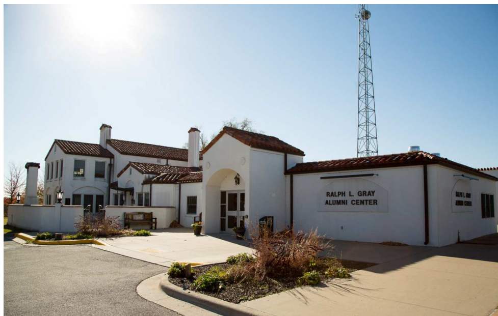
Figure 6: Northeast elevation facing southwest.
