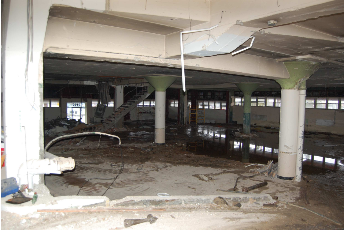
Figure 5. Concrete columns are intact throughout the building. First floor view is southeast.
