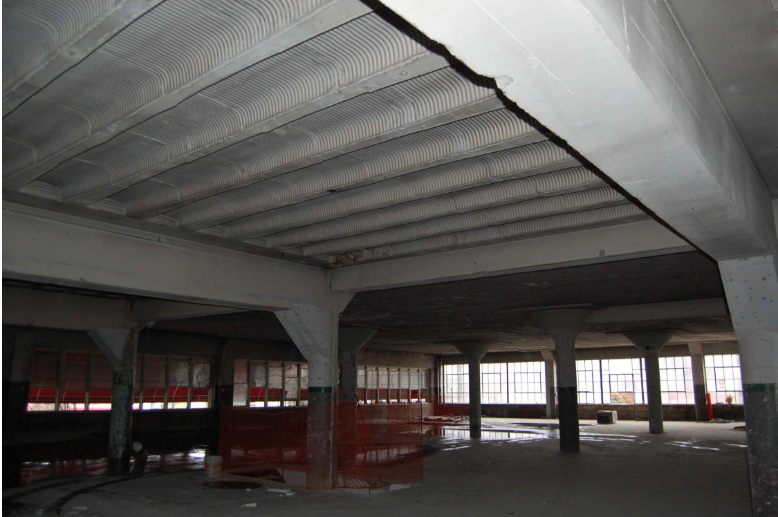
Figure 7. The building is primarily constructed of concrete, including the ceilings. View is second floor, southeast. Note the floor's ribbed concrete ceiling detail.
