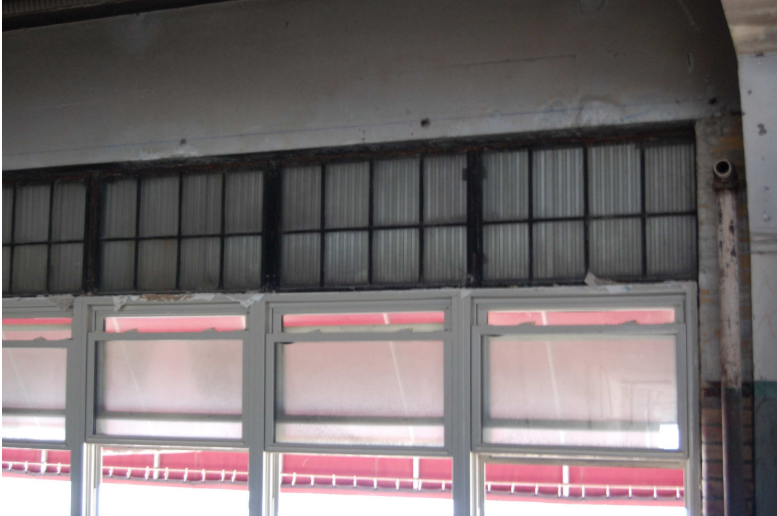
Figure 3. Original clerestory hopper windows, second floor, south wall.
