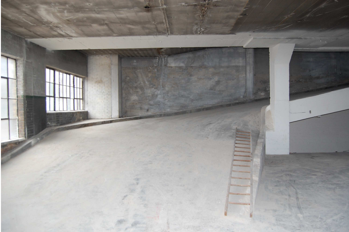
Figure 6. The building retains concrete ramps used to transport automobiles from the first floor to the roof. View is second floor, northwest corner.
