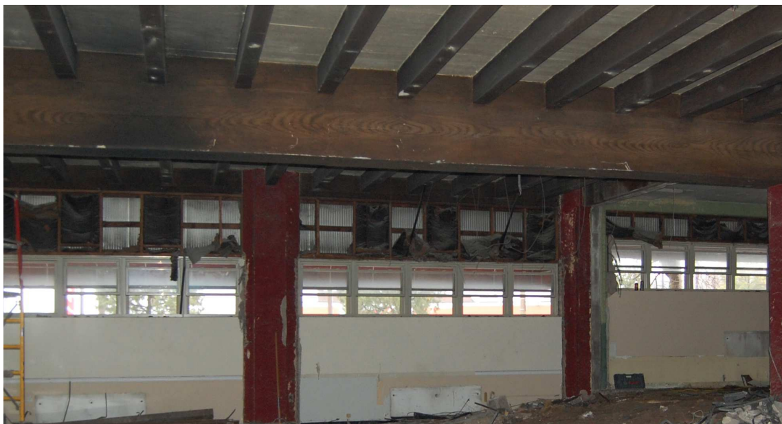
Figure 4. Original clerestory four-light windows above infilled display window bays, first floor, south wall.
