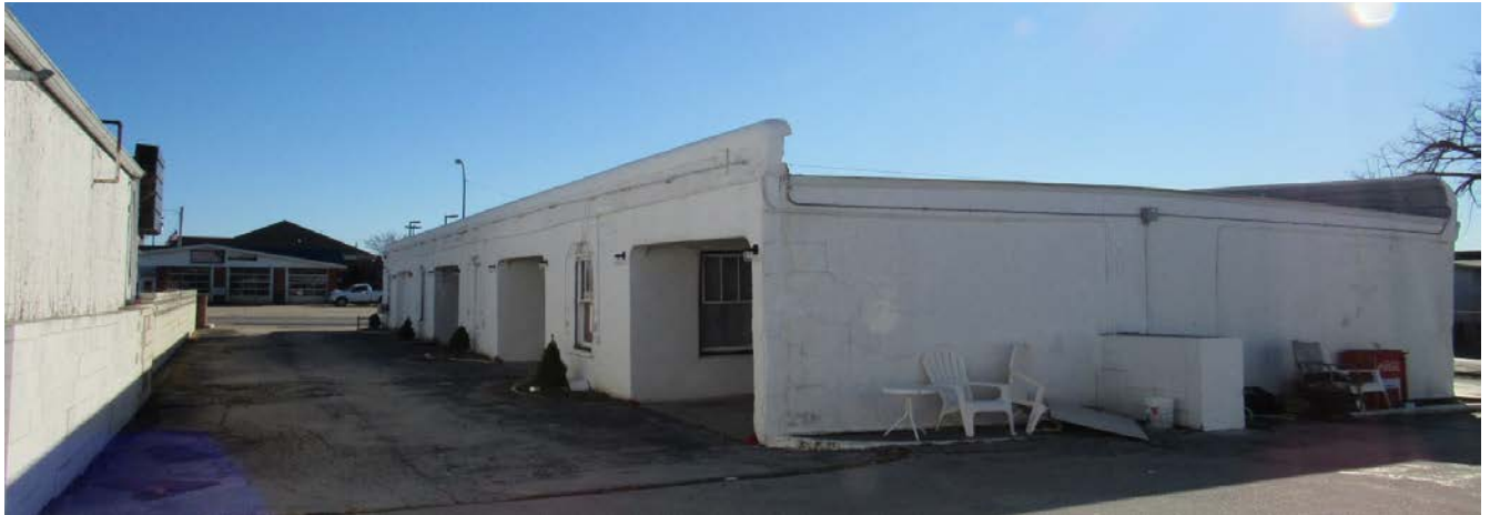
Figure 34. North and West elevations of 1939 building. Tunnel air access is located on the rectangular extension. (Emrie, 2022)
