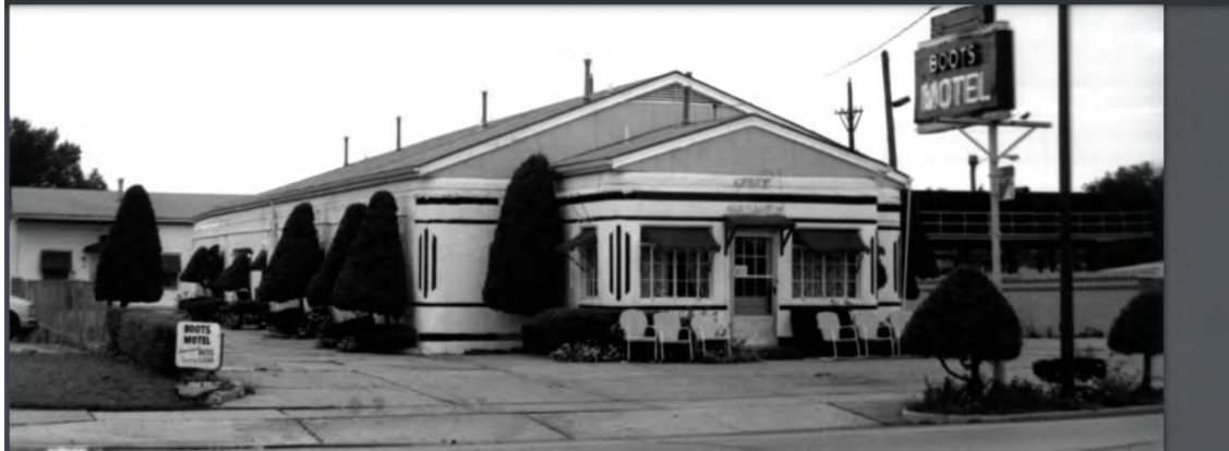
Figure 24. 1993 image of Boots Motel showing gable roofs installed in the 1970s. (Johnson)
