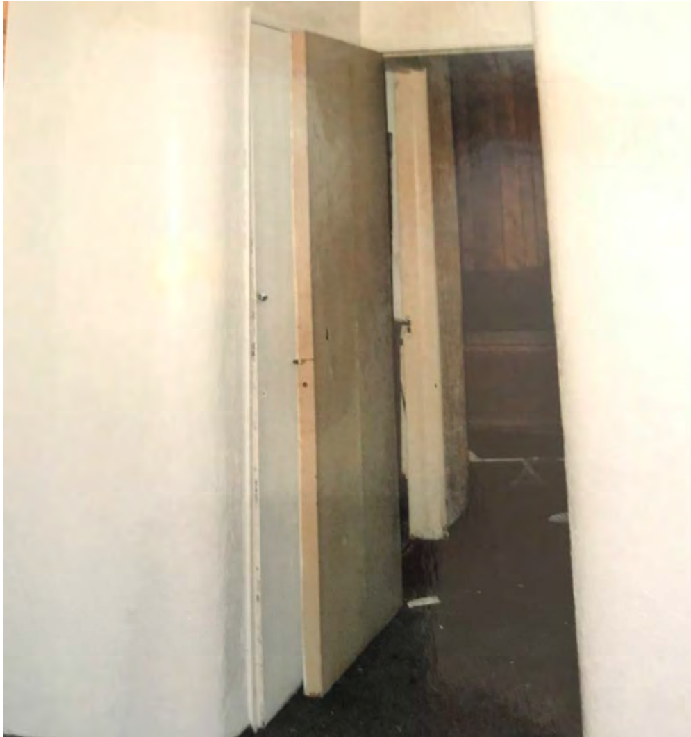
Figure 36. Connecting door between motel rooms 1 and 2 looking north. (Emrie)
