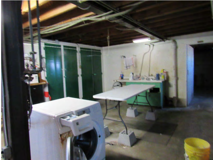
Figure 17. Tunnel from 1946 basement to 1939 Building. (Harvey)
