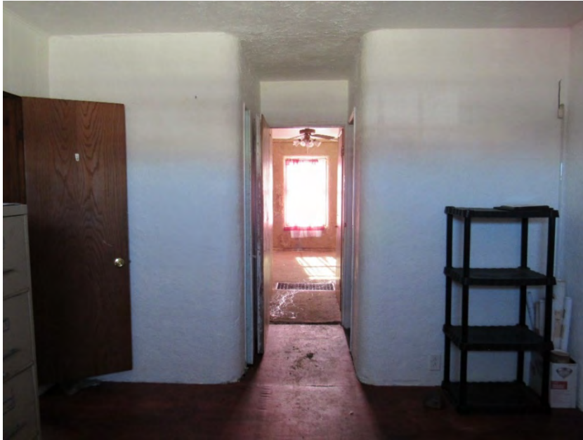
Figure 14. Interior of connecting units 1 and 2 in 1939 Building. Phase one of motel construction design. Note rounded corners on plaster walls, floor furnace in far room, plain wood door (probably homemade). (Emrie)
