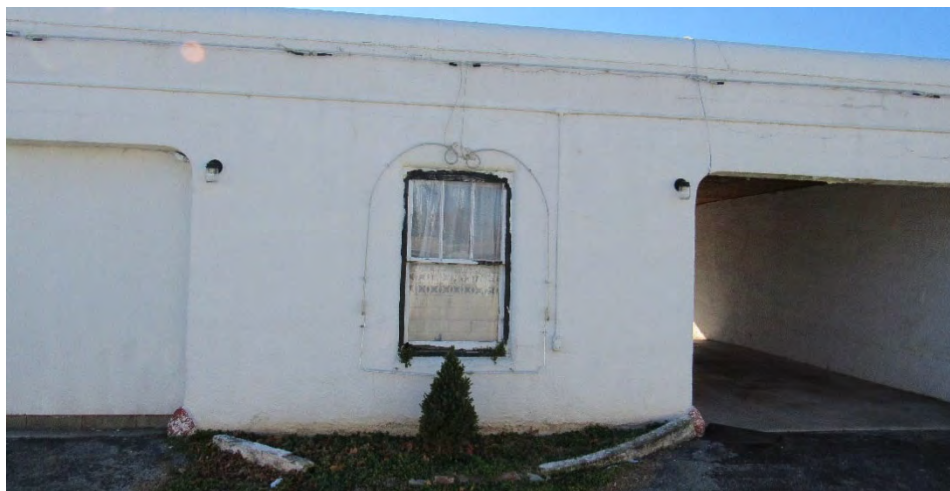
Figure 11. Detail north elevation of 1939 building showing closed in carport on left, Unit 3 window (3 Over 1), neon arch around window and open carport on right. (Emrie)
