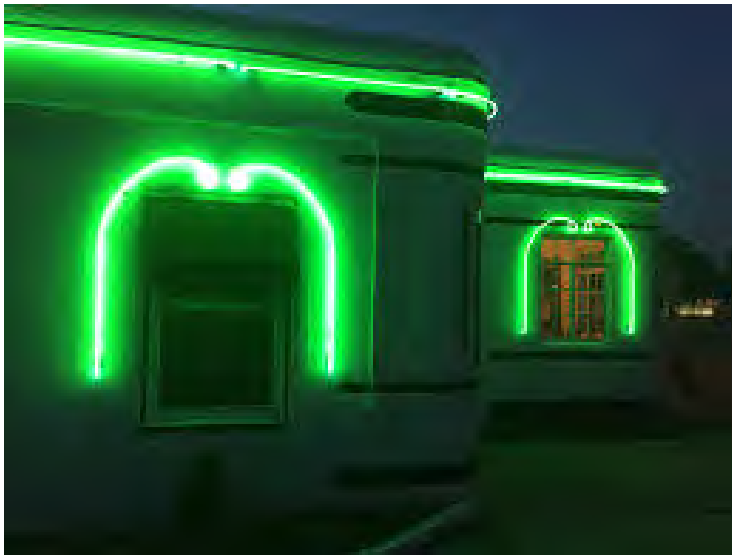
Figure 25. Detail of lighted neon around parapets and windows. SE corner of 1939 Bldg. (Halla)
