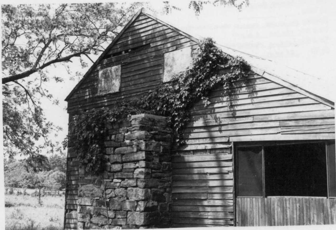
This building was built by the early settlers of the town of ... .. ... .. ... ..
