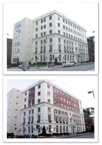
Top: Painted masonry building before paint removal. Kansas City, MO, 2004. Bottom: Masonry building after paint removal. Kansas City, MO 2006.
