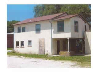
• Remove rear covered porch structure of Building B to restore integrity to original roofline. Replace with porch deck to match period with balustrade to match same on front of Building B.
