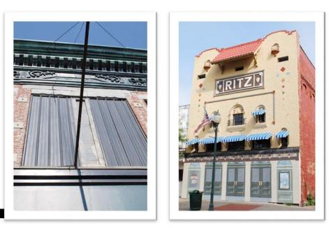
Left: Example of temporary mothball treatment . The metal coverings are neatly fit over the historic wood windows underneath providing protection from the elements until the building can be rehabilitated. Joplin, MO 2010. Right: View of painted plywood mothball treatment makes the temporary covering more aesthetically pleasing, Centerville, IA, 2009.
