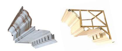
Left: Original deteriorated architectural cornice. Right: Replicated architectural cornice. New metal cornice has structural supports and is made of the same lead coated copper as the original, Rockport, Missouri, 2009.
