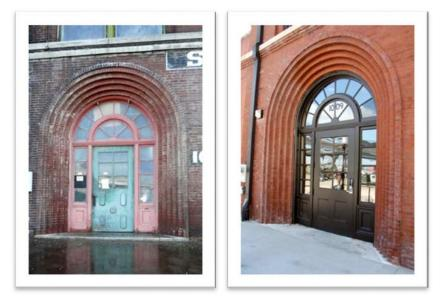
Left: Image of a deteriorated historic wood door with transom and sidelites. Right: Image of new replica aluminum door with transom and sitelites. The new door accurately recreates the look and feel of the original in a new material. Kansas City, MO 2009.
