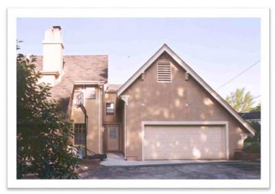
Example of traditional stucco installed on a new garage addition. Kansas City, MO, 2005.
