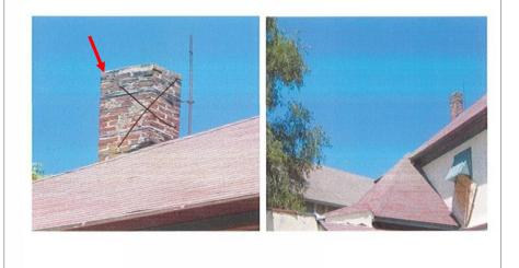
Remove existing shingles, repair decking as needed and re-roof with architectural 40 yr. shingles. (color sample to be provided)
