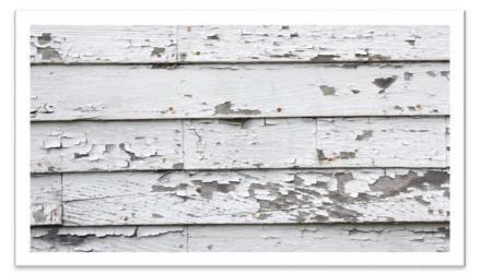
Example of cracked and peeling paint in need of repair. Loose paint should be carefully removed prior to priming and painting, Harrisburg, Missouri, 2008.
