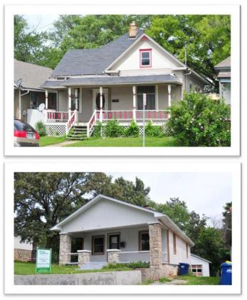
Top: Example of a wood railing in good condition, 512 Isley Boulevard, 2014. Bottom: Example of a house with its historic railing removed and an incomplete railing installed, 103 North Francis, 2014.
