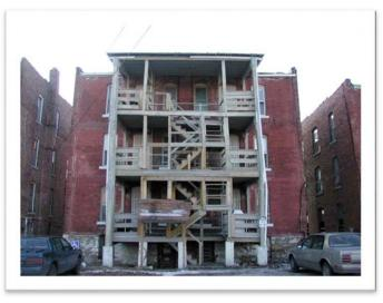
View of a rear stair enclosure in need of repair. The majority of the deterioration to the porch is from weather and water. Kansas City, MO, 2000.
