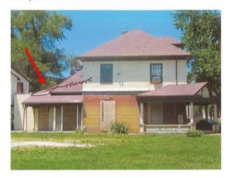
• Remove roofing addition at rear of Building A to restore original roofline on add-on. (This add-on is believed to be the jail structure added by Bill Payne after original construction of home. The roofline has been compromised by adding multiple pitches in an attempt to shed water.) Make repairs to framing of roof as needed and re-roof. \*refer to pictures #4 & 5
