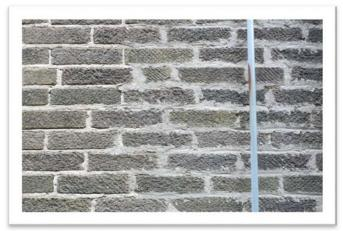
Incompatible Mortar Joints. New mortar installation (right side of the picture) does not match the original (left). Repointing has left mortar on the face of the brick.
