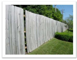
Example of fencing in need of repair. Missing or broken fencing should be replaced to match the existing fence in-kind. All fencing should be painted or stained with a solid stain.
