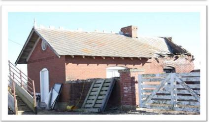
Top: View of mothballed house, ready for rehabilitation. Lawrence, KS, 2009. Below: View of structurally unsound roof structure on a historic outbuilding. The rest of the structure is in good condition, therefore only select demolition of the deteriorated roof structure is needed and can be repaired and saved. Boonville, MO 2009.
