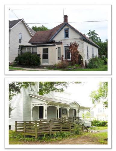
Top: Example of an inappropriate infill of a front porch. Bottom: Example of an inappropriate exterior ramp installation on the front of a historic house. The ramp design dominates the first impression of the house and does not resemble the house's style, nor is it painted to match.
