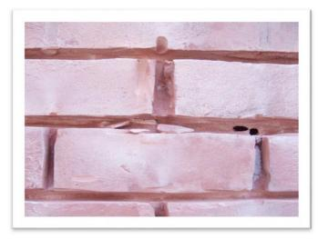
Incorrect mortar removal has caused permanent and irreparable damage to the historic brick, Kansas City, Missouri, 2009.
