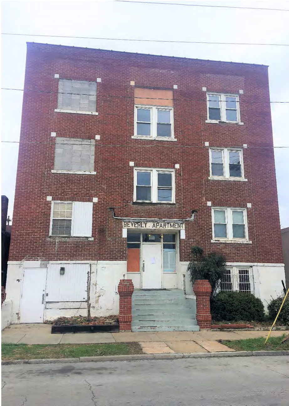
Photo 3 of 18: Façade (South wall), looking north.
