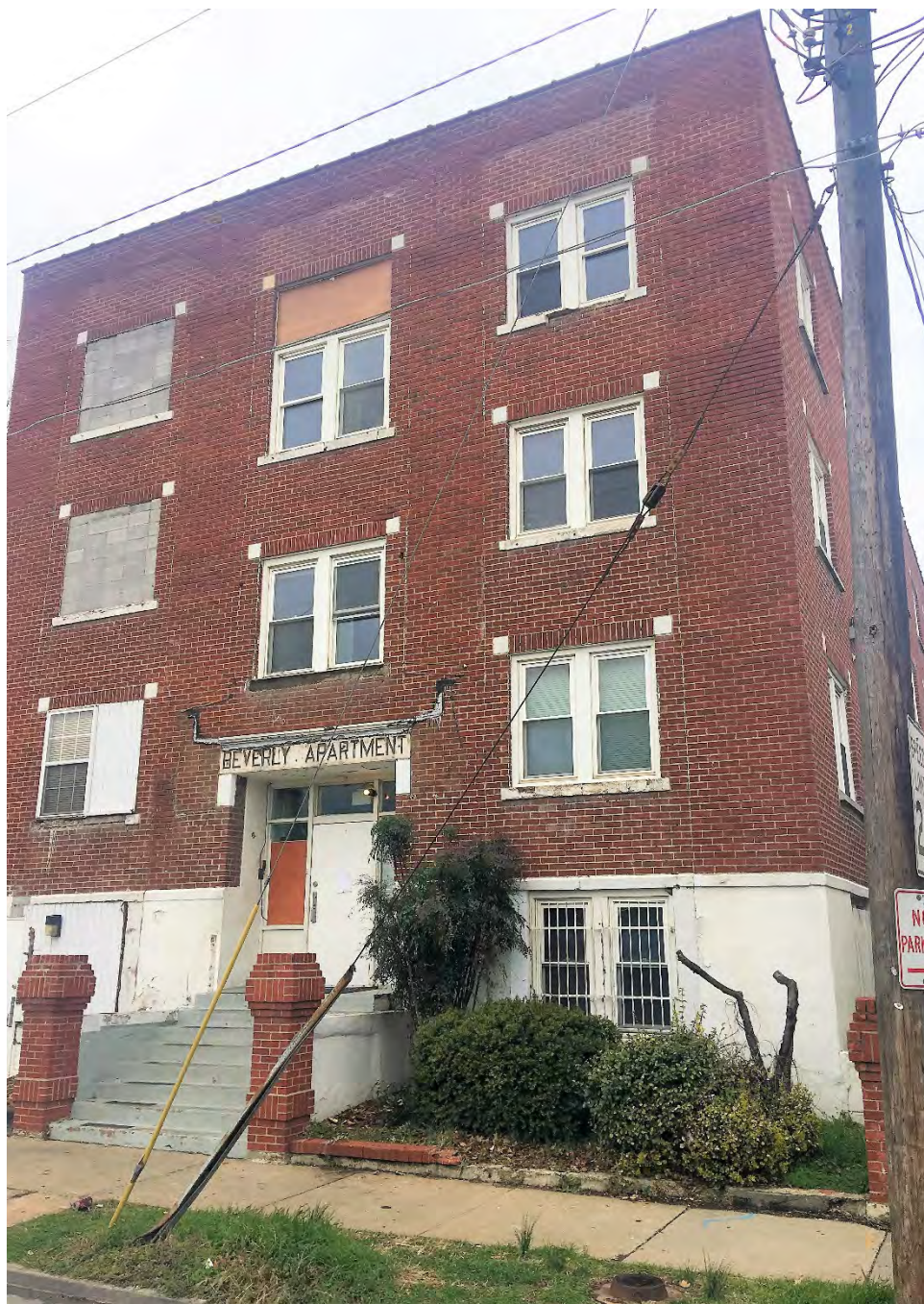
Photo 5 of 18: Southeast corner, looking northwest.
