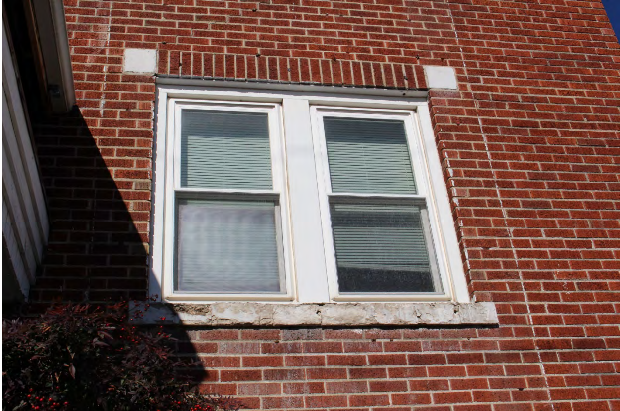
Photo 4 of 18: Window detail: façade, looking north.
