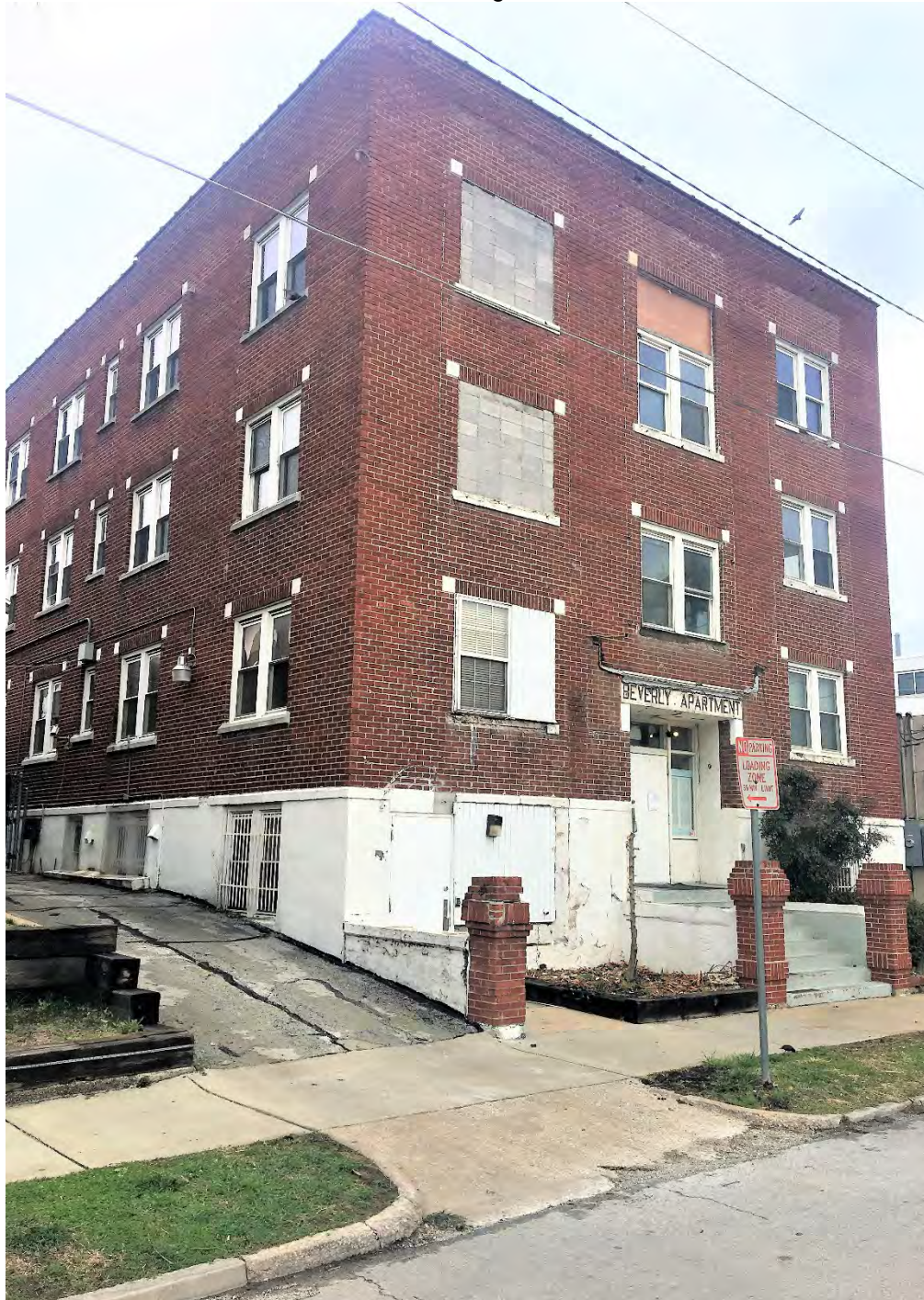
Photo 2 of 18: Southwest corner, looking northeast.
