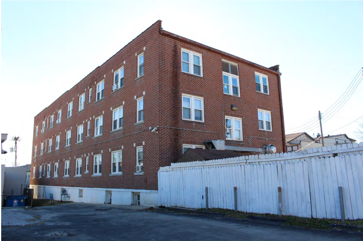
Photo 6 of 18: Northeast corner, looking southwest.
