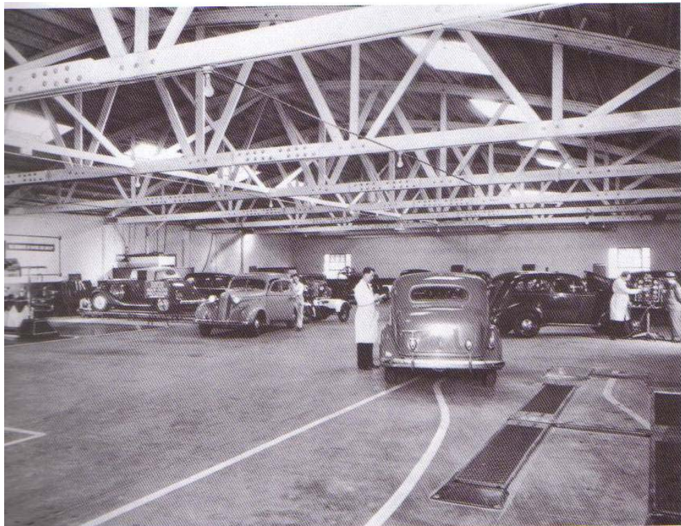
Figure 7. Interior view of a service facility (site unknown) similar to the Berry Motor Car Service Building. Note windows, open plan, concrete floor, and overhead lighting/trusses. Photo from GM Media Archives – Source: Robert Genat, The American Car Dealership (St. Paul, MN: Motorbooks International, 2004), p. 149.
