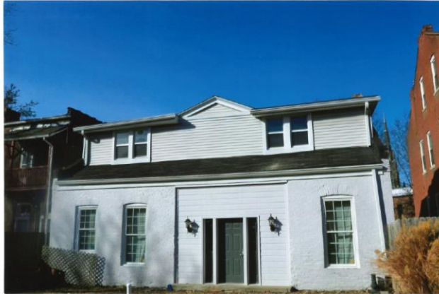
Back of 2724 S. Jefferson. Addition of large dormer and loss of back porch.
