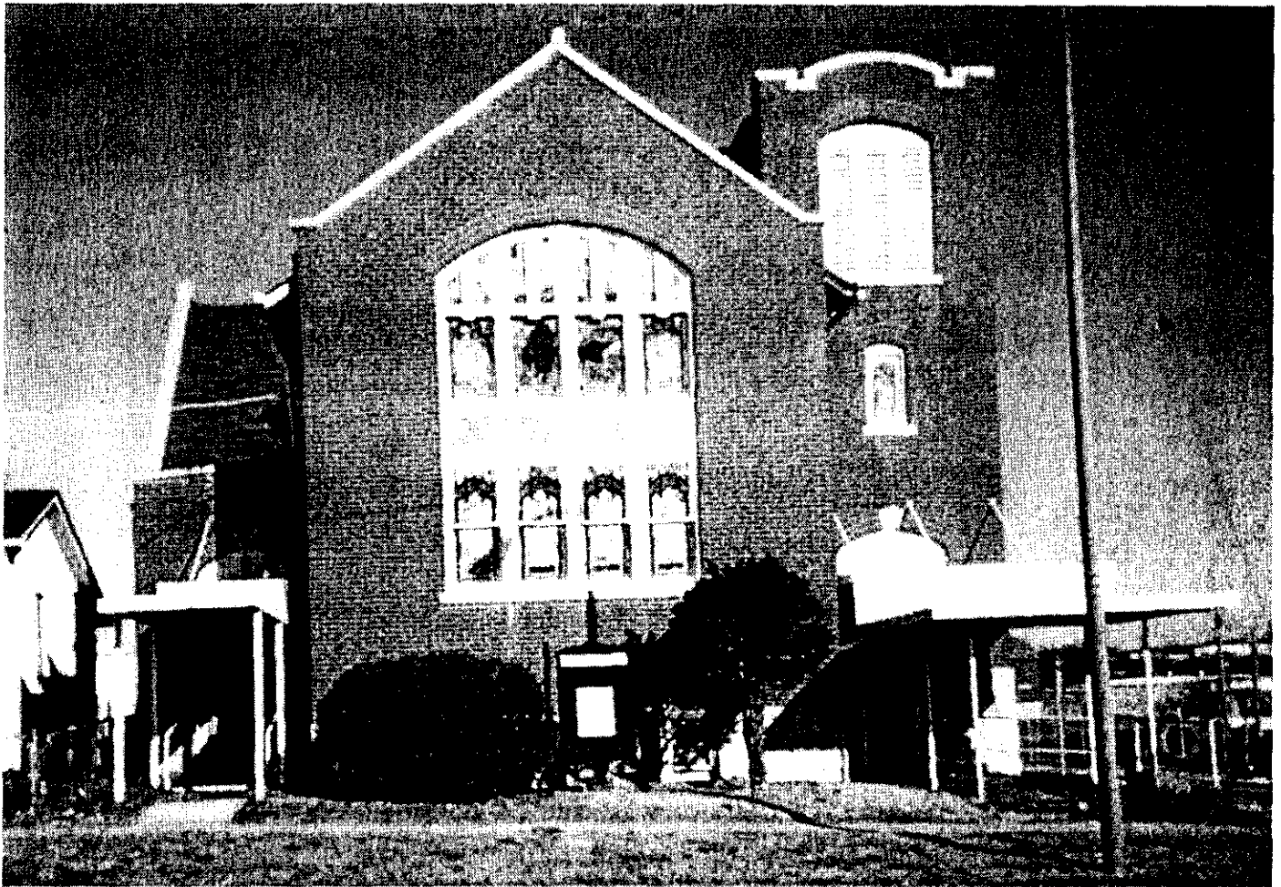
Figure 17: Historic Photograph Pitts Chapel (c. 1912) at 706 North Benton Avenue in Springfield, Greene County, Missouri. (Photo: 2000. Historic Springfield, Inc. Used with permission.)
