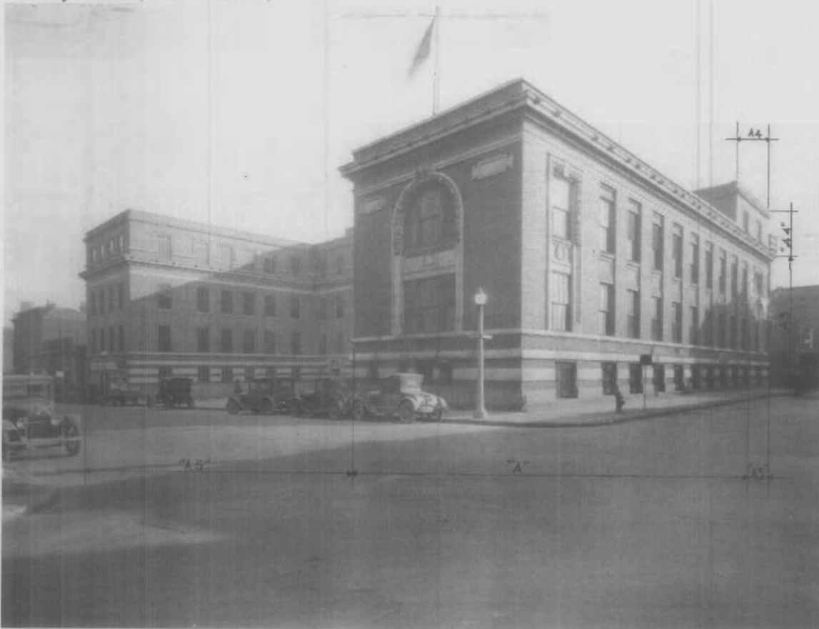
Figure 3: Beaumont Telephone Exchange. Circa 1927. Courtesy of SBC Archives and History Center, San Antonio, Texas.
