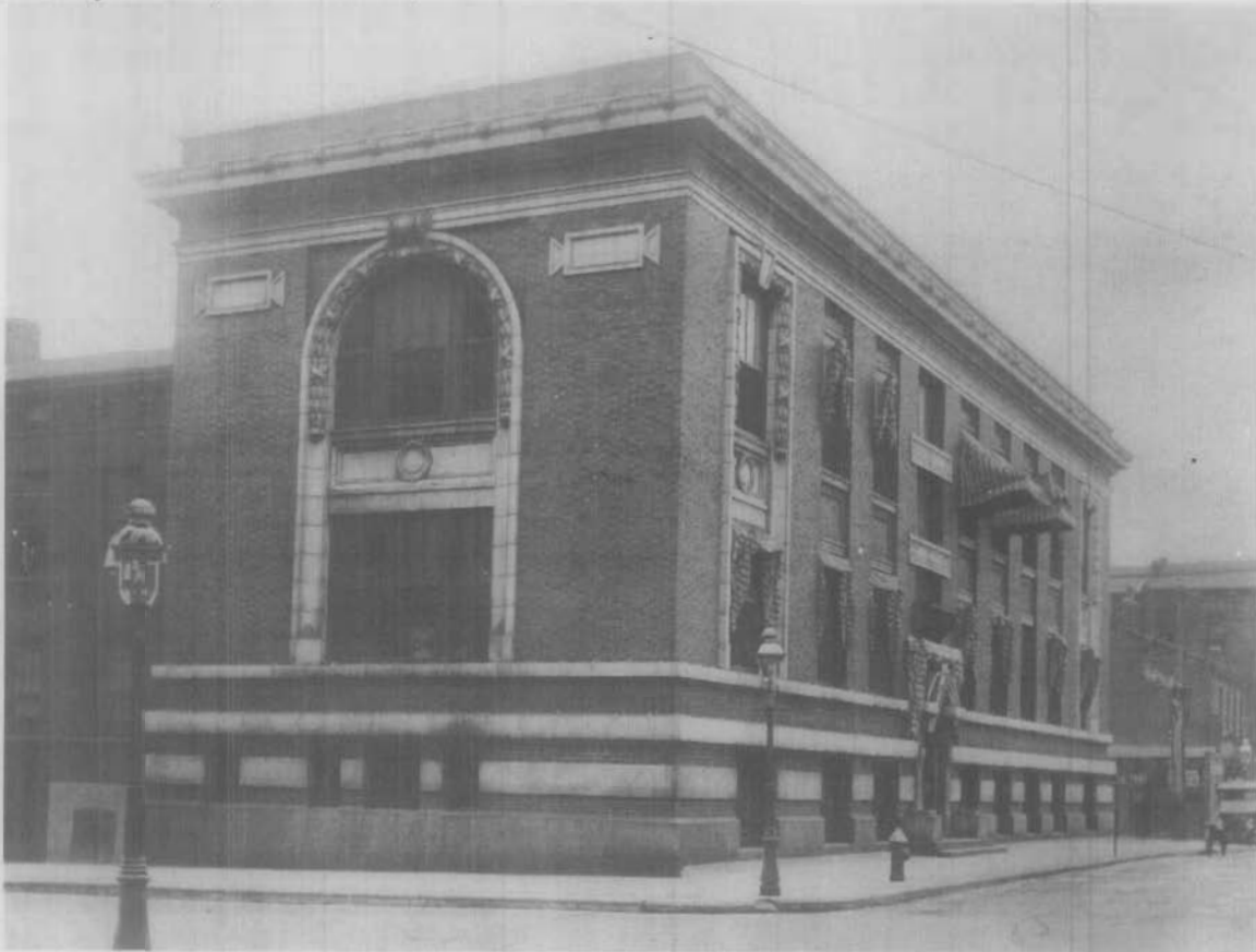
Figure 2: Beaumont Telephone Exchange. Circa 1903. Courtesy of SBC Archives and History Center, San Antonio, Texas.
