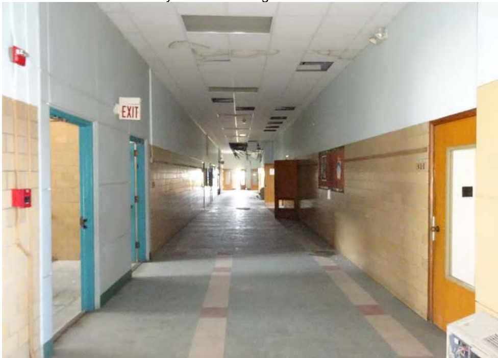
26 of 29 Third floor hallway. Camera facing west.
