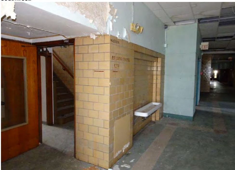
18 of 29 First floor hallway with "Reading Center" sign and east mezzanine stairs. Camera facing southwest.
