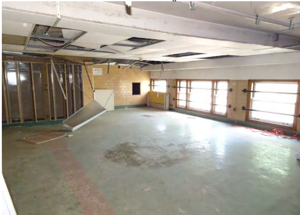
19 of 29 North mezzanine. Camera facing northwest.
