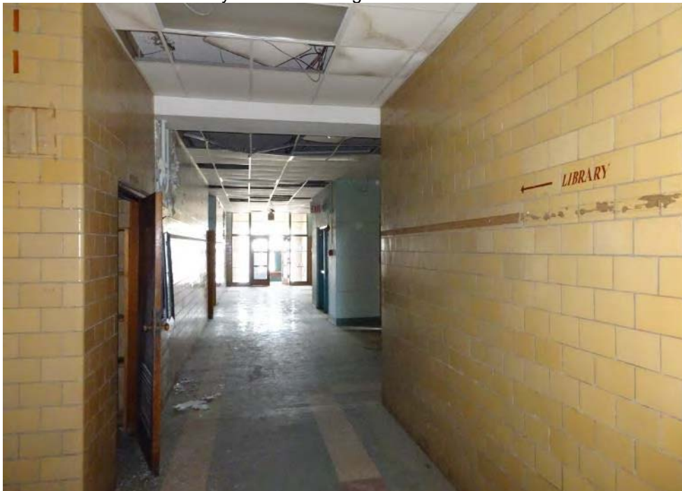
17 of 29 First floor hallway. Camera facing east.
