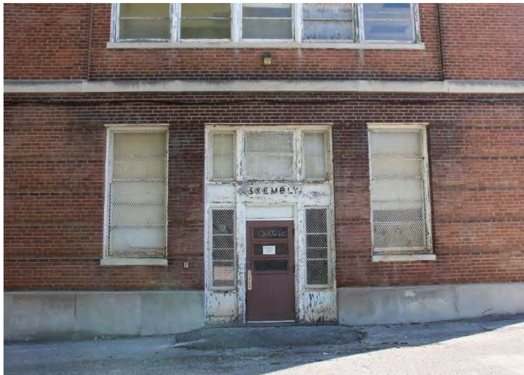
12 of 29. Assembly room entrance. Camera facing south.
