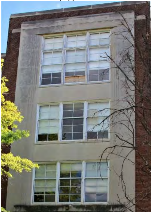
13 of 29. Detail, upper center facade. Camera facing south.
