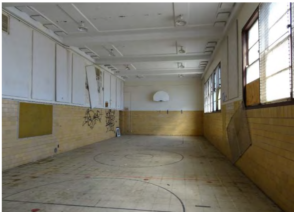
20 of 29 Gymnasium. Camera facing east.
