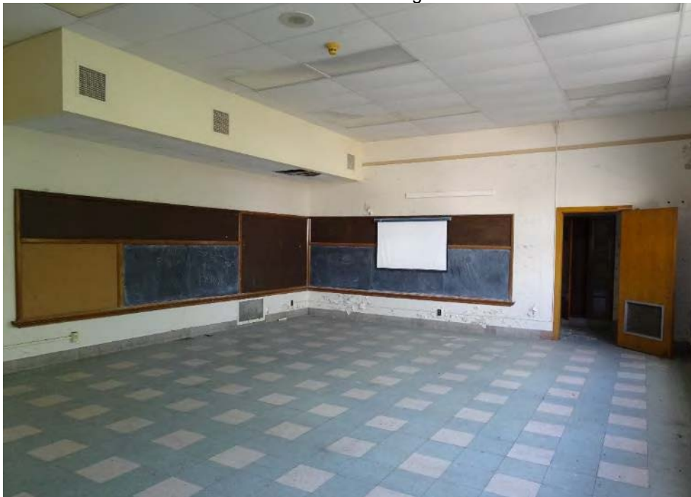
25 of 29 Second floor classroom. Camera facing southwest.
